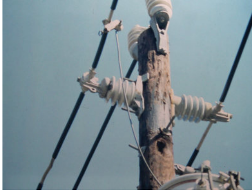
Figure 3.13 Example of a compact armless design using covered conductors. (Courtesy of Duke Energy.)
