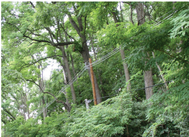
Figure 3.14 Spacer cable. (Courtesy of Hendrix Wire and Cable Inc.)
