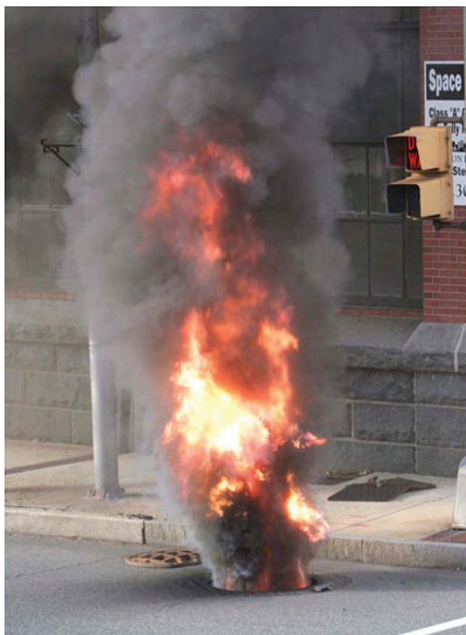
Figure 14.33 Example manhole event. (From EPRI 1015889, Manhole Event Risk Management Strategies: High-Level Overview , Electric Power Research Institute, Palo Alto, CA, 2008. Copyright 2008. Reprinted with permission.)
