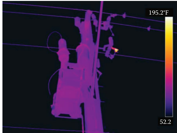
Figure 7.24 Hot capacitor cutout. Note the blown fuse on another phase. (Courtesy of Osmose Utilities Services, Inc.)
