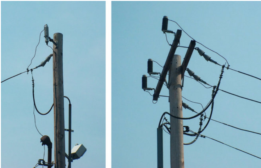
Figure 13.21 Arrester applications with long lead lengths.
