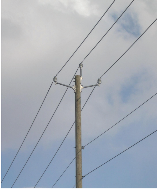
Figure 2.1 Three-phase 34.5-kV armless construction with covered wire.
