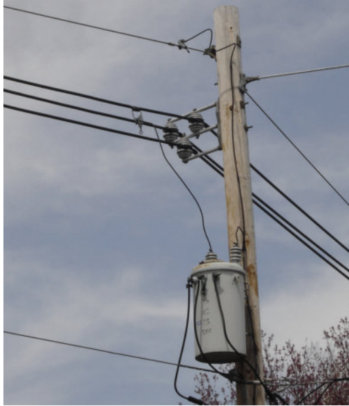
Figure 9.15 Unfused CSP on a mainline.
