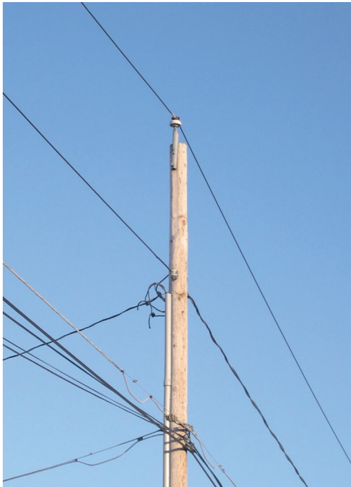
Figure 2.2 Single-phase circuit, 7.2 kV line-to-ground.
