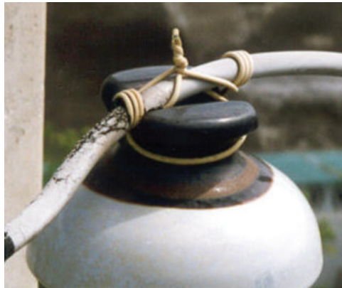
Figure 3.15 Example of a covered wire tie on a covered conductor. (From Vincent, W. R. et al., The Mitigation of Radio Noise and Interference from External Sources , 6th ed, United States Navy Naval Postgraduate School, 2007.)
