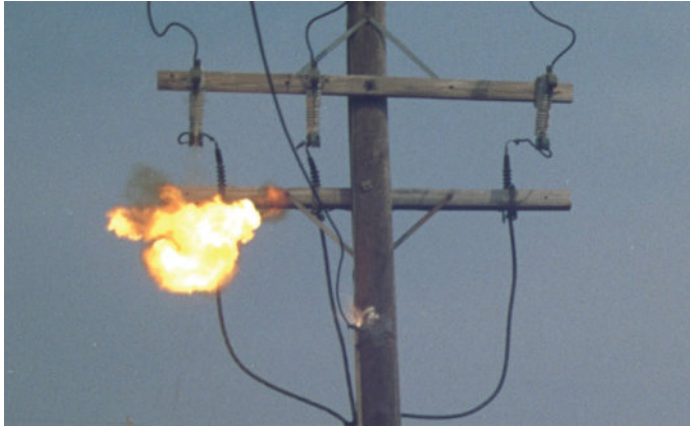
Figure 9.3 Example operation of an expulsion fuse during a fault. (Courtesy of the Long Island Power Authority.)
