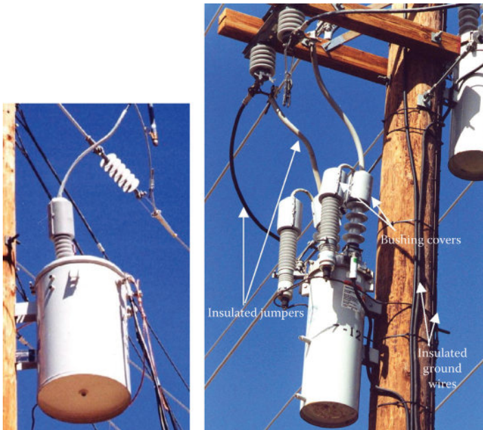
Figure 3.18 Examples of wildlife protection with animal guards and covered jumpers. (From EPRI 1001883, Distribution Wildlife and Pest Control , Electric Power Research Institute, Palo Alto, CA, 2001. Copyright 2001. Reprinted with permission.)
