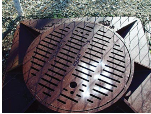
Figure 14.34 Vented manhole cover. (From EPRI 1015889, Manhole Event Risk Management Strategies: High-Level Overview , Electric Power Research Institute, Palo Alto, CA, 2008. Copyright 2008. Reprinted with permission.)
