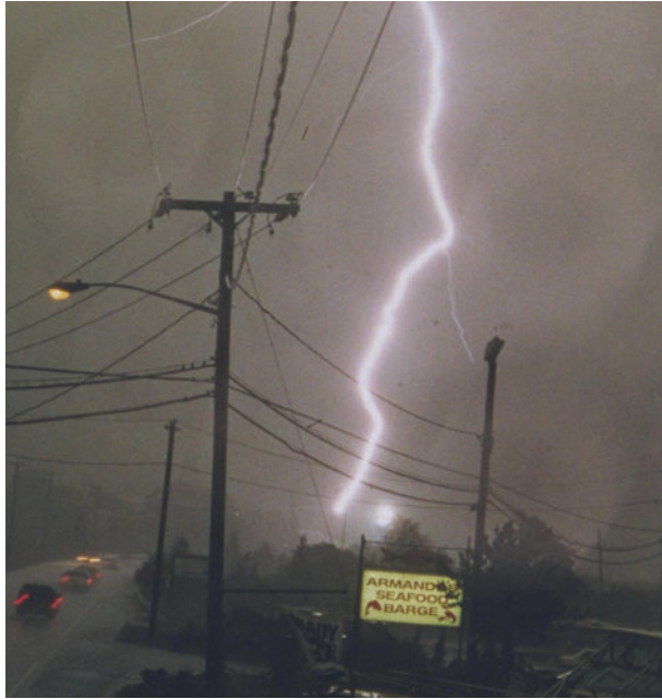
Figure 13.31 Lightning-caused fault on a Long Island Lighting Company 13-kV circuit. (Short, T. A. and Ammon, R. H., Monitoring results of the effectiveness of surge arrester spacings on distribution line protection, IEEE Transactions on Power Delivery , vol. 14, no. 3, pp. 1142–50, July 1999. © 1999 IEEE.)
