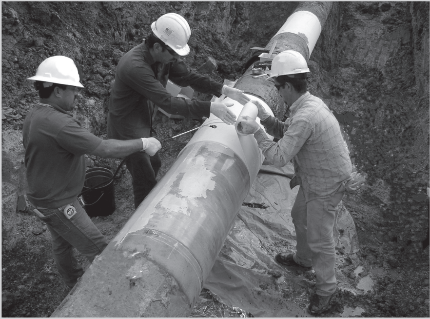
Fig. 9–27. Composite wrap reinforcing the pipe (Courtesy CorroDefense, LLC)
