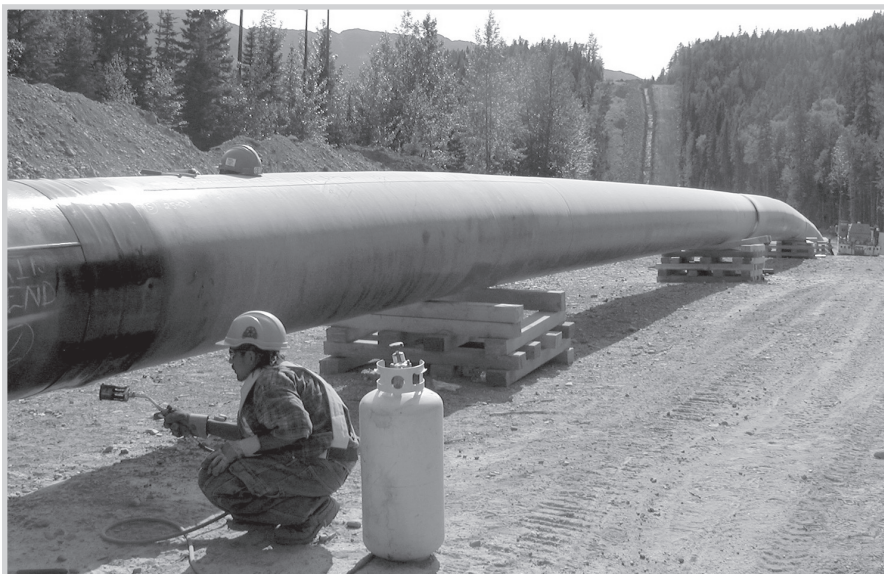
Fig. 11–4. Shrink sleeve being installed on a girth weld (Courtesy Canusa–CPS)
