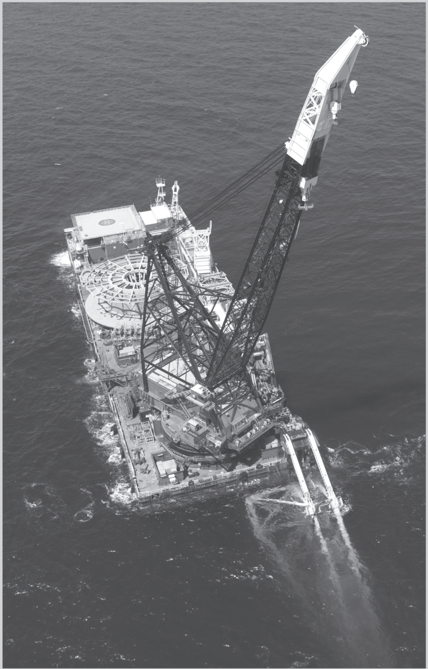
Fig. 7-8. Reel barge laying pipe (Courtesy Global Contractors)
