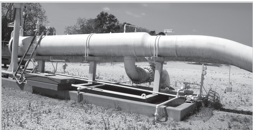
Fig. 9–31. Pig receiver. Note the “barrel” of the receiver has a larger diameter than the pipeline. Flow pushes the pig past the outlet on the bottom of the barrel, and it coasts to a stop. A valve (not shown) is closed to stop flow through the receiver, and the pig is removed by opening the closure on the end (left). (Courtesy Miesner, LLC)
