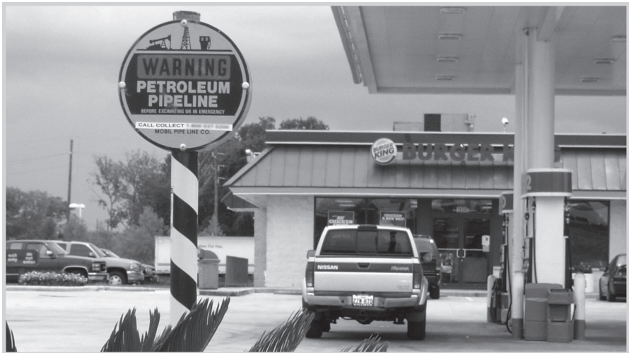
Fig. 9–11. Typical ROW marker (Courtesy Miesner, LLC)
