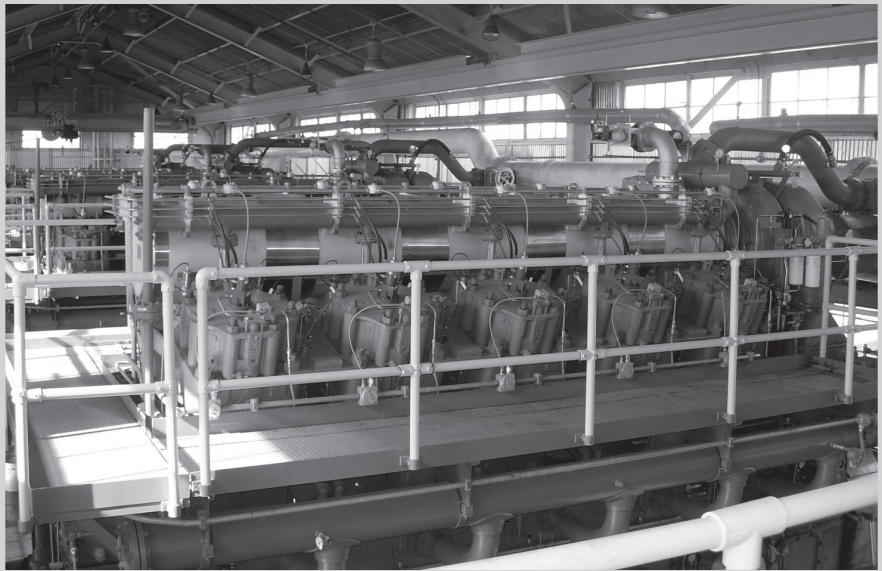
Fig. 5–9. Inside of a origination station with reciprocating compressors. From a catwalk about 10 ft from the floor in the compressor station (shown in fig. 5–10), five cylinders of the V-10 engine are visible. (Courtesy Williams Gas Pipeline; photo by Tom Miesner)
