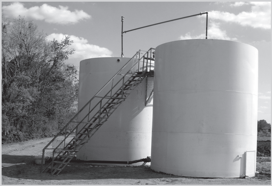
Fig. 1–2. Crude oil tank battery at a well site (Courtesy Miesner, LLC)
