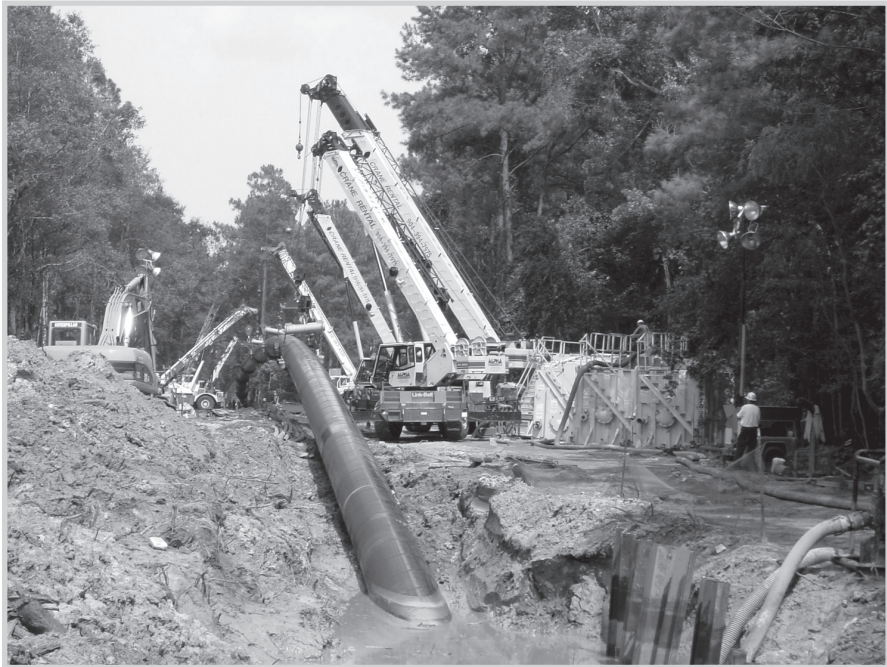
Fig. 13–15. Pulling the pipe through a directional drill (Courtesy Mears Group, Inc.)
