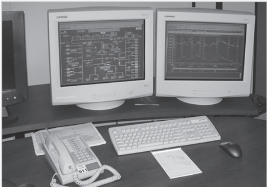
Fig. 8-4. Human-machine interface. This picture only shows two displays, but the controller consoles typically have four to six. (Photo by Tom Miesner)
