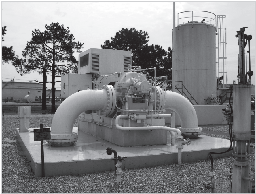
Fig. 11–23. Electric motor driving a centrifugal pump (Courtesy Miesner, LLC)
