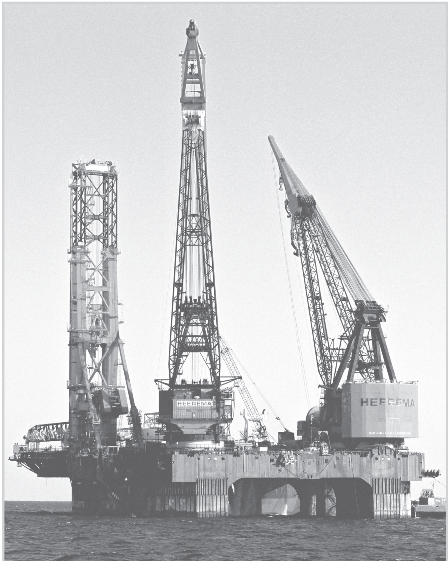
Fig. 2–9. Pipe-laying vessel. Vessels like this one can lay pipe in water depths as great as 10,000 ft. (Courtesy Heerema Marine Contractors)
