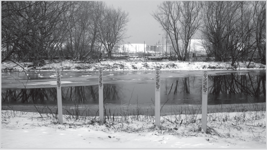
Fig. 9–10. Cleared and marked ROW (Courtesy Miesner, LLC)
