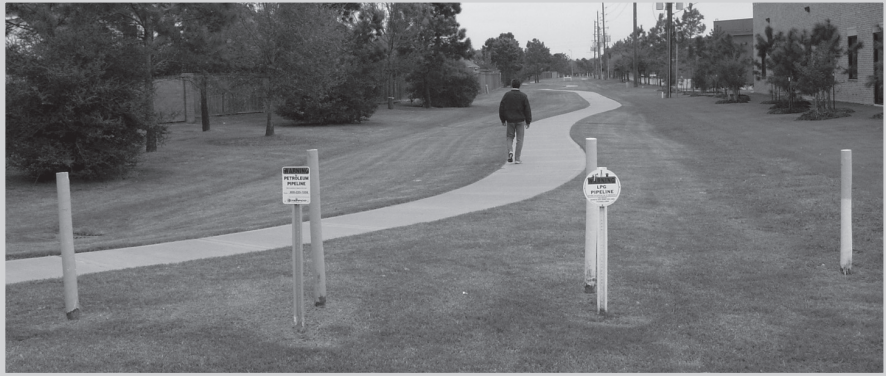
Fig. 14–3. Suburban ROW. Two pipelines snake between a shopping center and a housing development. In this case, the subdivision and pipeline companies cooperated to build a green belt with a walking path. (Courtesy Miesner, LLC)
