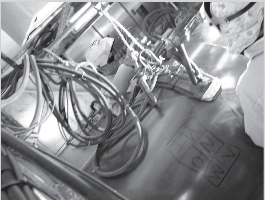
Fig. 13-6. Automatic welding (Courtesy U.S. Pipeline, Inc.; photo by Adam Aronson)
