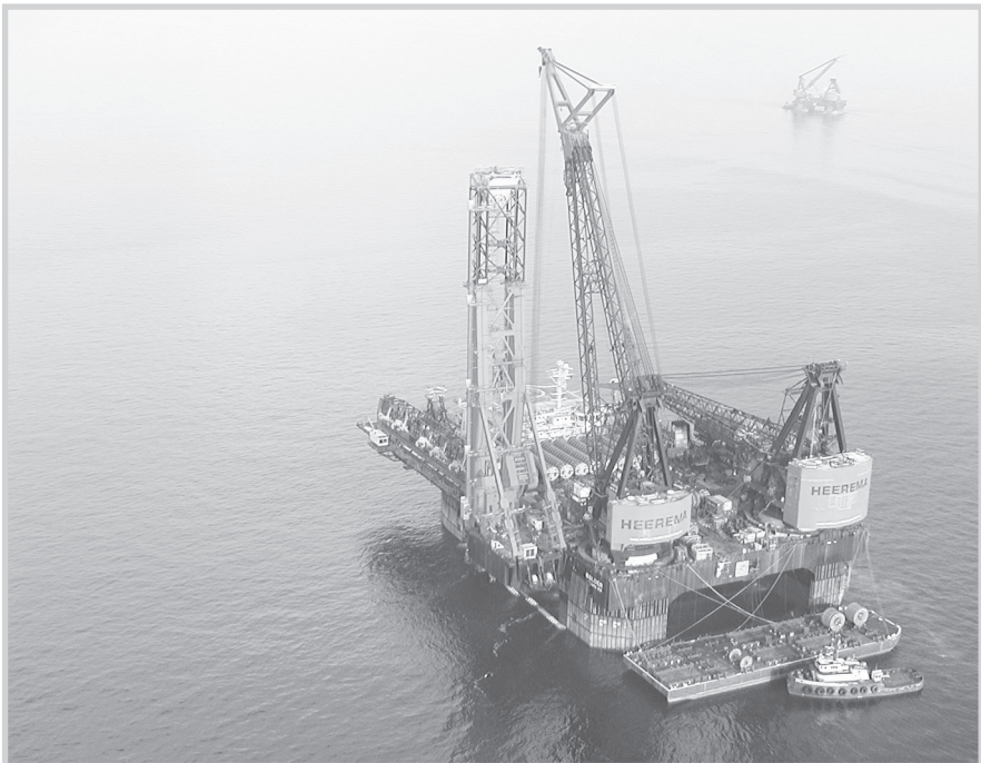
Fig. 7-6. J-lay barge (Courtesy Heerema Marine Contractors)
