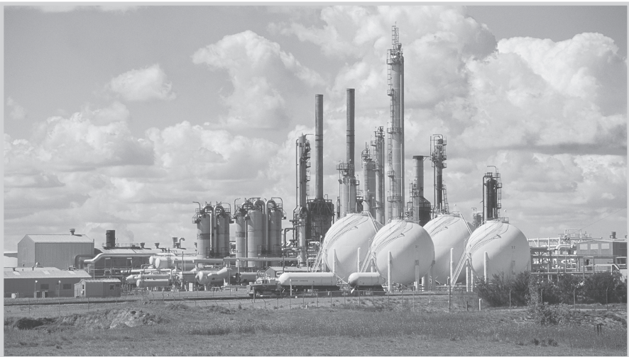
Fig. 1–4. Natural gas processing plant (Courtesy ConocoPhillips)
