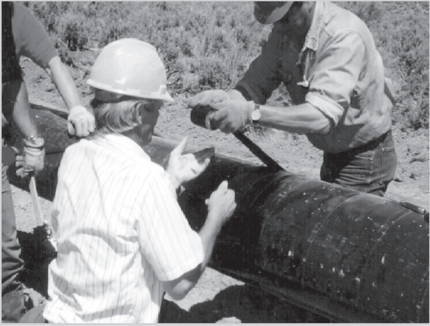
Fig. 11-3. Applying spiral wrapping tape to a pipe (Courtesy Corrosion Control Products Company)
