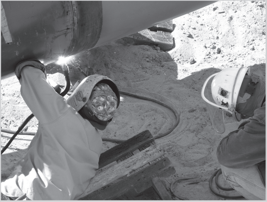
Fig. 13-5. Manual welding (Courtesy U.S. Pipeline, Inc.; photo by Adam Aronson)
