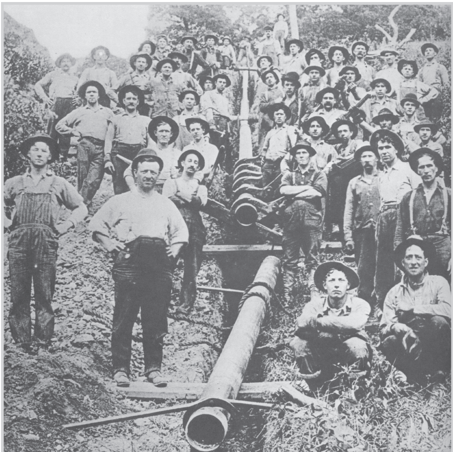
Fig. 2–6. A pipeline gang installing threaded pipe, circa 1890. The crews used long tongs to grip and turn the pipe. (Courtesy API and the Behring Center of the Smithsonian Institute)
