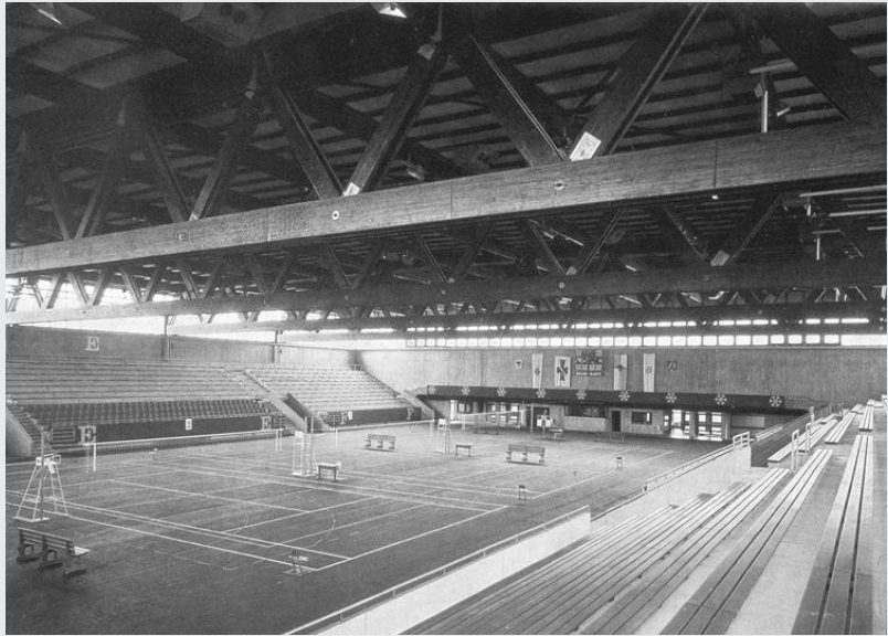
V-girder trusses supporting sports hall roof Types of trusses.
