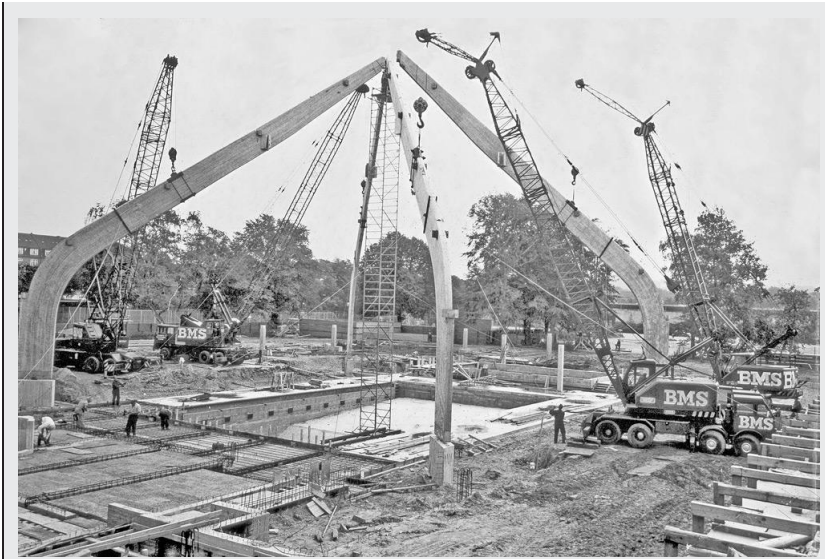
Erection of glulam portal frames
