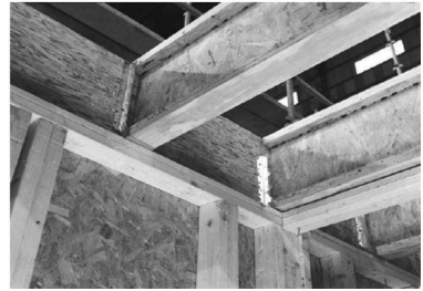
Fig. 2.23 Geometry of typical I-beams and metal web beams
