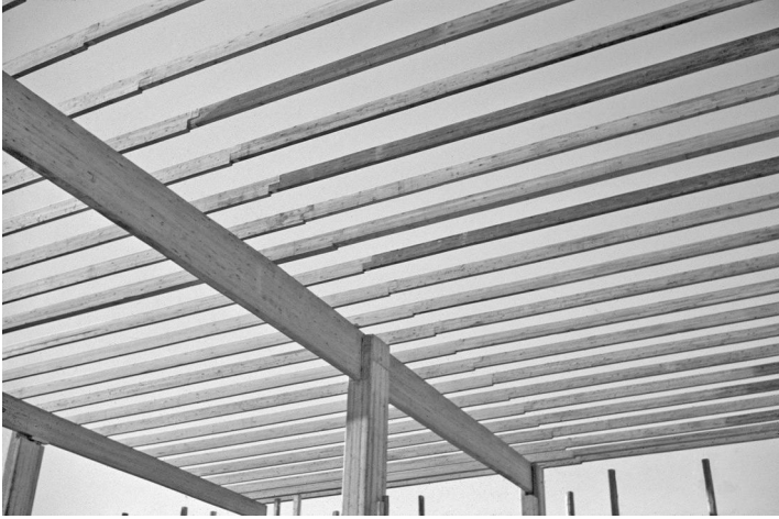
Fig. 3.1 Structural timber joists supported by glulam beams
