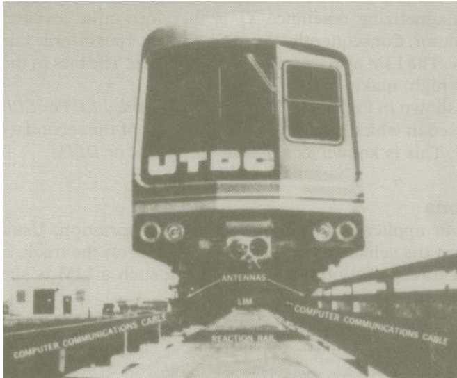
FIGURE 5.49 Transportation test vehicle using LIM.
