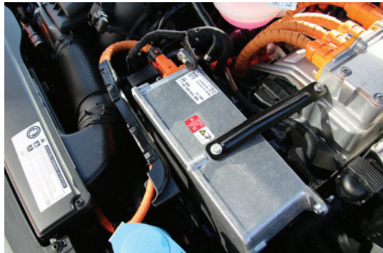
Figure 2.9 Orange high-voltage cables
