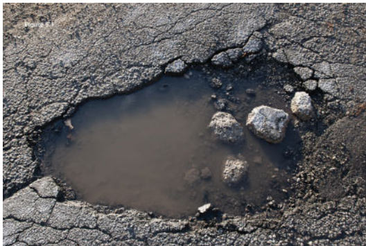
Figure 5.1 Pothole.
