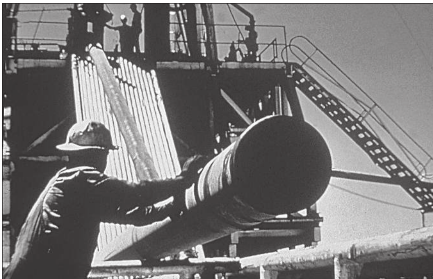
Plate 19–2. Casing being run up the pipe ramp onto the drill floor. (Courtesy of API.)
