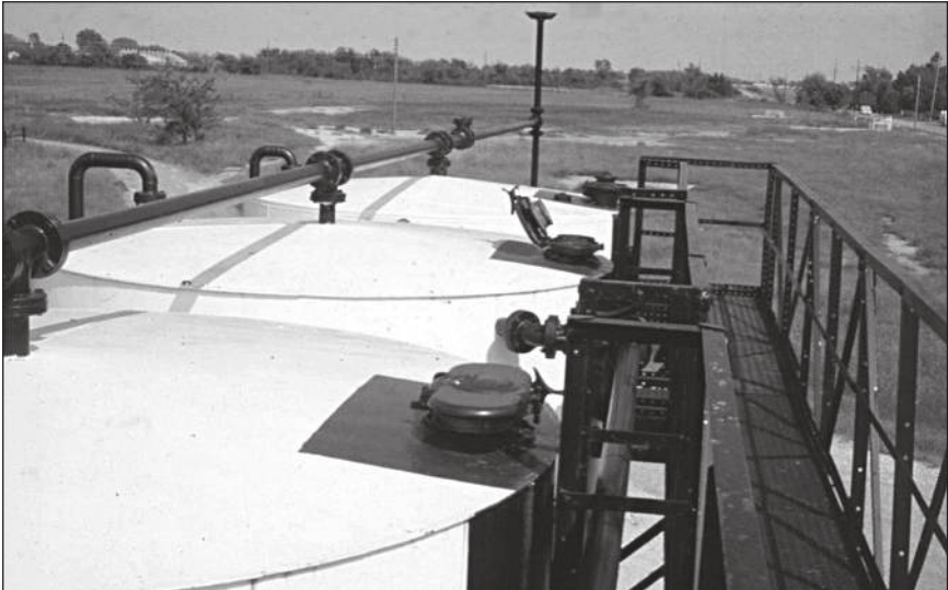
Plate 20-3. Top of stock tanks showing open and closed thief hatches and catwalk
