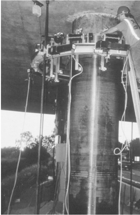
2.6 Automated winding of prepreg tow for seismic retrofit of columns.
