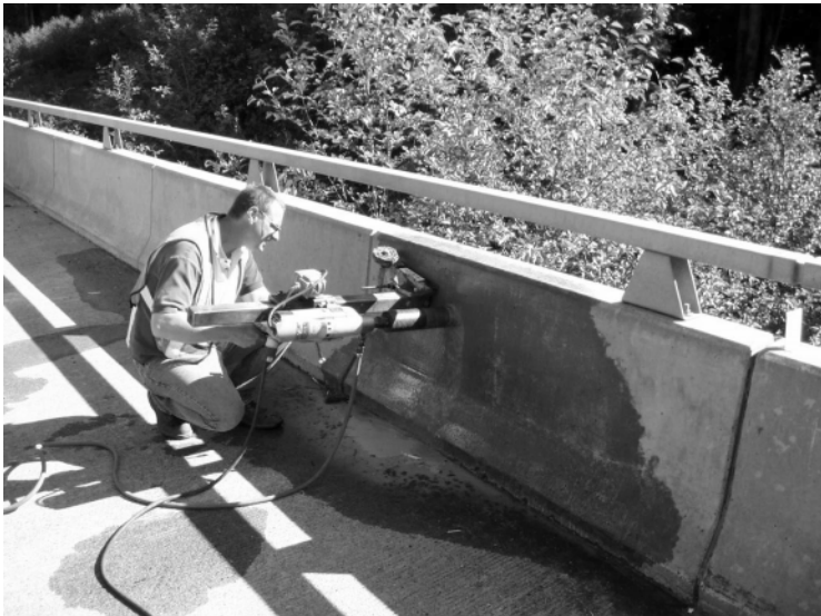
14.24 Waterloo Creek Bridge – core sample extraction.
