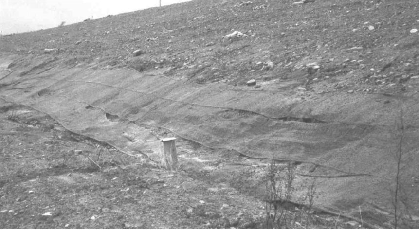
12.10 Vegetable fibre net on a landfill final cap.
