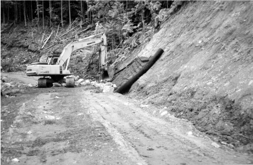
6.1 Cut-slope stabilization: geotextile filter and rock blanket.
