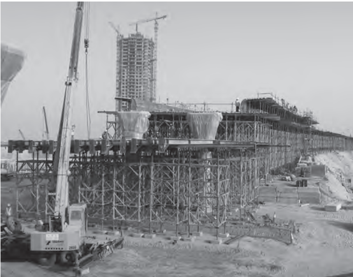
Figure 9.17 In situ box girder, construction on falsework
