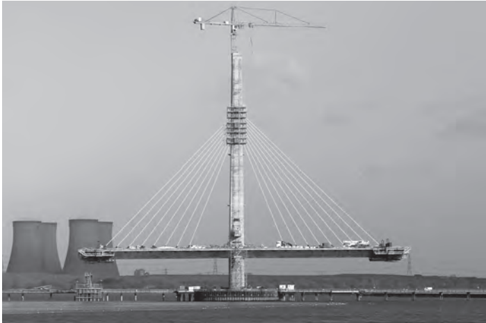
Figure 19.42 Mersey Gateway: deck construction (courtesy of Merseylink CJV)
