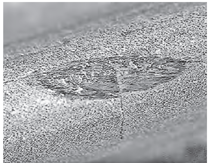
Figure 24.12 Fretting on contact surfaces leading to fretting fatigue failure in tendon wires (photograph courtesy of LCPC)
