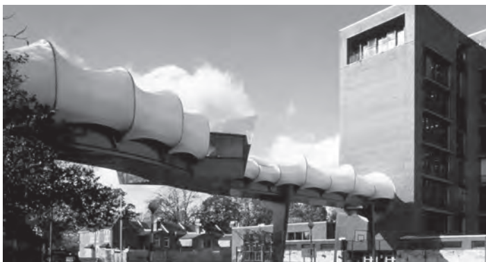
Figure 17.20 Covered steel bridge of sculpted plate and rolled sections (photograph courtesy of Techniker).
