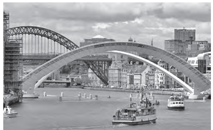
Figure 16.43 Gateshead Millennium Bridge – open position (image courtesy of Wilkinson Eyre Architects)
