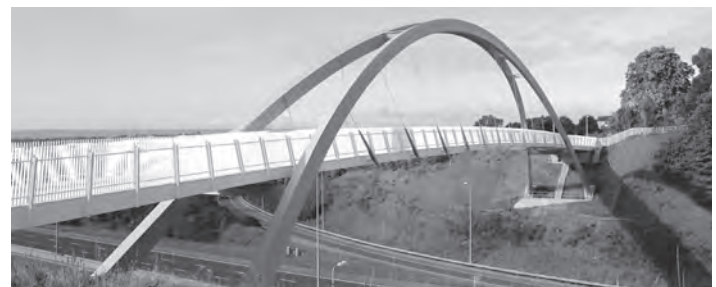
Figure 17.11 Completed bridge, showing the simple yet elegant structure over the motorway
