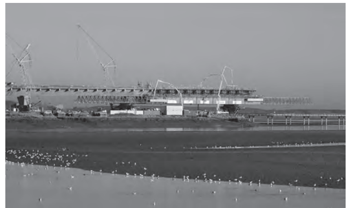
Figure 19.26 Movable scaffold system courtesy (courtesy of Merseylink CJV)
