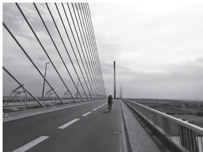
Figure 1.17 Brotonne Bridge, Sotteville, France
