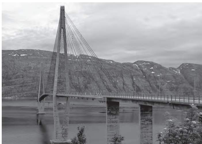
Figure 14.34 Helgeland Bridge, Norway (courtesy of Leonhardt, Andra und Partners)
