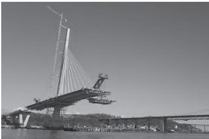
Figure 19.28 Queensferry Crossing: deck construction (courtesy of Transport Scotland)
