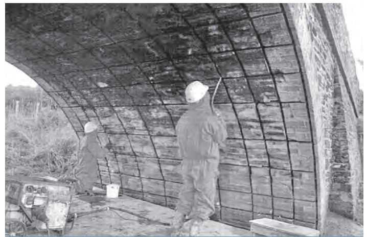
Figure 26.12 The MARS system under construction (courtesy of MARS)
