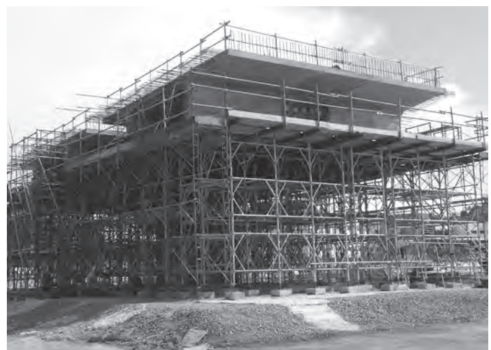
Figure 9.21 Balanced cantilever pier head segment casting
