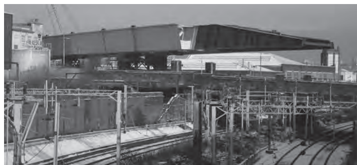
Figure 19.1 Bridge erection in Glasgow, Scotland, latitude 55.858°N; temperatures reached –18°C during the construction of the M74 extension (courtesy of Tony Gee)
