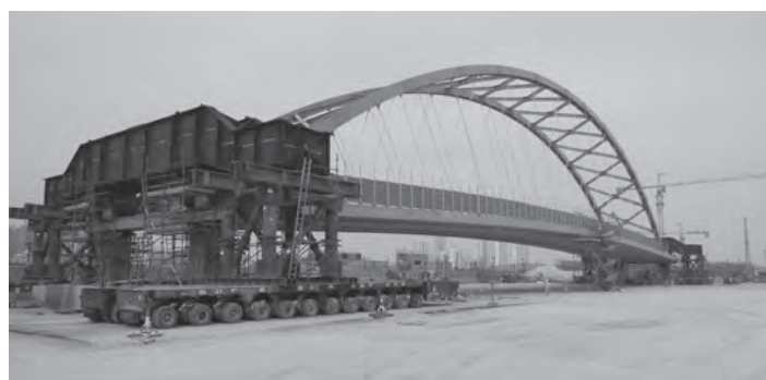
Figure 19.24 P954 flyover, Bahrain: bridge installation by SPMT (courtesy of Tony Gee)
