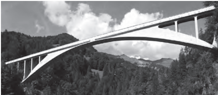
Figure 8.2 Salginatobel Bridge by Maillart
