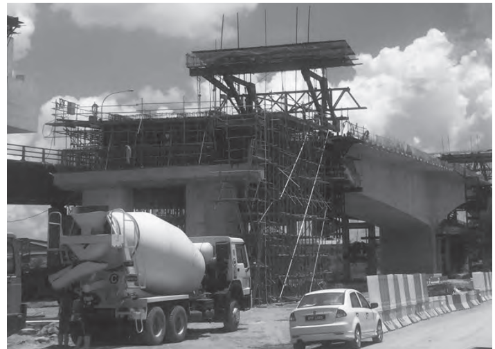
Figure 9.20 Balanced cantilever end span falsework
