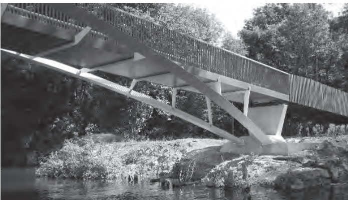
Figure 17.16 View showing key features of the bridge (© Knight Architects)
