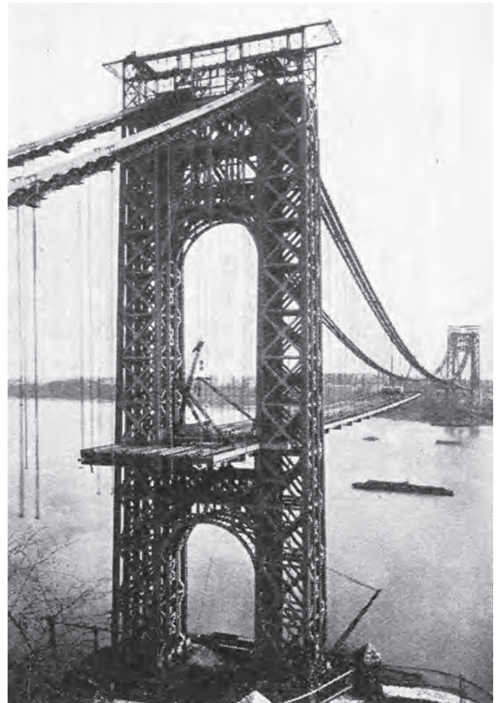
Figure 1.14 George Washington Bridge, New York
