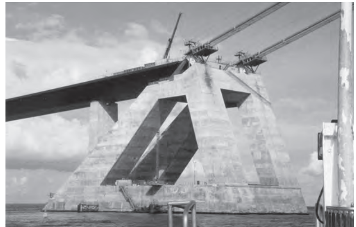
Figure 15.34 Storebælt East Bridge anchor block
