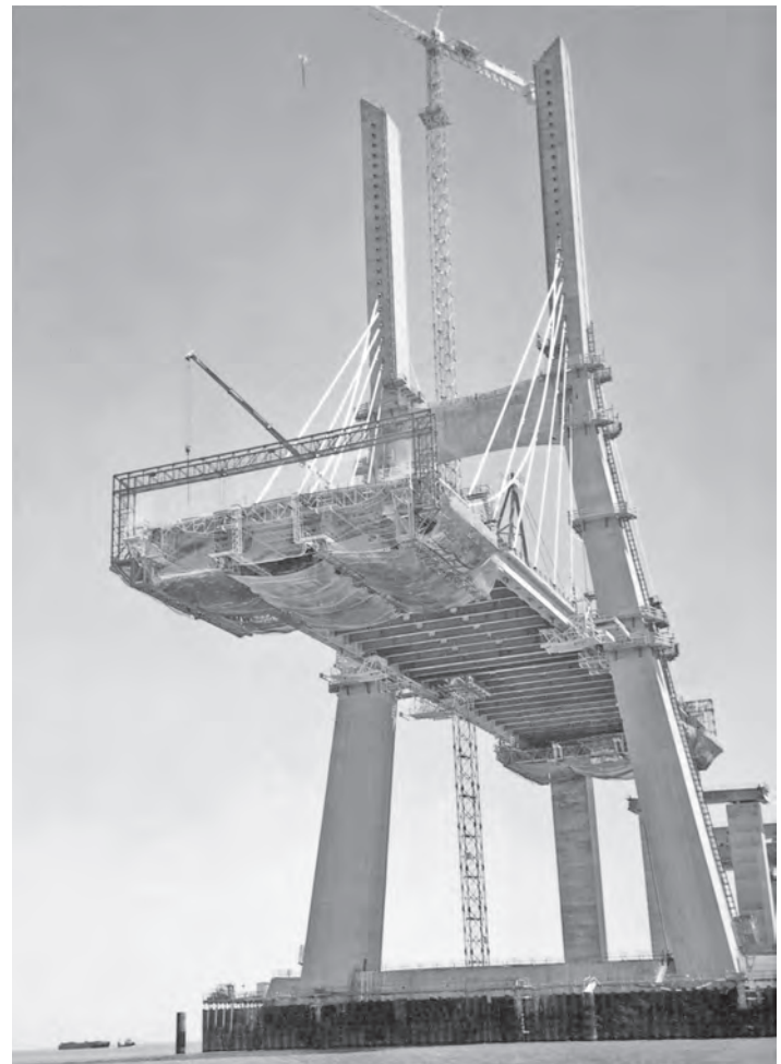
Figure 9.35 Vasco da Gama Bridge under construction
