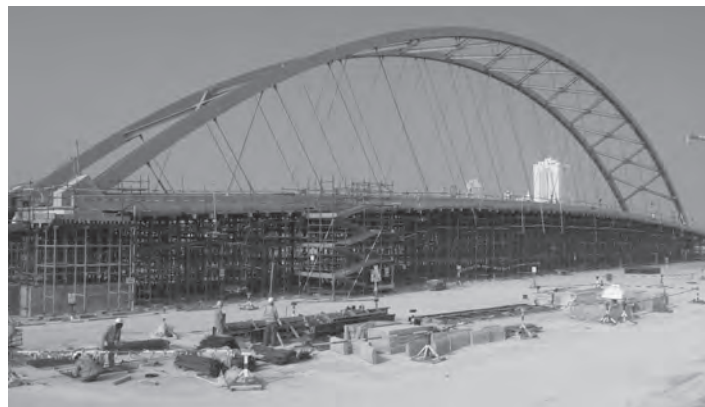
Figure 19.2 Bridge erection in Kuwait, latitude 29.321°N; Jamal Abdul Nasser Street Bridge (courtesy of Tony Gee)
