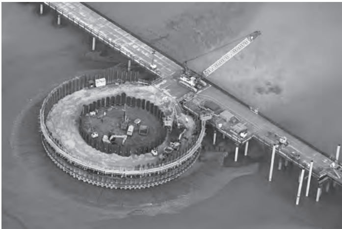
Figure 19.39 Excavating for pier foundation; access bridge in place (courtesy of Merseylink CJV)
