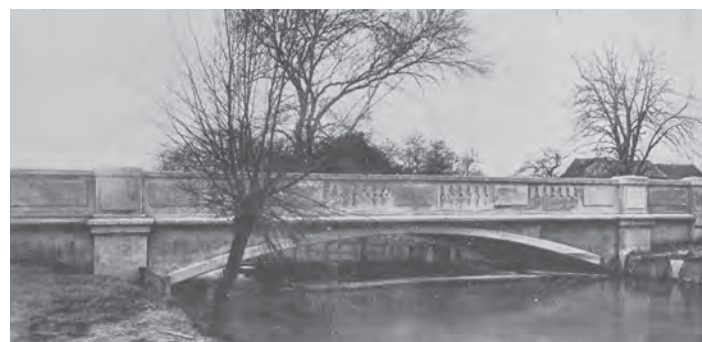
Figure 8.1 Beam-and-slab bridge over the River Wey, dating from 1913
