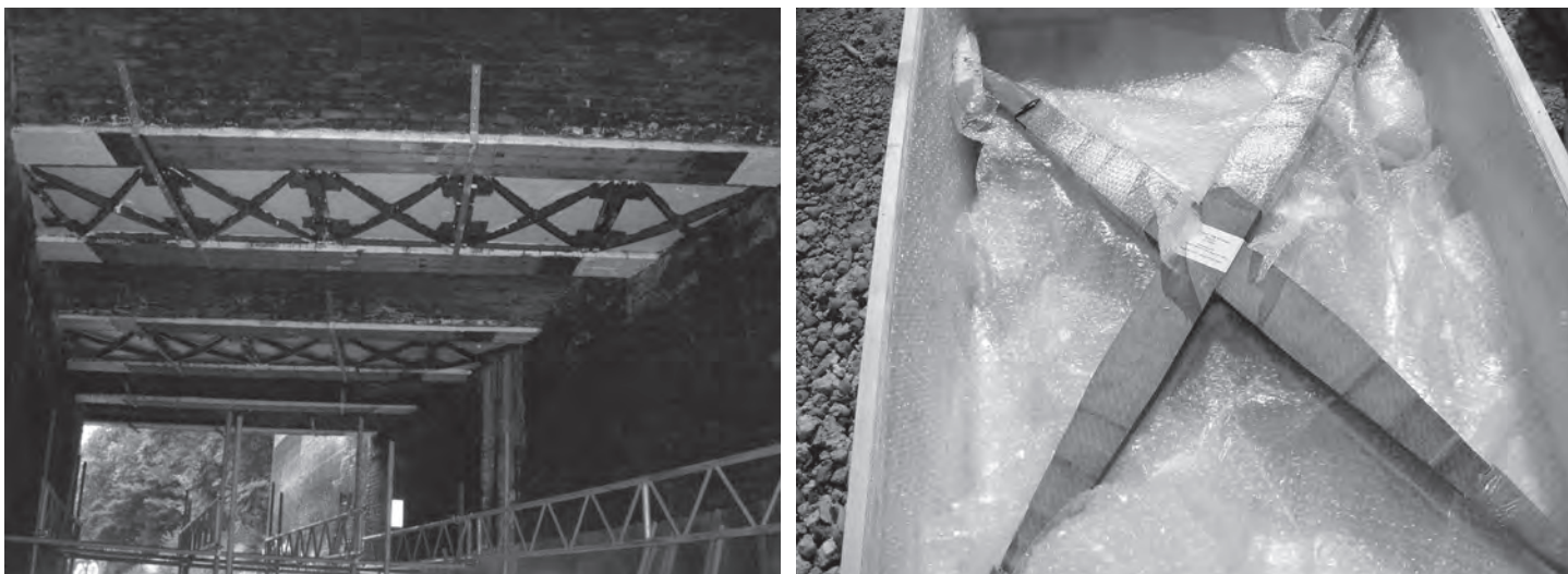
Figure 26.3 FRP plate bonding of cast iron girders and deck plate downstands (left) using curved tapered FRP cruciforms (right) (photograph courtesy of Mouchel Parkman)
