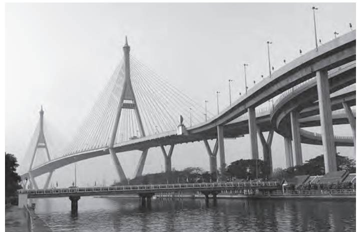
Figure 14.20 Industrial Ring Road Bridges, Thailand (courtesy of Ian Martin)
