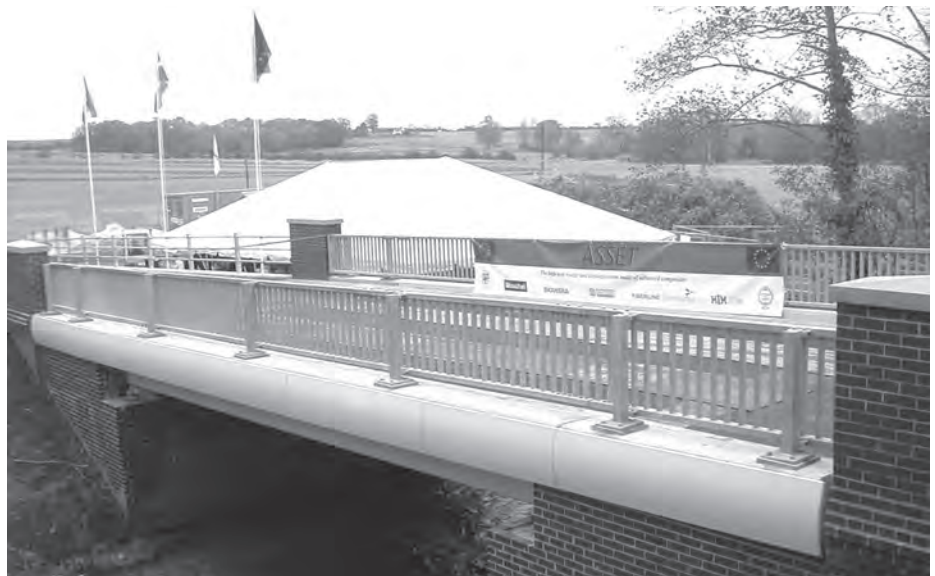
Figure 18.13 The GFRP deck and GFRP–CFRP main beam (span, 10 m) construction of the bridge over the River Cole, Oxfordshire, UK; the main beams were manufactured from pultruded GFRP composites and strengthened and stiffened with CFRP composite plates on the tension and compressive flanges of the beams. (photograph courtesy of Mouchel Parkman)
