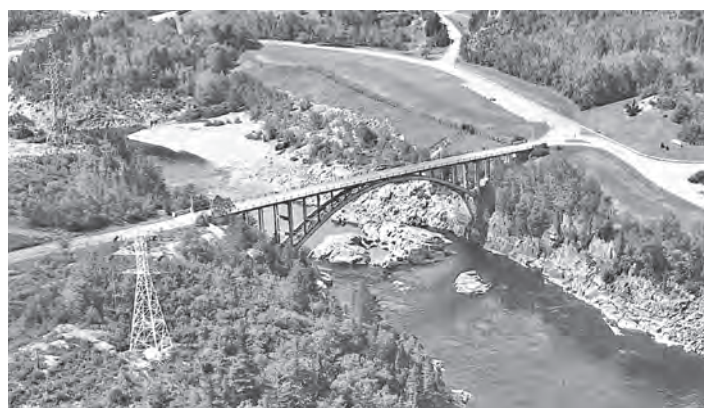
Figure 12.1 The Arvida Bridge over the Saguenay (courtesy of Alcan Aluminium Co. Canada)
