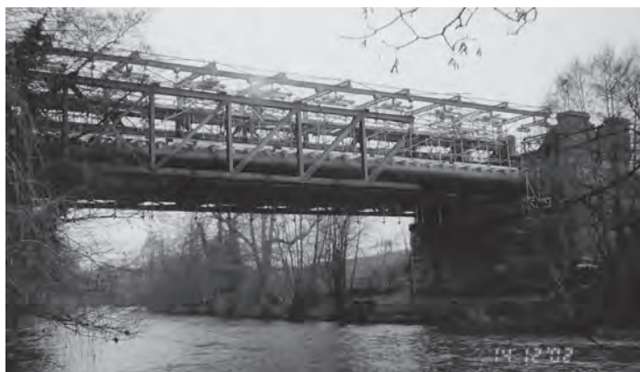
Figure 19.49 Steventon Viaduct: removal of existing bridge without the use of a crane, while supported on a temporary gantry (courtesy of VINCI)
