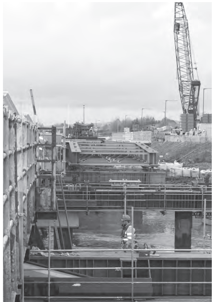
Figure 19.45 Temporary piers and temporary crosshead extensions (courtesy of Tony Gee)
