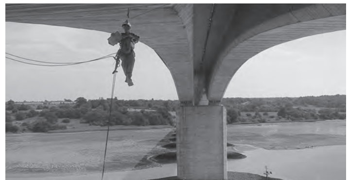
Figure 25.2 Inspection of bridge soffit over river
