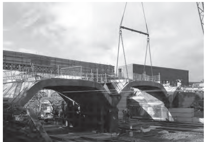
Figure 19.48 Sydney Road Bridge: demolition of reinforced concrete arch by saw cutting and crane lifting (courtesy of John Murphy and Sons)
