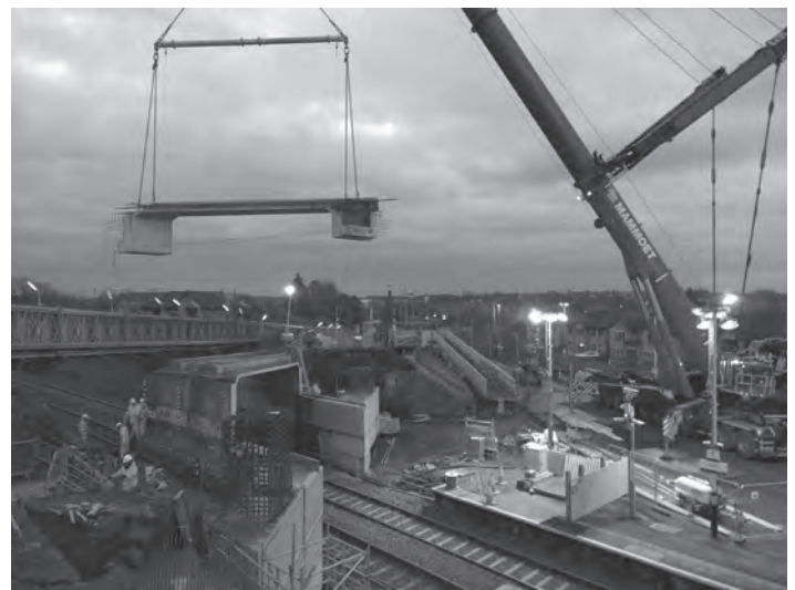
Figure 19.16 Over Bridge 59: abutments constructed using modular precast units (courtesy of Tony Gee)
