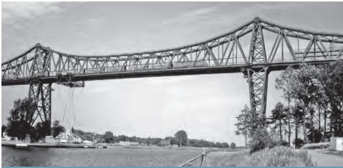
Figure 16.14 Transporter bridge at Rendsburg, Germany (photograph courtesy of J Baetke)
