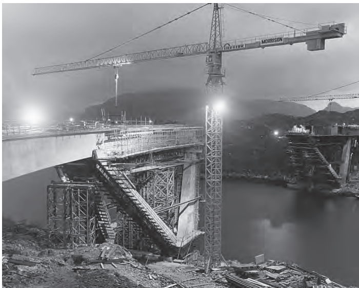
Figure 19.15 Kylesku Bridge construction; formwork and falsework to inclined piers (courtesy of Tony Gee)
