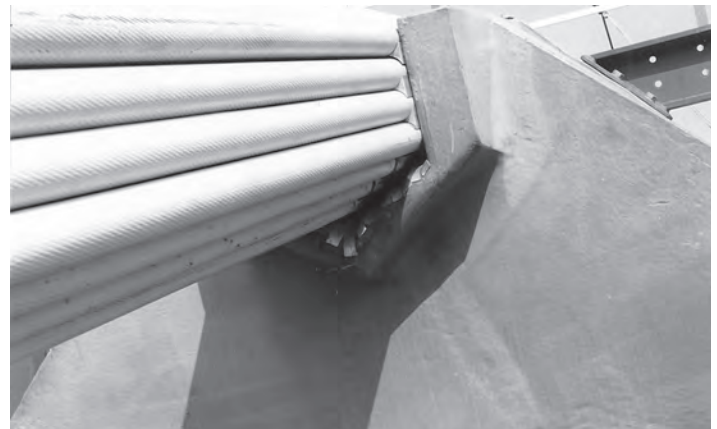
Figure 15.21 Tower saddle for spiral strand cable
