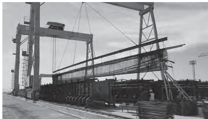
Figure 9.11 Casting bed for post-tensioned beam
