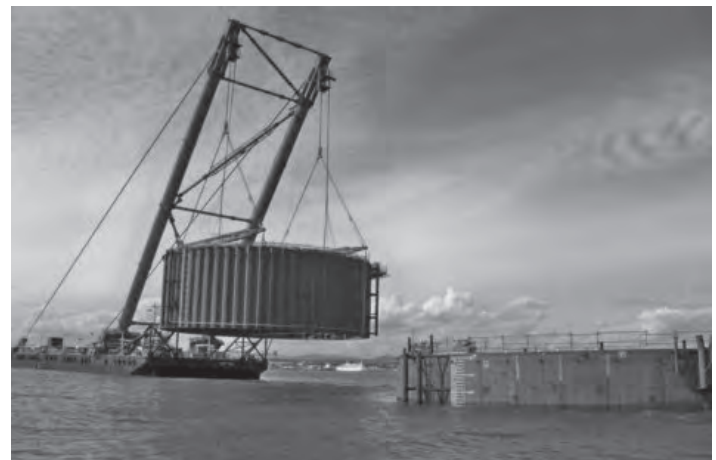
Figure 19.37 Base of caisson after installation (courtesy of FCBC)
