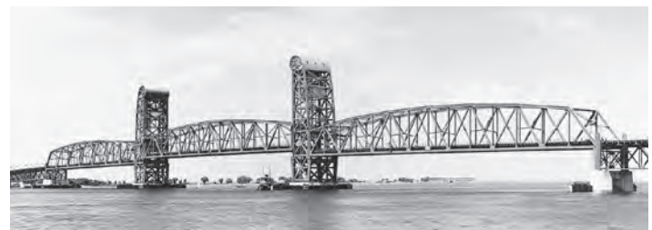
Figure 16.39 Marine Parkway–Gil Hodges Memorial Bridge (photograph courtesy of Hardesty & Hanover, LLP)
