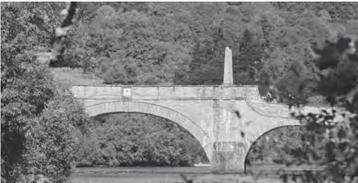
Figure 2.2 ‘Good ordinary’ – military infrastructure elevated to refined civic architecture: Tay Bridge, Aberfeldy, designed by William Adam (1733) for General George Wade’s Highlands military transport road (image © Jim Barton, https://www.geograph.org.uk/photo/4656319 )
