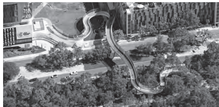
Figure 2.6 Bridge as a curated journey: Kids' Bridge, Perth WA (image: Stephen Heath/BEAM)
