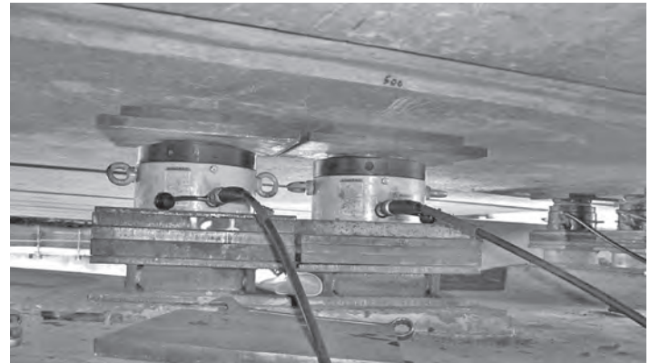
Figure 20.30 Jacking concrete deck (reproduced with permission © the Highways Agency)
