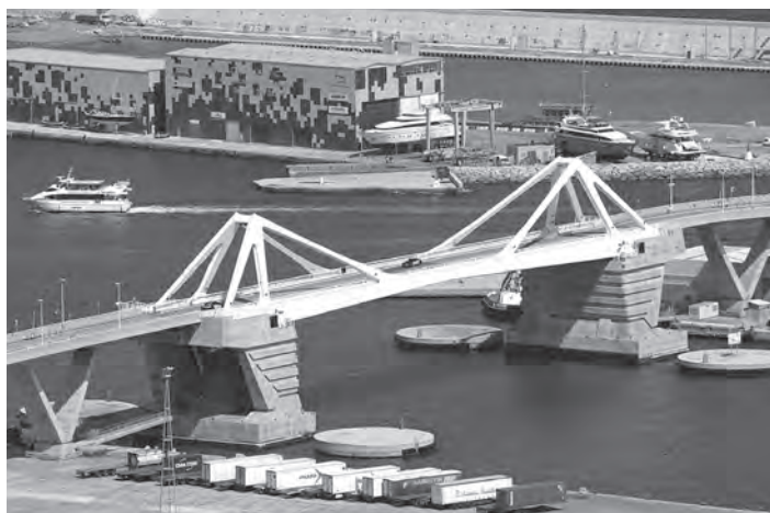
Figure 16.31 La Porta d'Europa bascule bridge (image courtesy of Arenas Associates)
