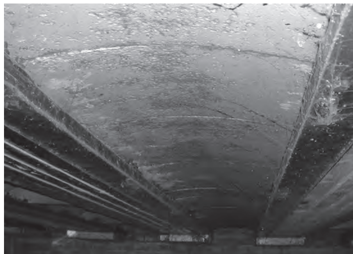
Figure 26.2 End anchorages and prestressed composites providing strengthening to Hythe Bridge in Oxford (photograph courtesy of Mouchel Parkman)
