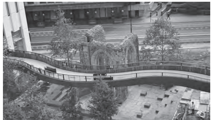
Figure 17.18 Curved footbridge, showing how the structure blends within its environment (© Brookfield Properties)
