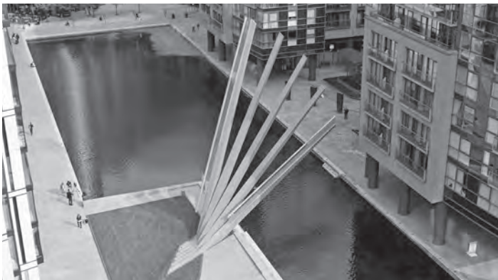
Figure 17.27 Bridge during opening (© Edmund Sumner)
