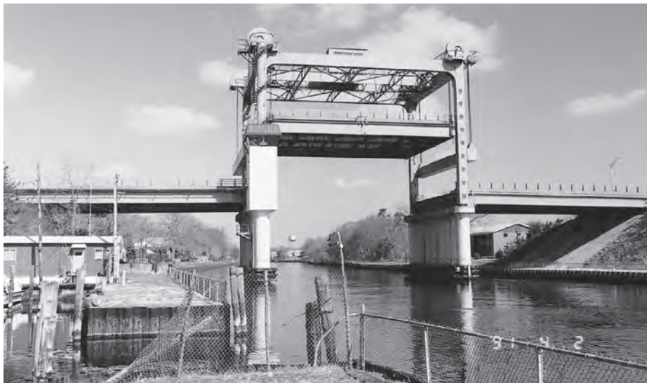
Figure 16.40 New Jersey Route 13 Bridge (photograph courtesy of C Birnstiel)
