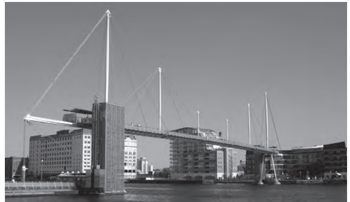
Figure 2.4 Historic structure type reinterpreted: Royal Victoria Dock Bridge, London (image: Liline sur Flickr, https://commons.wikimedia.org/wiki/File:Royal_Victoria_Dock_Bridge.jpg )
