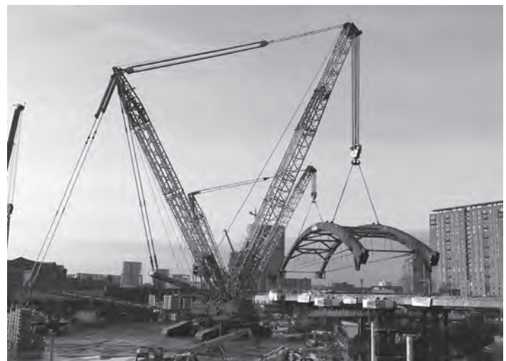
Figure 19.4 Ordsall Chord Bridge installation (Skanska BAM): a substantial piled reinforced concrete slab was required to provide an adequate working platform for the operation of a 1350t crawler crane, with operational track bearing pressures of 600 kPa (courtesy of Tony Gee)
