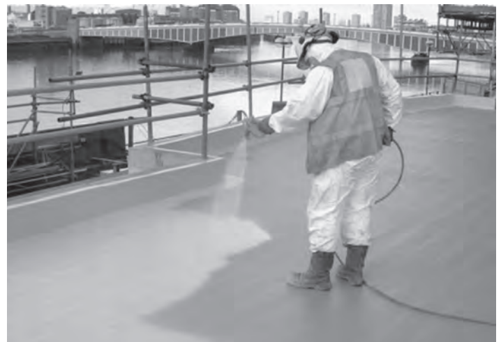
Figure 21.19 Application of bridge deck waterproofing
