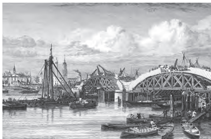
Figure 1.6 John Rennie's New London Bridge – under construction
