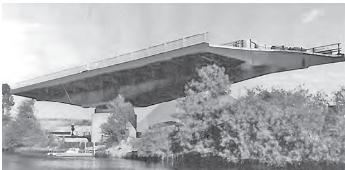
Figure 16.34 Næstved Swing Bridge (image courtesy of the Danish Road Directorate)
