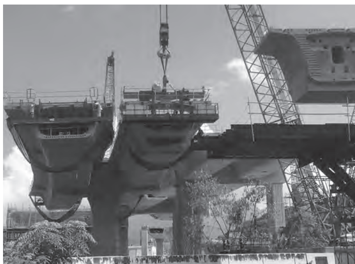
Figure 9.22 Precast segmental erection by crane
