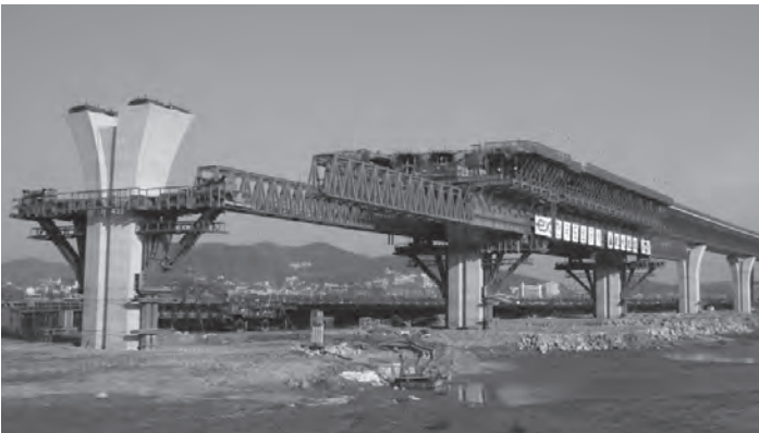
Figure 9.18 In situ box girder cast on self-launching truss
