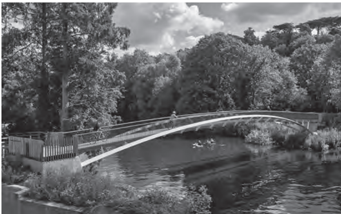
Figure 2.10 Order, symmetry and clear delineation: Taplow Bridge, Buckinghamshire (image: © Lance McNulty/Knight Architects)
