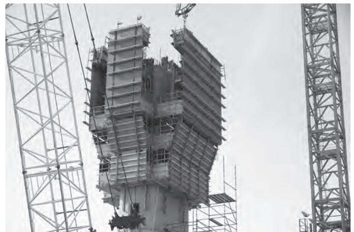
Figure 19.9 Independently supported pier formwork (courtesy of Merseylink CJV)
