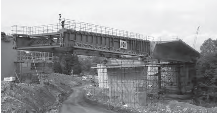
Figure 9.31 Incrementally launched box girder
