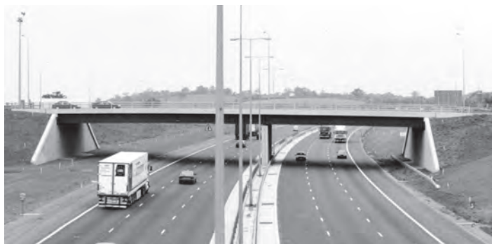
Figure 11.5 Continuous steel–concrete bridge spanning the M5 motorway, UK
