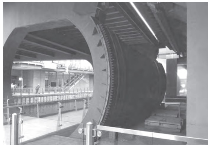
Figure 16.6 Bellmouth Passage Road Bridge, London, UK
