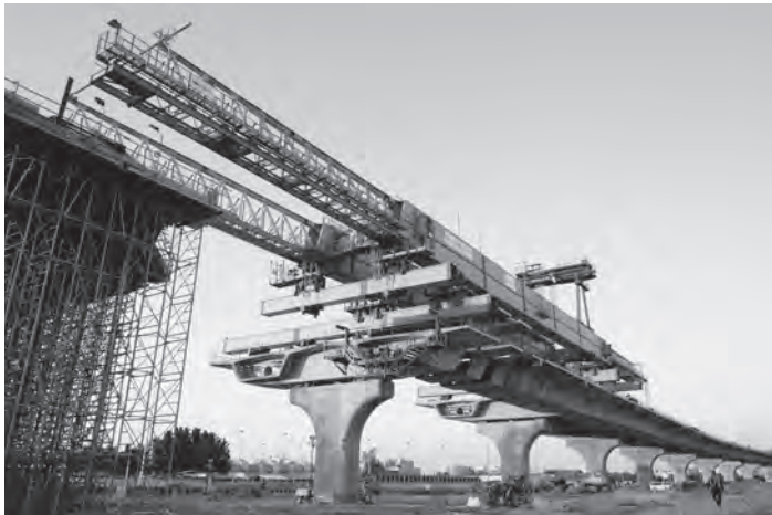
Figure 19.27 Jamal Abdul Nasser Street Bridge: overhead gantry supporting precast elements (courtesy of Tony Gee)
