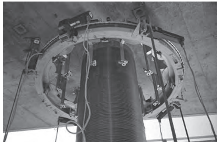
Figure 18.7 Column wrapping using XXsys technique (by kind permission of XXsys Technologies, Inc., San Diego, CA, USA)
