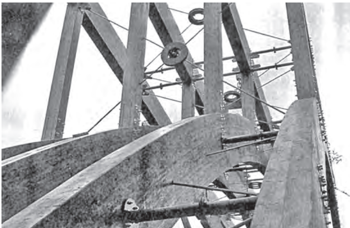
Figure 13.8 Mur River Bridge – bracing (Pischl and Schickhofer, 1993)
