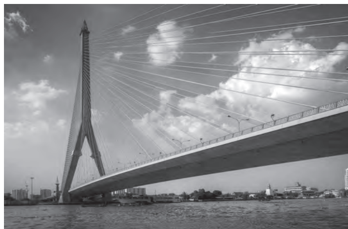
Figure 14.6 Rama VIII Bridge, Bangkok (courtesy of Yee Associates)
