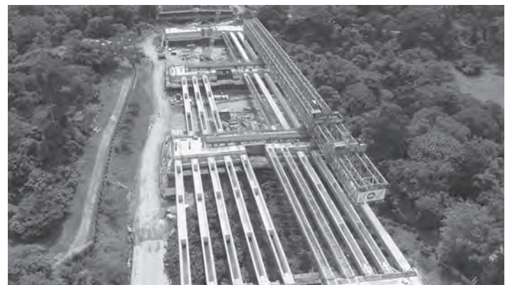
Figure 9.13 Gantry for erection of precast beams
