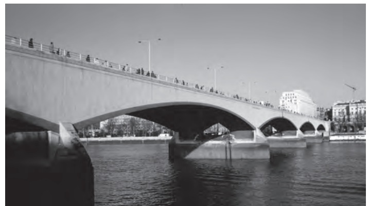
Figure 8.9 Waterloo Bridge: a haunched reinforced concrete box girder
