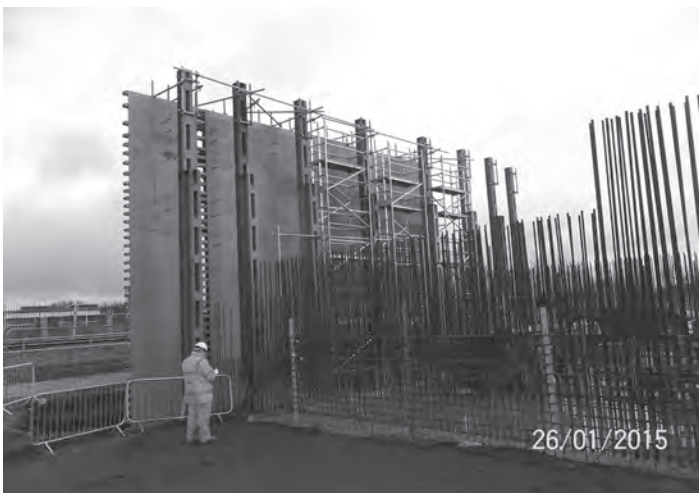
Figure 19.11 Bridge abutment being constructed adjacent to live railway: temporary vertical posts support formwork, which in turn supports reinforcement and provides a protection screen between the workforce and the railway – access for fixing the reinforcement is from the rear of the wall; the front face must be fixed before the rear face (courtesy of Balfour Beatty and Tony Gee)
