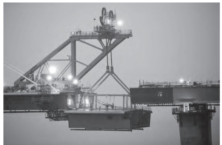
Figure 19.41 Queensferry Crossing: deck construction (courtesy of Transport Scotland)
