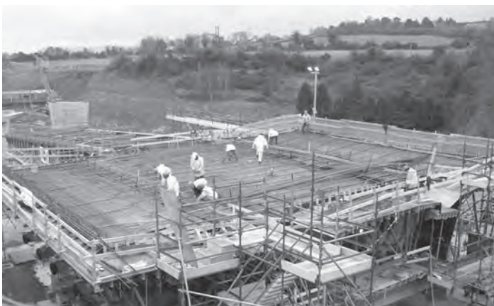
Figure 9.32 Casting area for launched box girder
