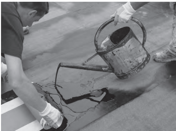
Figure 21.22 Application of hot-melt bitumen
