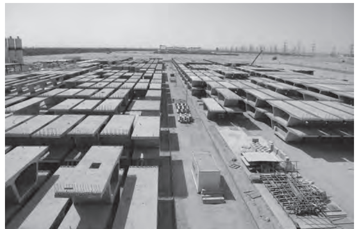
Figure 19.3 Site storage for precast bridge segments (courtesy of Tony Gee)
