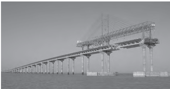
Figure 9.37 Bubiyan Bridge under construction (courtesy of Bouygues)
