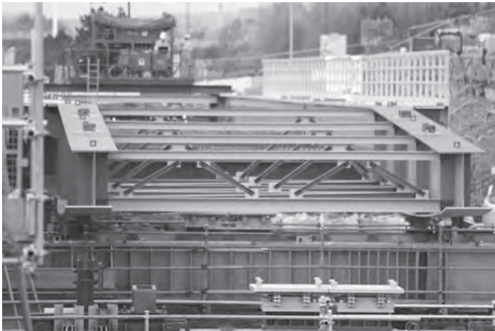
Figure 19.46 Launching nose, launching equipment rollers, foundations, jacks and anchorages and sliding system (courtesy of Tony Gee)
