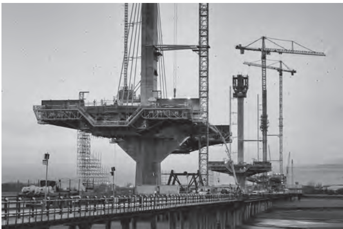
Figure 19.43 Mersey Gateway: deck construction (courtesy of Merseylink CJV)
