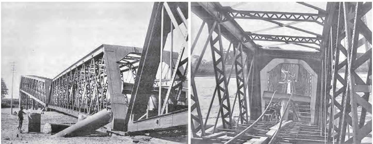
Figure 6.1 Damage to the Nagara Gawa Railway Bridge, Gifu (Japan) earthquake of 28 October 1891 (courtesy of INGV – National Institute of Geophysics and Volcanology, Italy)
