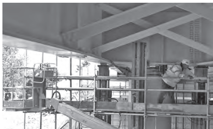
Figure 20.27 Jacking down off jacking trestle (reproduced with permission © the Highways Agency)
