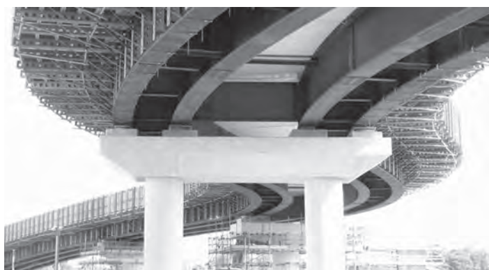
Figure 19.22 Formwork for construction of in situ concrete deck between girders: wet concrete is supported by permanent formwork, cantilever edges of deck are supported by removable RMD Paraslim brackets (courtesy of RMD)
