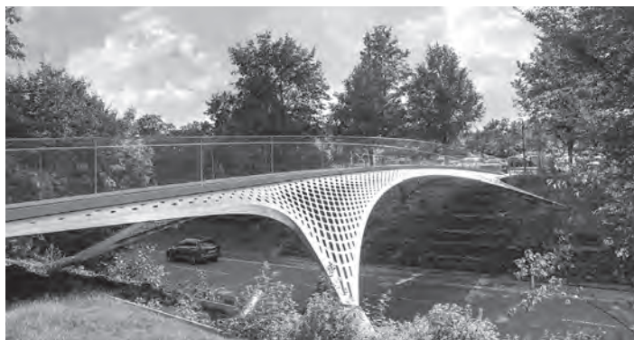
Figure 17.12 Shallow arch effect with glass parapet providing minimal visual impact (© sbp/Andreas)
