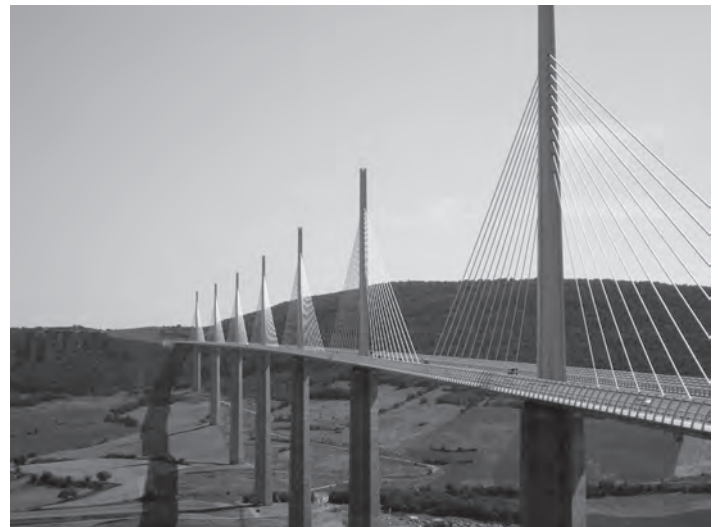
Figure 1.23 The A75 Clermont–Ferrand highway bridge (the Millau Viaduct)
