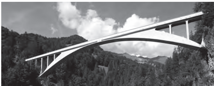
Figure 1.15 Salginatobel Bridge – one of the most aesthetic arch spans of Maillart (courtesy of EH)
