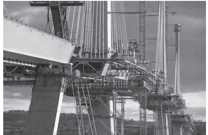
Figure 19.40 Queensferry Crossing: deck construction (courtesy of Transport Scotland)
