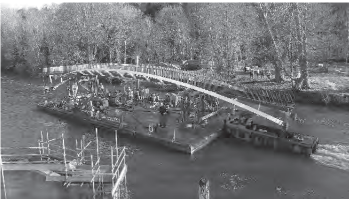
Figure 17.17 Entire bridge transported for installation (© Knight Architects)
