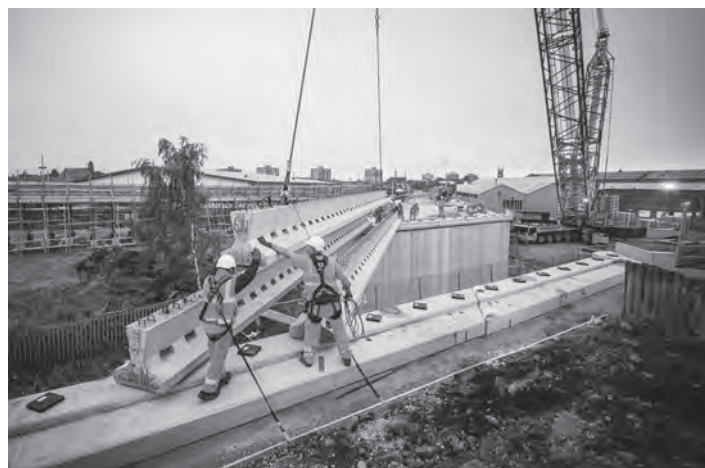
Figure 19.20 Placing precast concrete beams, Richmond Street Bridge (courtesy of John Murphy and Sons)
