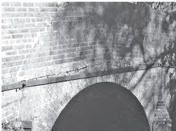
Figure 26.14 Arch strengthening with tie-bars
