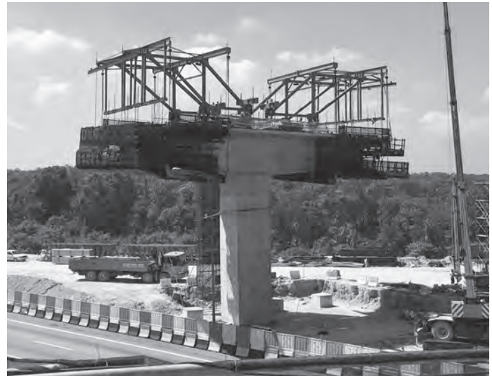
Figure 9.19 In situ balanced cantilever construction
