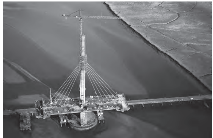
Figure 19.29 Mersey Gateway: deck construction (courtesy of Merseylink CJV)
