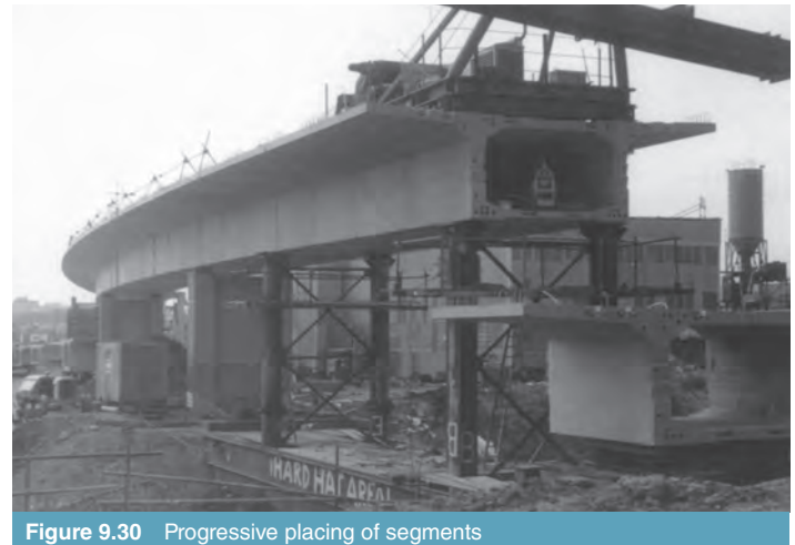
Figure 9.30 Progressive placing of segments
