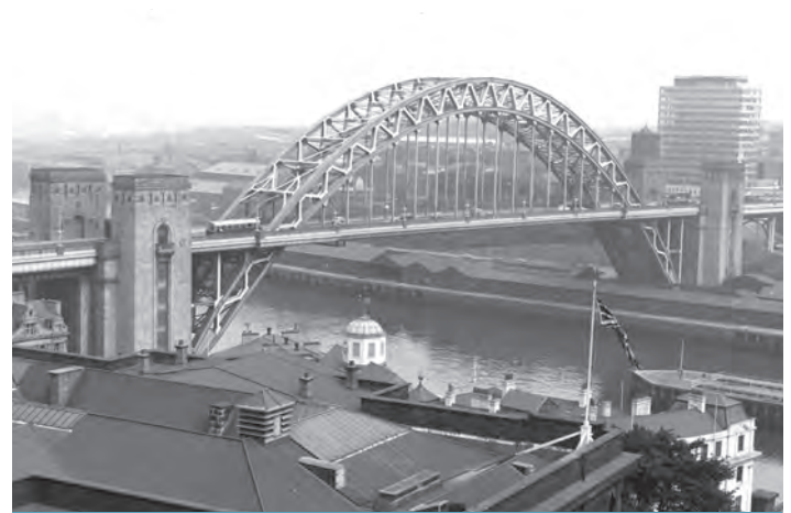
Figure 1.12 Tyne Bridge, Newcastle upon Tyne
