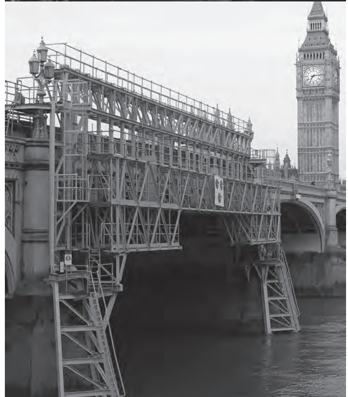
Figure 19.5 Temporary works doubling as (a) lifting beam and (b) temporary support during repairs to the fascia of Westminster Bridge (courtesy of Tony Gee)
