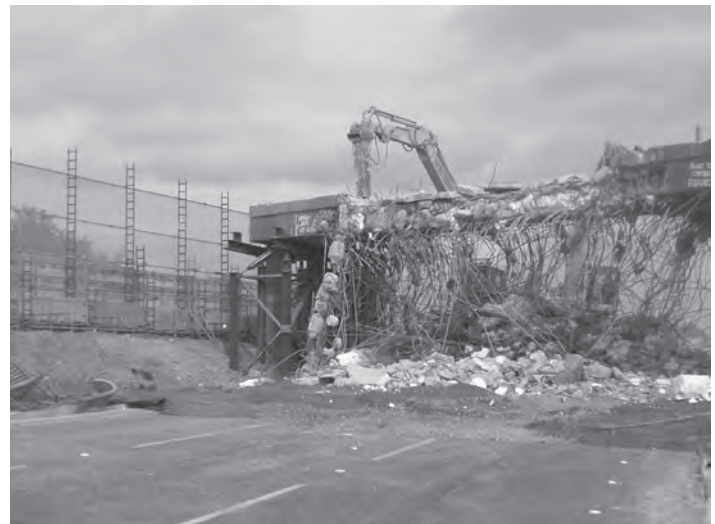
Figure 19.47 Bridge demolition M5 Jn 12 (courtesy of Norwest Holst )
