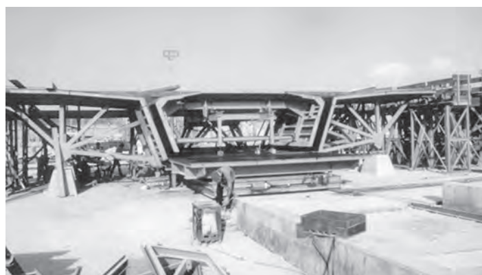
Figure 9.25 Precast segment casting cell
