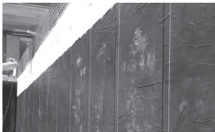
Figure 21.21a Self-adhesive bituminous membrane
