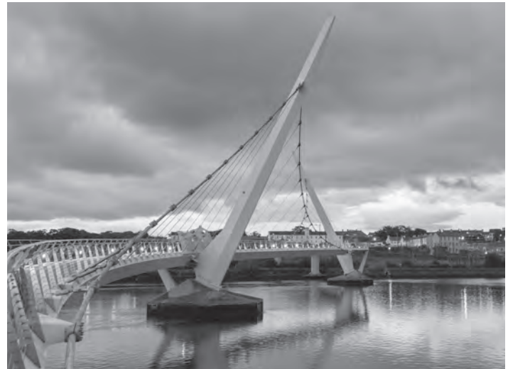
Figure 17.25 The two sloping pylons supporting the deck
