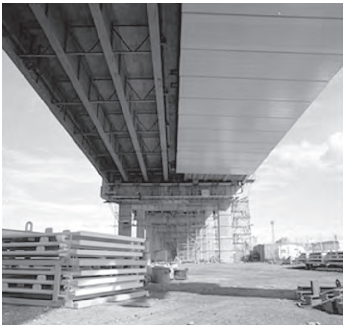
Figure 18.16 Maunsell Caretaker system used on the A19 Tees Viaduct at Middlesbrough (by kind permission of Maunsell Structural Plastics, Beckenham, Kent, UK)
