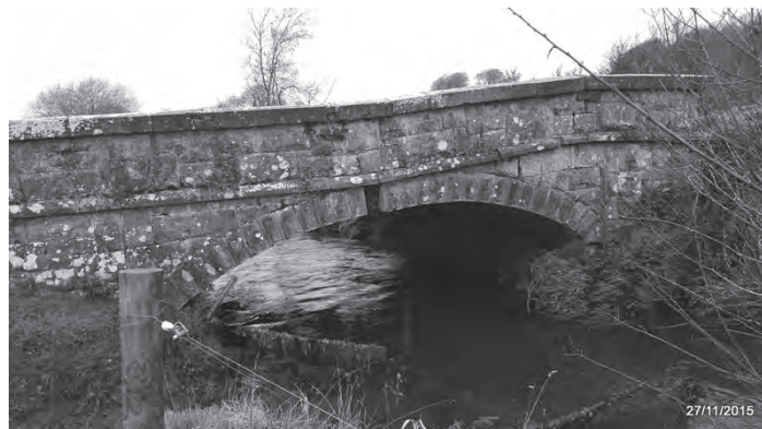
Figure 25.10 Deformed masonry arch
