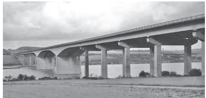
Figure 1.16 Medway Bridge, Kent
