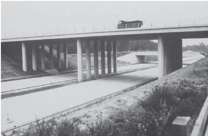
Figure 7.9 Spill-through abutment (in fill, to left) and piers, M25, Wisley, UK (before widening and central protection barrier)
