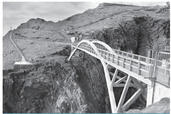
Figure 8.17 Mizen Head Bridge, a new bridge replicating the original structure
