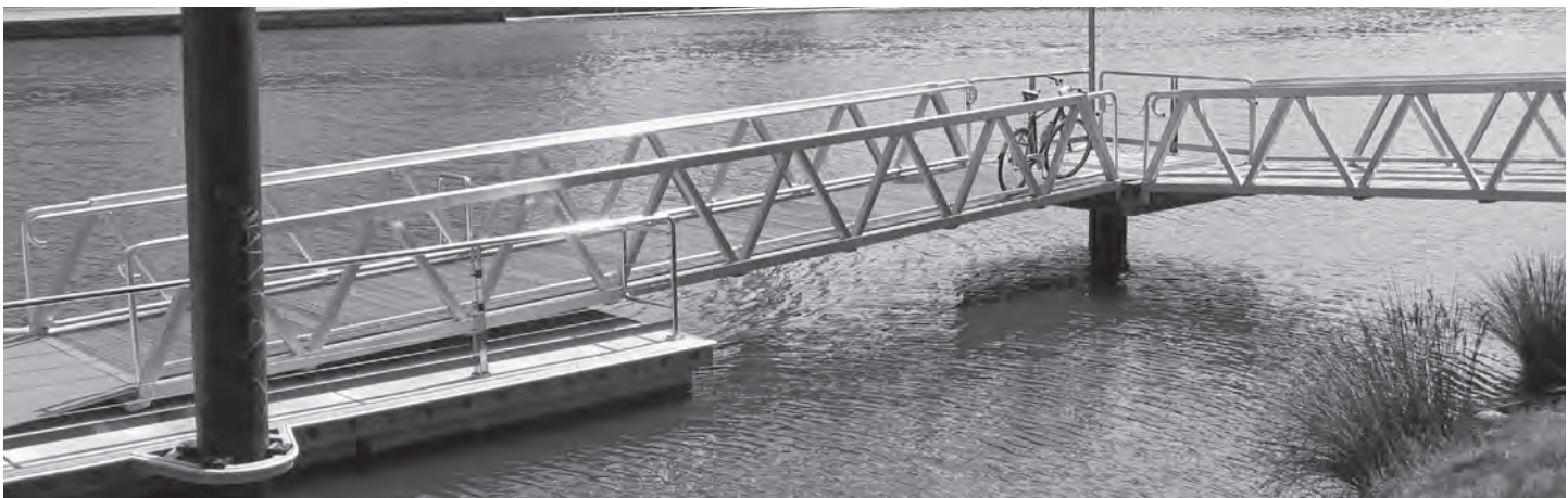
Figure 12.8 Typical marine link bridge (photo courtesy of P Tindall)
