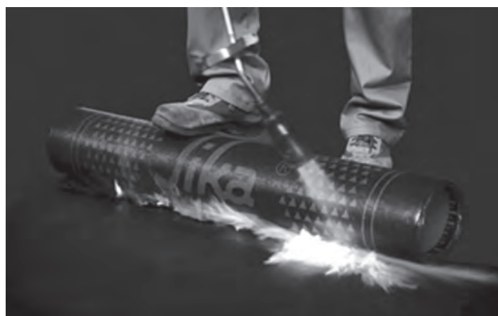
Figure 21.20 Application of torch-applied bituminous membrane
