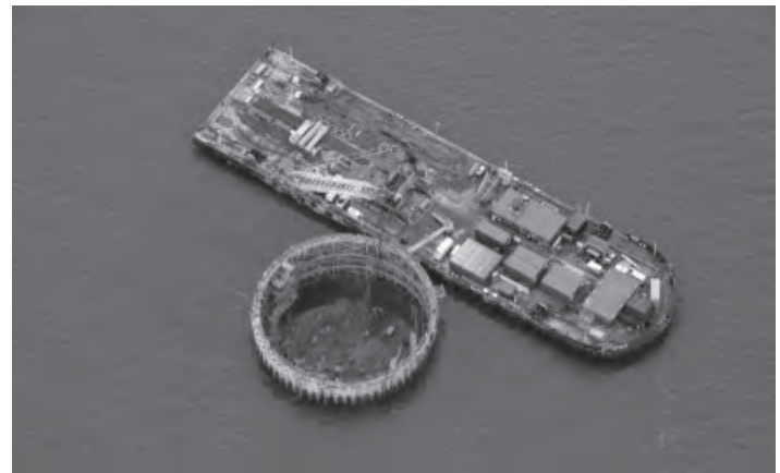
Figure 19.36 Installation of top single-skin caisson on permanent double-skin caisson before sinking (courtesy of FCBC)
