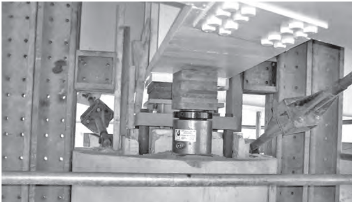
Figure 20.28 Jacking steel diaphragm beam, showing transverse restraints (reproduced with permission © the Highways Agency)
