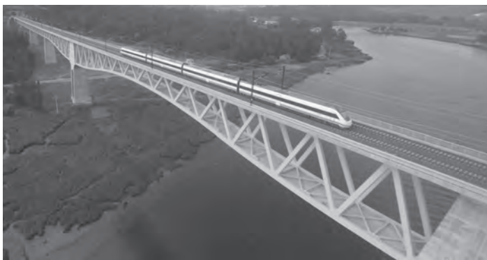
Figure 11.8 Ulla River composite truss viaduct for high-speed railway
