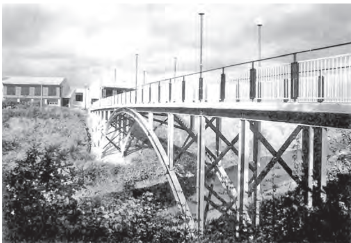
Figure 13.4 Chippingham Street footbridge (Taylor, 1995)
