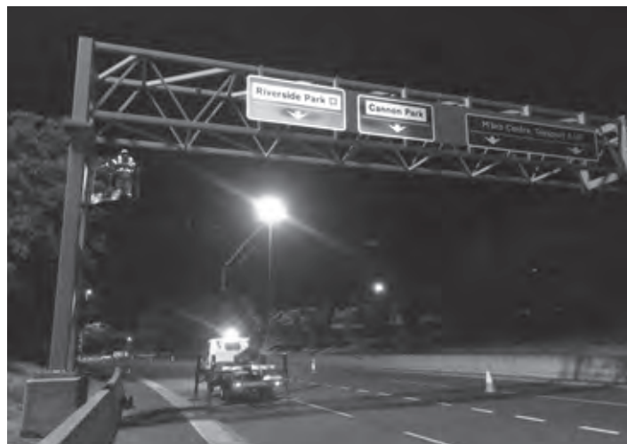
Figure 25.3 Access using mobile elevated work platform during bridge inspection
