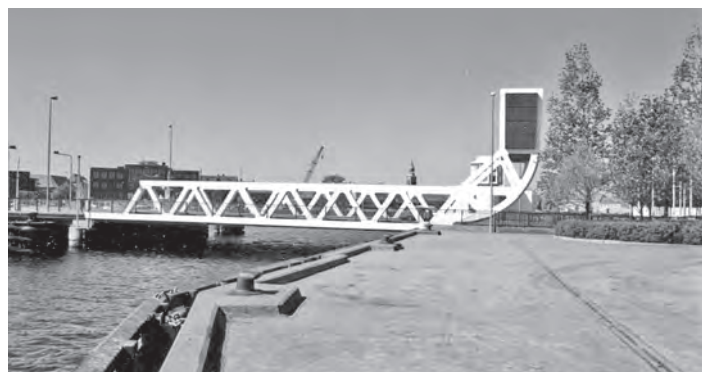
Figure 16.32 Halsskov Bridge (photograph courtesy of C Birnstiel)
