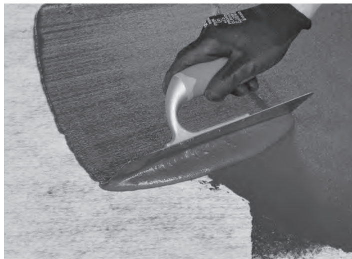
Figure 21.23 Application of cold-applied bitumen
