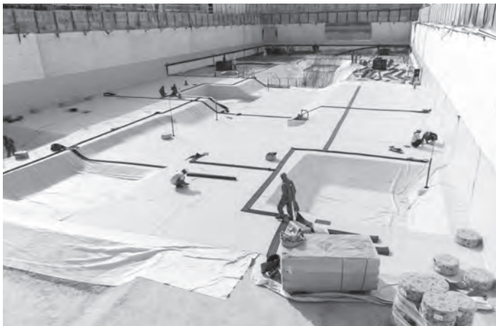
Figure 21.24 Application of loosely laid sheet membrane
