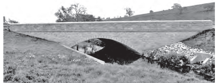
Figure 13.3 Monk New Bridge
