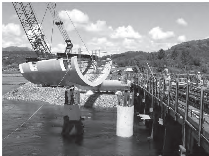
Figure 7.20 Precast shell for crosshead being installed
