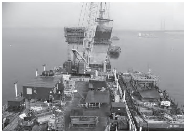
Figure 19.8 Independently supported pier formwork: Queensferry Crossing (courtesy of FCBC)
