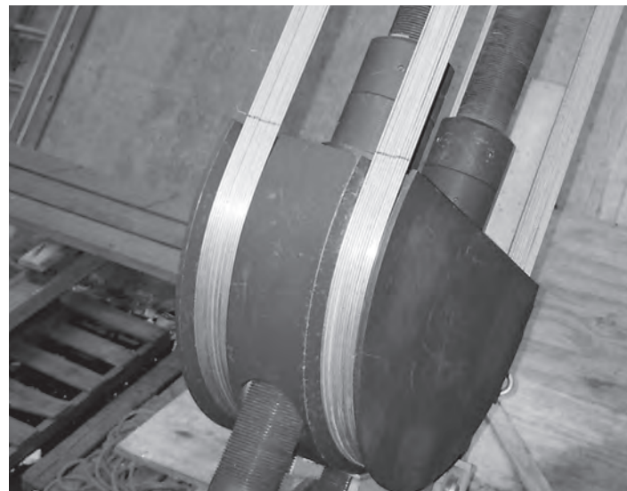
Figure 15.4 Anchorage termination for spun cable
