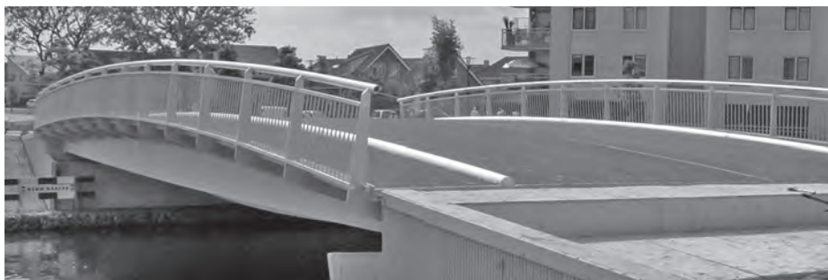
Figure 12.2 Raalte Verkeersbrug (courtesy of Bayards Aluminium Constructions BV, the Netherlands)
