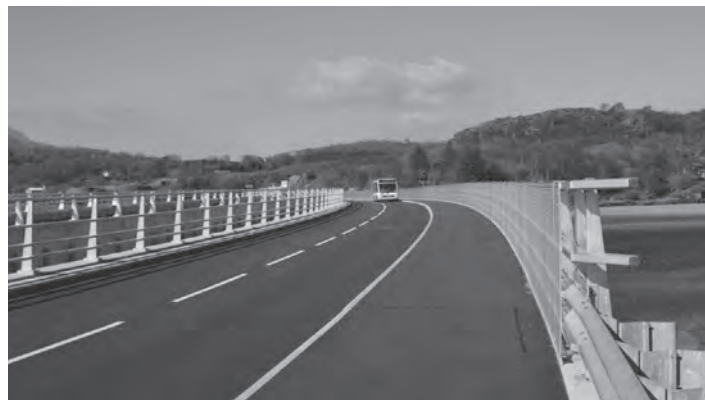
Figure 21.3 Metal parapet with and without fencing
