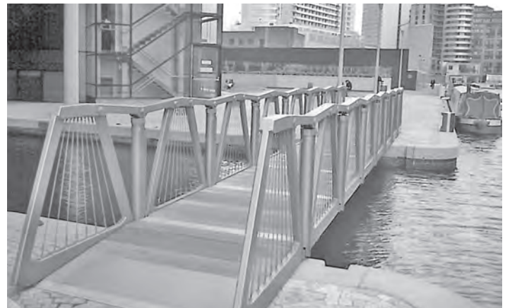
Figure 16.15 Folding pedestrian bridge at Paddington Basin, London, UK (photograph courtesy of C Birnstiel)
