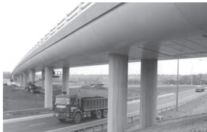
Figure 18.15 Approach road to the Second Severn Crossing, showing the Maunsell composite enclosure and fairings (by kind permission of Maunsell Structural Plastics, Beckenham, Kent, UK)
