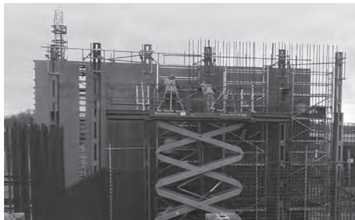
Figure 19.7 Bridge abutment with access provided by mobile elevated working platform (MEWP) (courtesy of BBCL)
