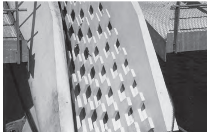
Figure 15.25 Splay saddle trough separators
