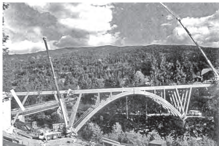
Figure 13.7 Mur River Bridge – construction (Pischl and Schickhofer, 1993)
