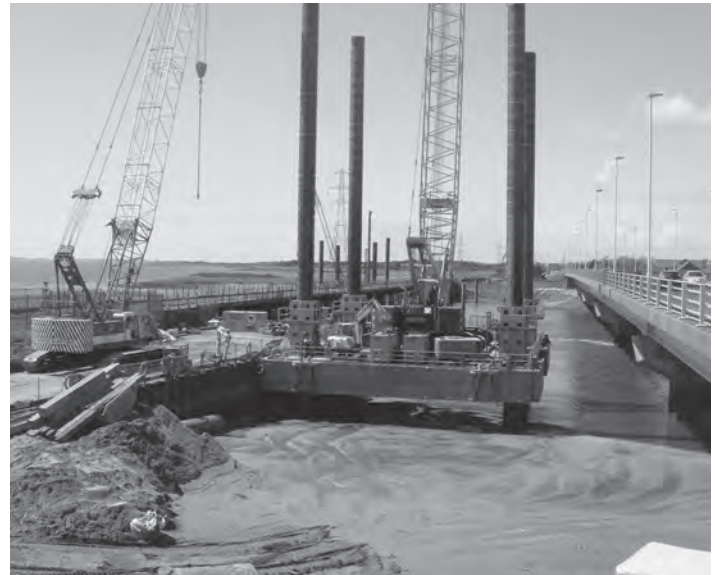
Figure 19.44 Floating piling plant (courtesy of Tony Gee)
