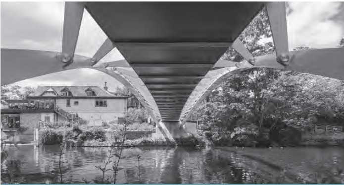
Figure 17.15 Underside of the deck, showing transverse stiffeners (© Lance McNulty)
