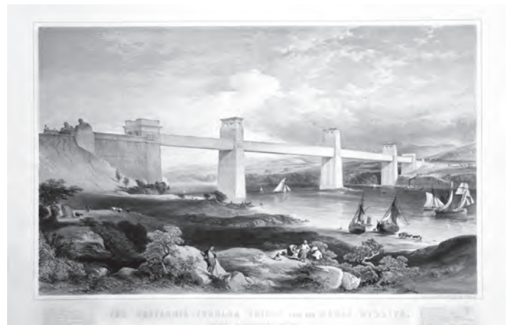
Figure 1.10 Britannia Bridge, Anglesey
