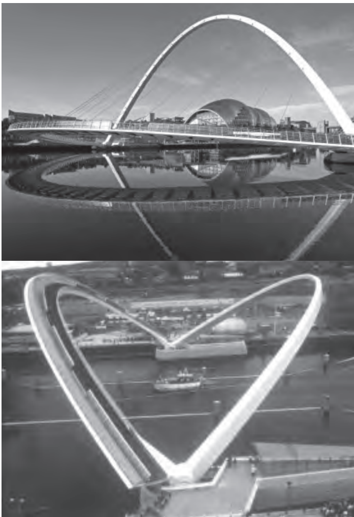
Figure 17.10 Gateshead Millennium Bridge – tilt bridge, Wilkinson Eyre/Gifford (copyright Graeme Peacock)
