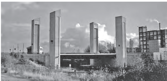
Figure 16.13 Centenary Bridge, Manchester, UK (photograph courtesy of C Birnstiel)
