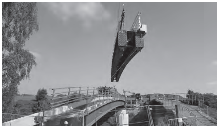
Figure 19.21 Placing twinned steel beams with precast kerb, Carters Bridge (courtesy of John Murphy and Sons)
