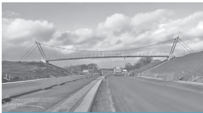
Figure 18.11 The Wilcott footbridge, Shropshire, UK, constructed from COMPOSOLITE (Strongwell, USA), a patented Maunsell plank (courtesy of Faber Maunsell)
