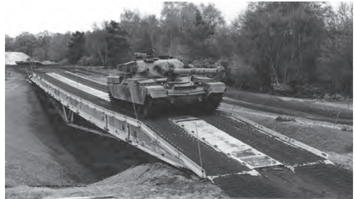
Figure 12.11 56t Chieftain tank crossing a 56m link reinforced aluminium alloy military bridge
