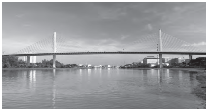
Figure 14.5 Sungai Prai Bridge, Malaysia. (Courtesy of Concessionaire, LLB)
