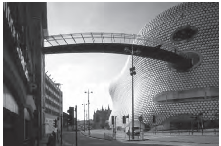
Figure 17.22 Sky bridge connecting Selfridges to multi-storey car park (photograph courtesy of Arup)
