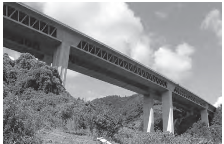
Figure 11.10 Precast slab on a composite truss bridge
