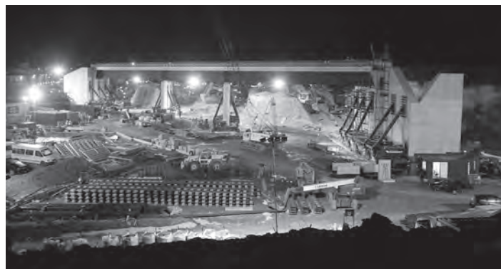
Figure 19.23 Channel Tunnel Rail Link 342: multispan viaduct with piers and abutments slid into position during a rail possession using slide tracks and hydraulic jacks (courtesy of VINCI)
