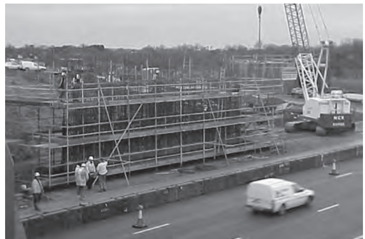
Figure 19.6 Bridge abutment constructed with access from traditional scaffolding system (courtesy of Norwest Holst)
