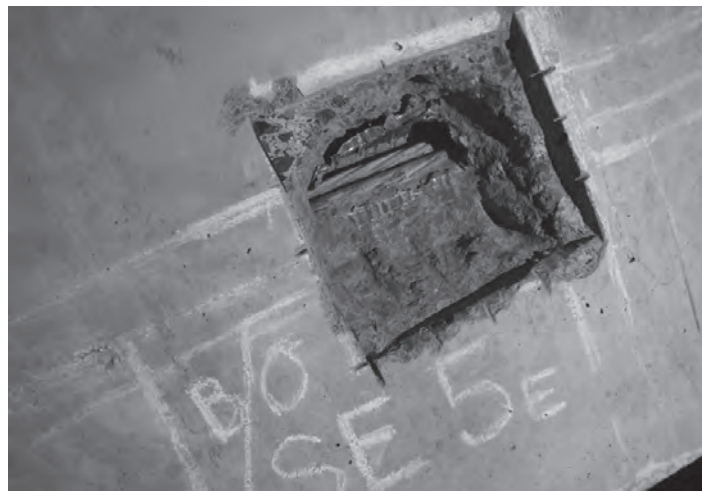
Figure 25.7 Post tensioned tendon investigations
