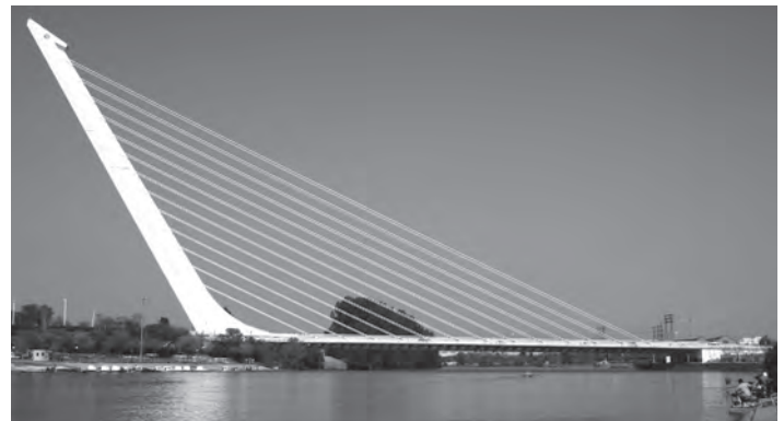
Figure 2.9 Visual clarity and meaning: Puente del Alamillo, Seville, Spain, noting technical ramifications of omitting back stays (image: https://commons.wikimedia.org/wiki/File:Puente_del_Alamillo_en_Sevilla.jpg )
