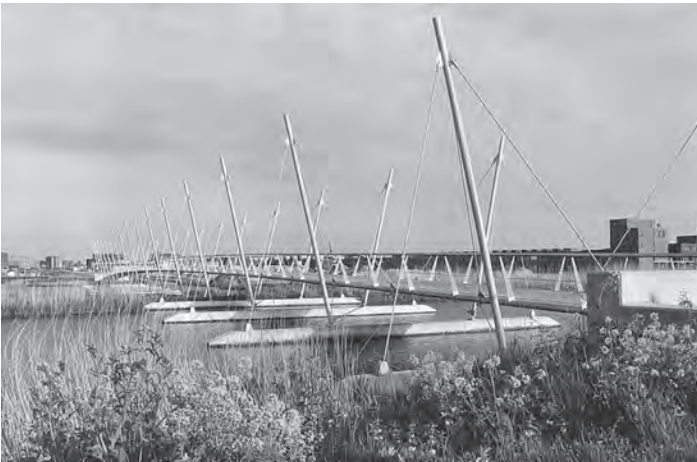
Figure 12.9 Stokkenbrug (courtesy of Bayards Aluminium Constructions BV, the Netherlands)
