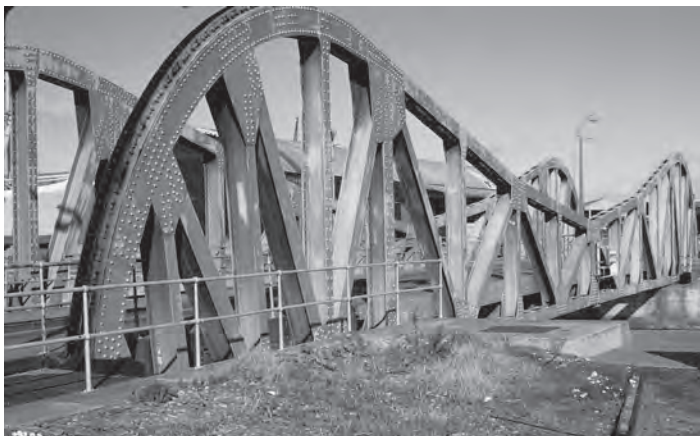
Figure 12.6 Hendon Dock Junction Bridge in Sunderland (courtesy of the Stafford Linsley collection)
