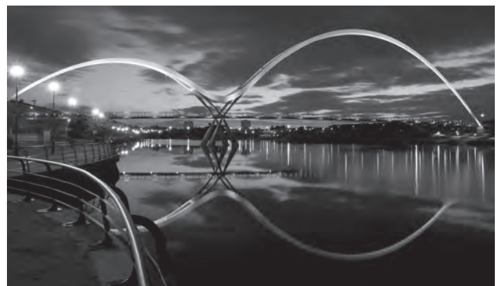
Figure 2.12 Infinity Bridge, Stockton ( https://commons.wikimedia.org/wiki/File:Night_Light.jpg )
