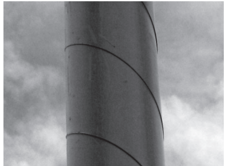
Figure 14.14 Outer sheath for parallel strand stay with helical ribs (courtesy of Nigel Hewson)
