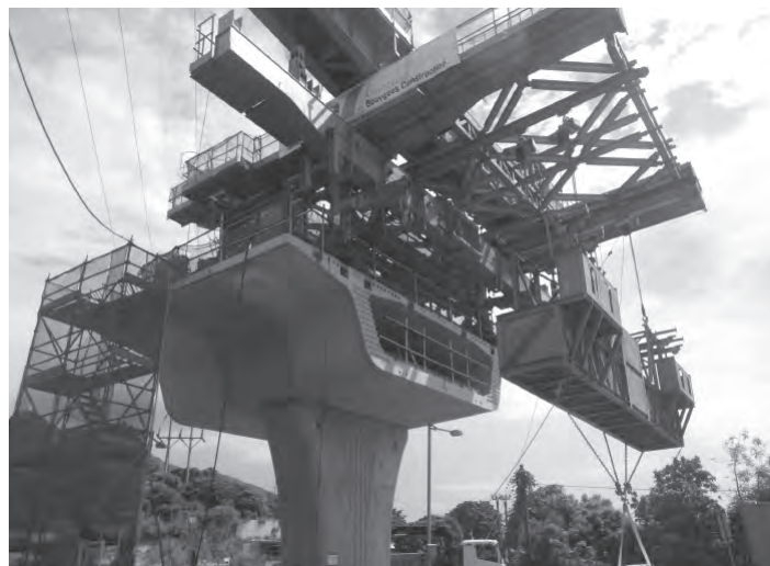
Figure 9.24 Precast segmental erection by lifting frame
