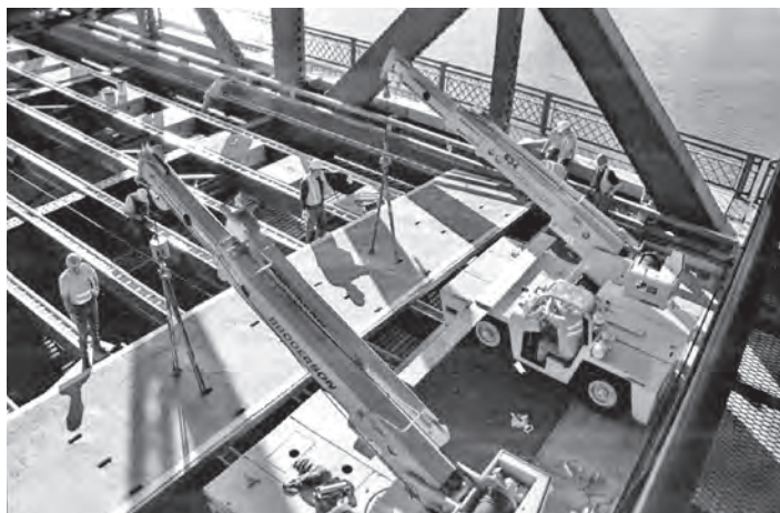
Figure 26.7 Replacement of steel grating deck with lightweight durable FRP deck on steel bascule bridge (photograph courtesy of Martin Marietta)
