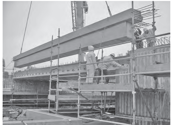
Figure 9.12 Crane erection of precast beams
