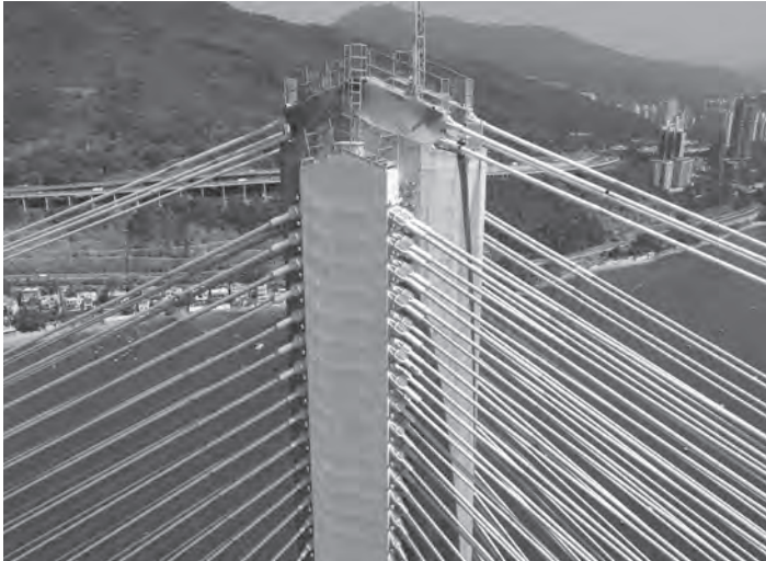
Figure 14.26 Fabricated anchor modules, Ting Kau Bridge, Hong Kong (contains photographs and information with the permission of the Highways Department of the Government of the Hong Kong Special Administrative Region; all rights reserved)
