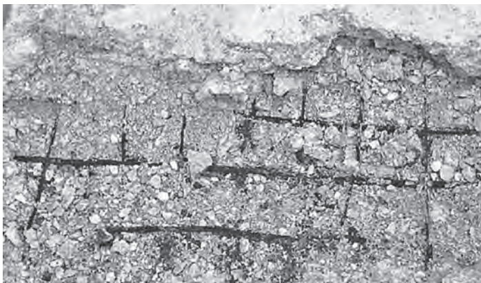
Figure 24.9 Corrosion in reinforcement tendon (photograph courtesy of LCPC)
