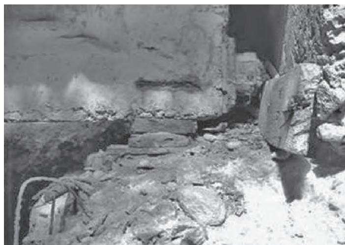
Figure 20.17 Lack of provision for jacking (reproduced with permission © the Highways Agency)
