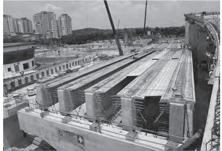
Figure 9.6 Beam-and-slab deck under construction
