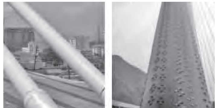
Figure 5.12 Surface finishes on stay cables: (a) ribbed HDPE ducting; (b) roughened HDPE ducting
