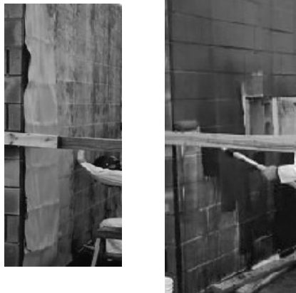
FIGURE 10.10: Kevlar® Wrap Retrofit to CMU Panel
