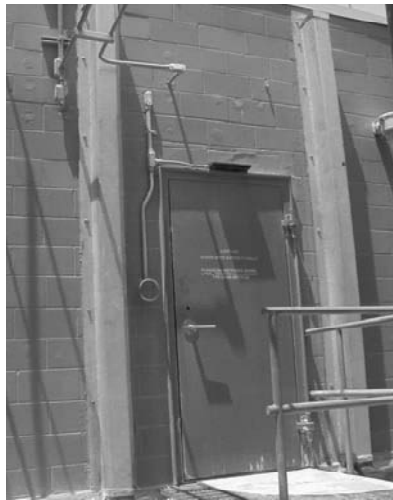
FIGURE 10.6: Masonry Wall Retrofit with Vertical Steel Posts
