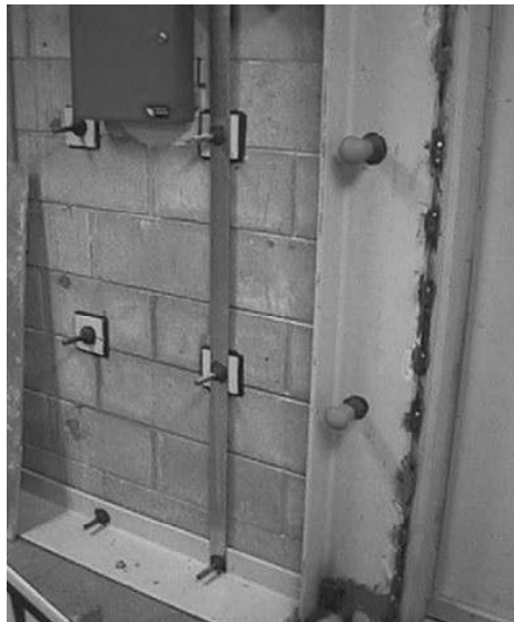
FIGURE 10.9: Through-Bolts on Inside Surface of Retrofitted Wall
