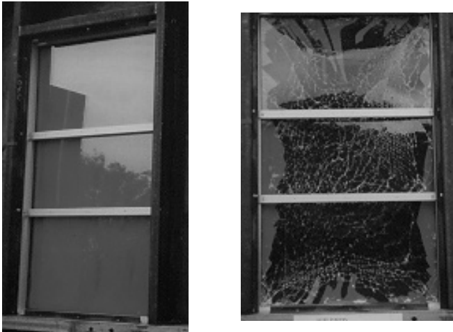
FIGURE 10.19: Window Retrofit Using Mullions and Film
