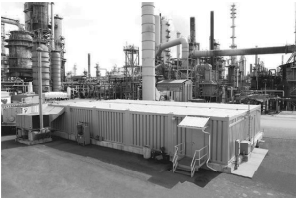
FIGURE 4.6: One-Story, Five Module Complex
