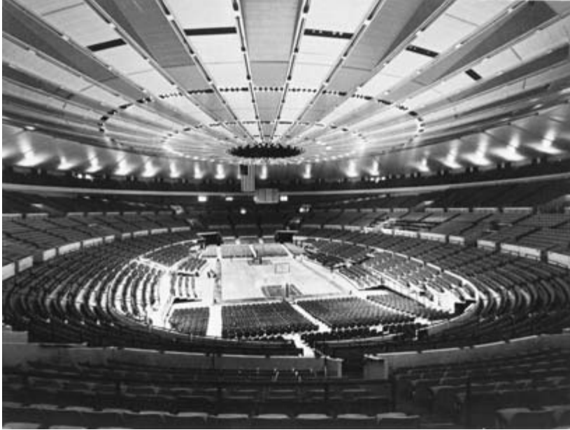
Our construction division's first project for an outside firm, Madison Square Garden.
