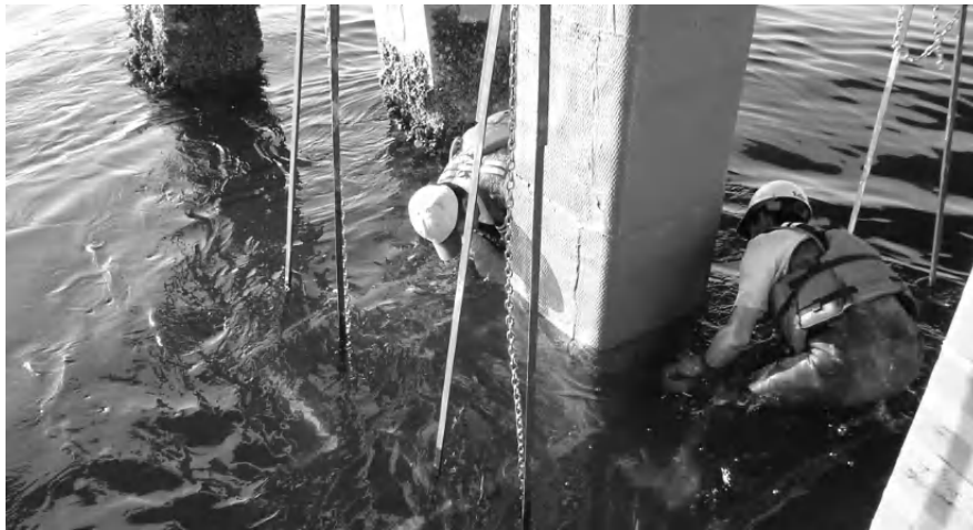
Figure 23.19. Underwater bonding of a glass fiber fabric (source: IIFC)
