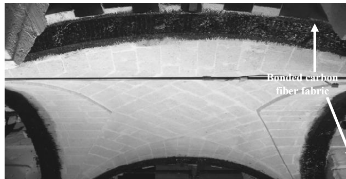
Figure 23.1. Strengthening of a masonry arch by externally bonded carbon fiber fabric (source: IIFC)
