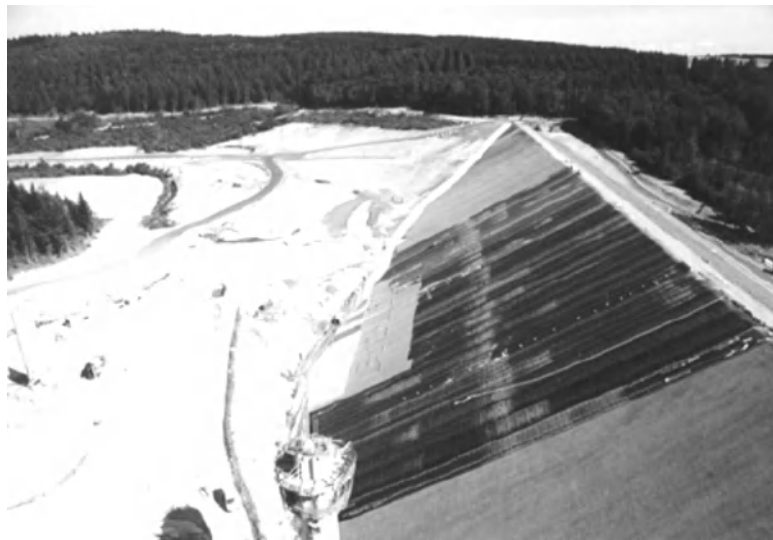
Figure 10.1. Geomembrane-lined dam (40 m high geomembrane for La Galaube dam over the river Alzeau, France) [GAU 02]
