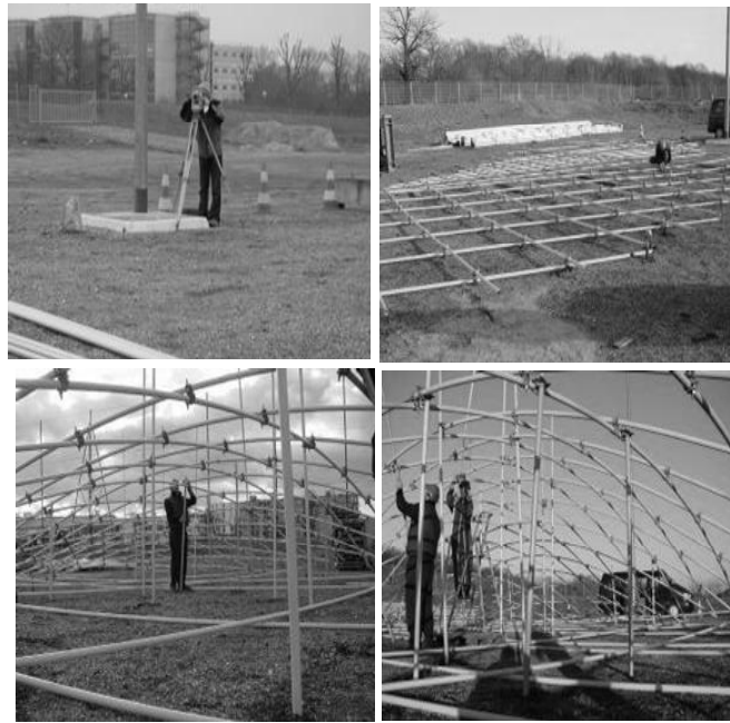
Figure 13.5. Assembly stage of a composite gridshell (ENPC)
