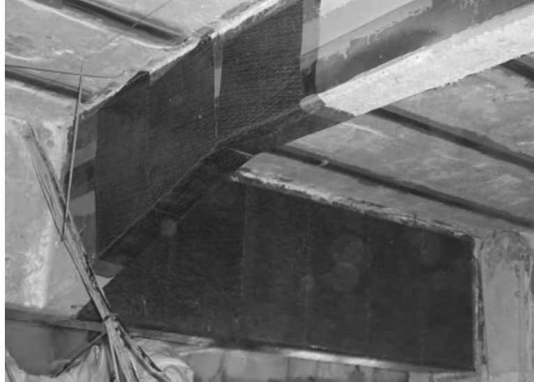
Figure 23.12. Example of a shear strengthening of a beam by bonded U-jacketed FRP (VSL-France)
