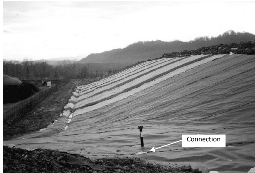
Figure 10.24. Example of waterproofing implementation on protective geotextile/drainage bands and connection the biogas collection network (waste storage site from Lescar [JAR 06])
