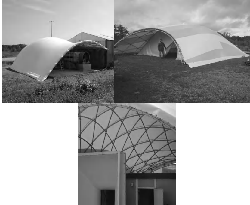
Figure 13.6. GFRP gridshell/coated polyester (ENPC)
