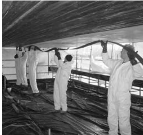
Figure 23.9. On-site girder strengthening by externally bonded FRP plate (source: Sika)
