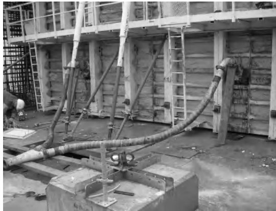
Figure 20.2. Vertical application. Concreting from the bottom
