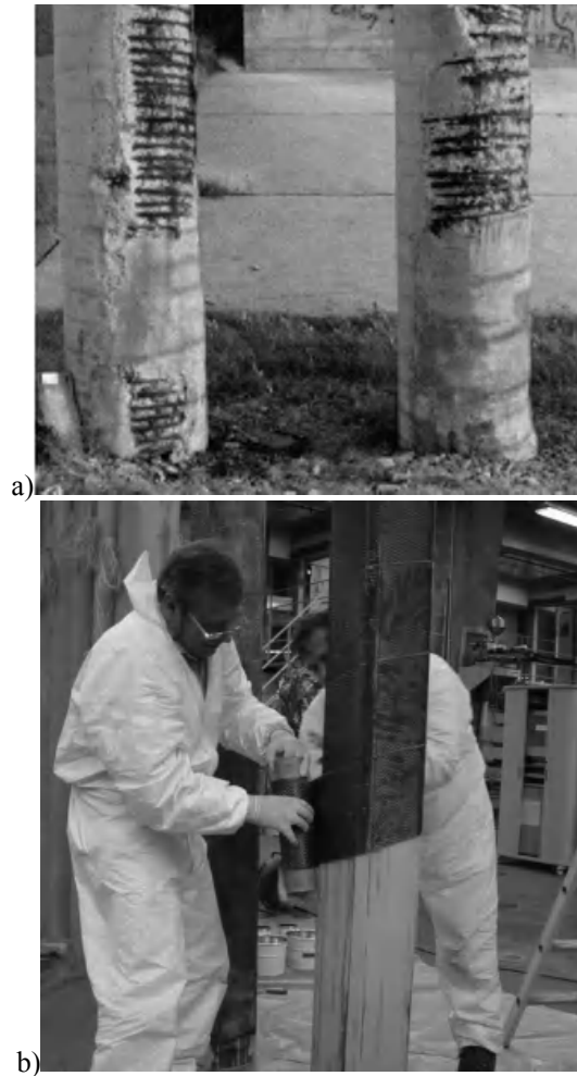
Figure 23.13. Rehabilitation of columns by wrapping: a) example of severely deteriorated column, (source: ISIS-Canada); b) application of FRP sheets using the wet lay-up technique, (source: LCPC)
