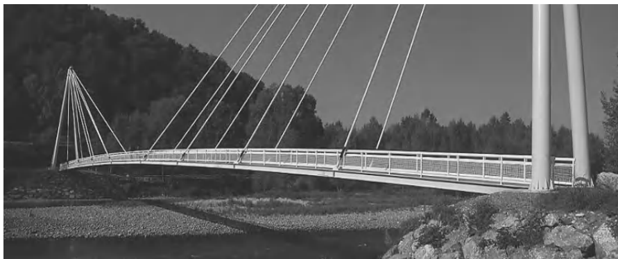
Figure 13.1. Laroin Footbridge (Freyssinet Photo Library)
