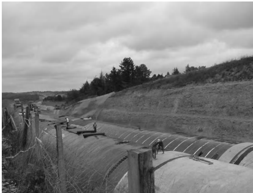
Figure 10.2. Cut-and-cover tunnel at Constans, and waterproofing device (cover) on an underground structure (photo taken from SEMALY, [MAH 06])
