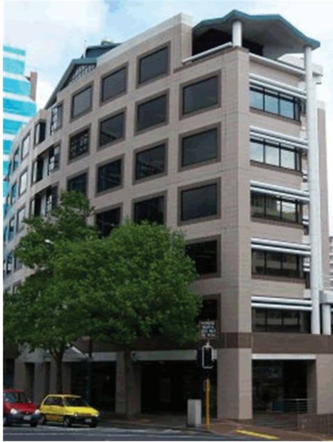
FIGURE 7.1 External view of Environment A.
