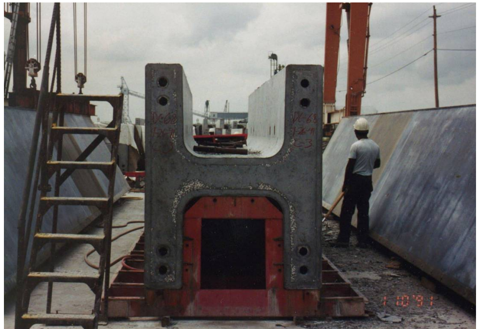
Figure 5.3.1.1-1 Precast Open Frame Pier Bent Top Photo: Overall Bridge Bottom Photo: Casting of Columns (source: Splice Sleeve North America Inc.)
