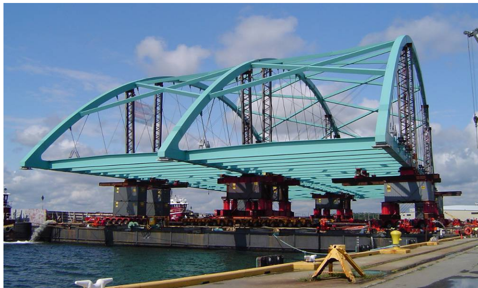
Figure 2.4.1-3 SPMT Bridge Move in Rhode Island
