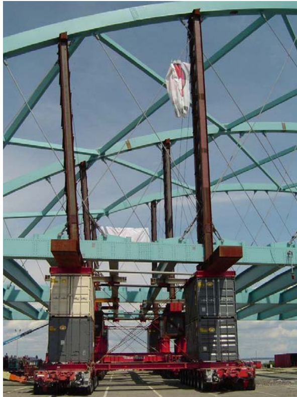
Figure 7.1.1-1 Shipping Containers Used for Shoring
