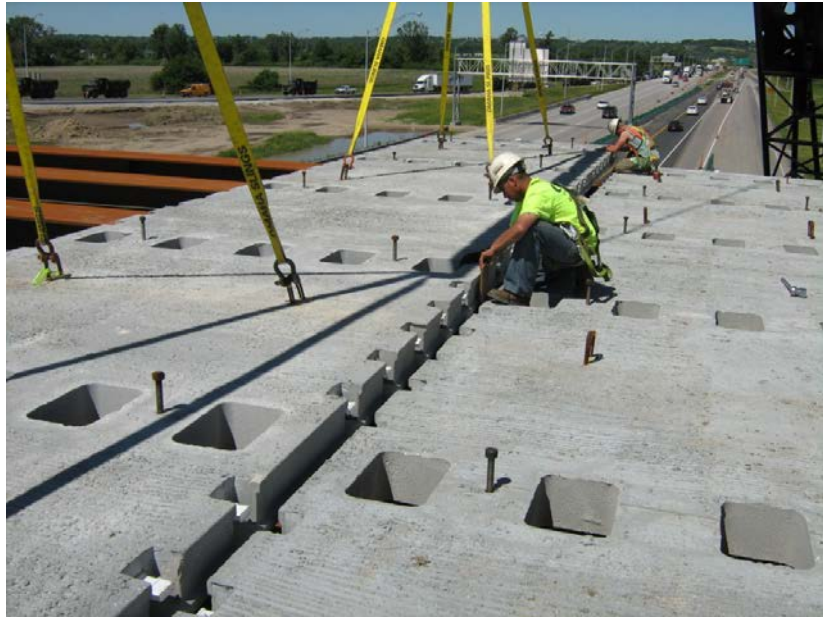
Figure 5.2.3.1-1 Precast Full Depth Deck Installation
