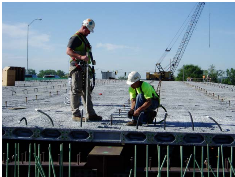
Figure 5.2.3.1-2 Precast Full Depth Deck Leveling System
