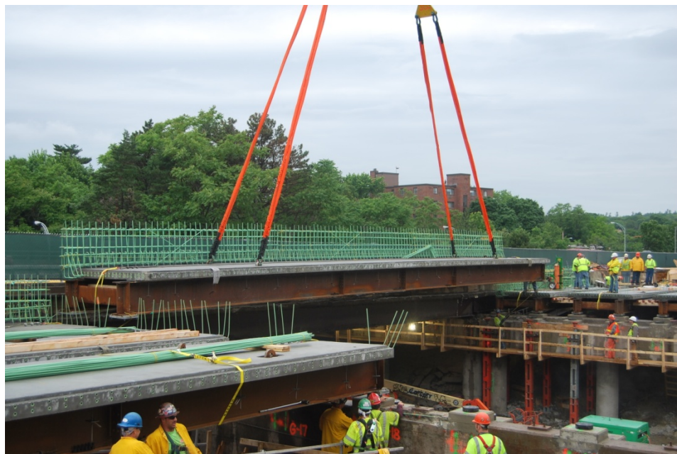
Figure 2.3.1-5 I-93 Superstructure Replacement Construction
