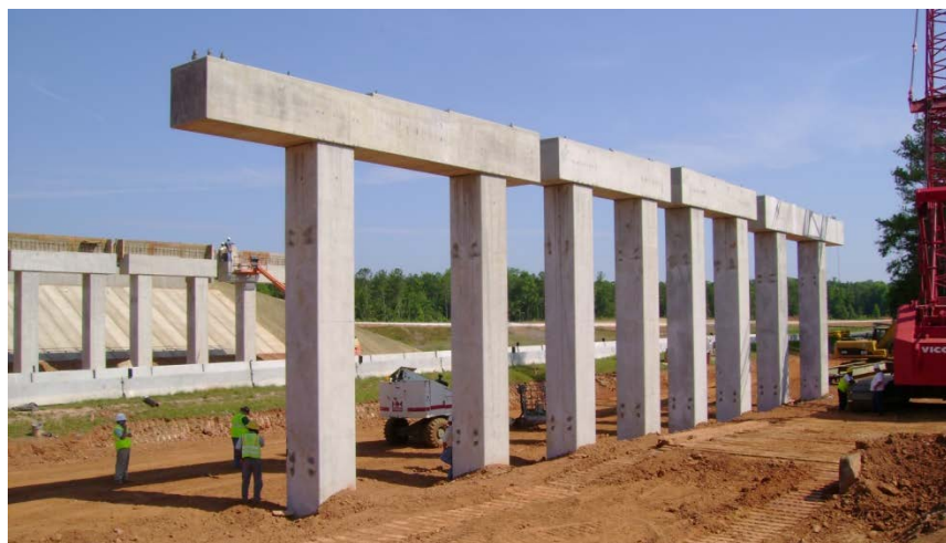
Figure 5.3.1.1-3 Precast Open Frame Pier Bent
