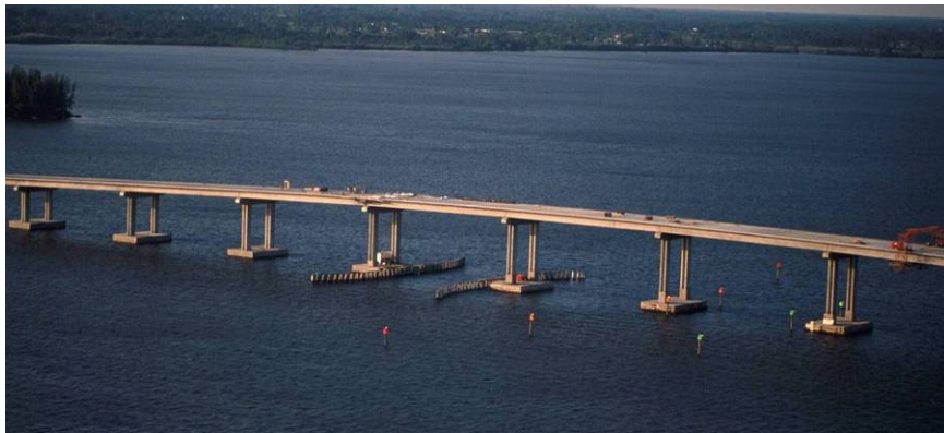
Figure 8.2.1.1-1 Edison Bridge Top Photo: During Construction Bottom Photo: Just Prior to Opening (source: Splice Sleeve North America Inc.)
