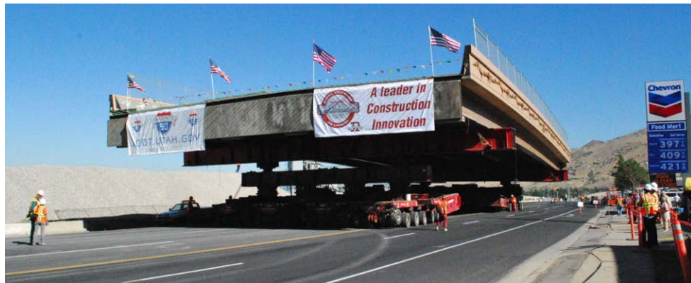
Figure 2.4.1-2 SPMT Bridge Moves in Utah
