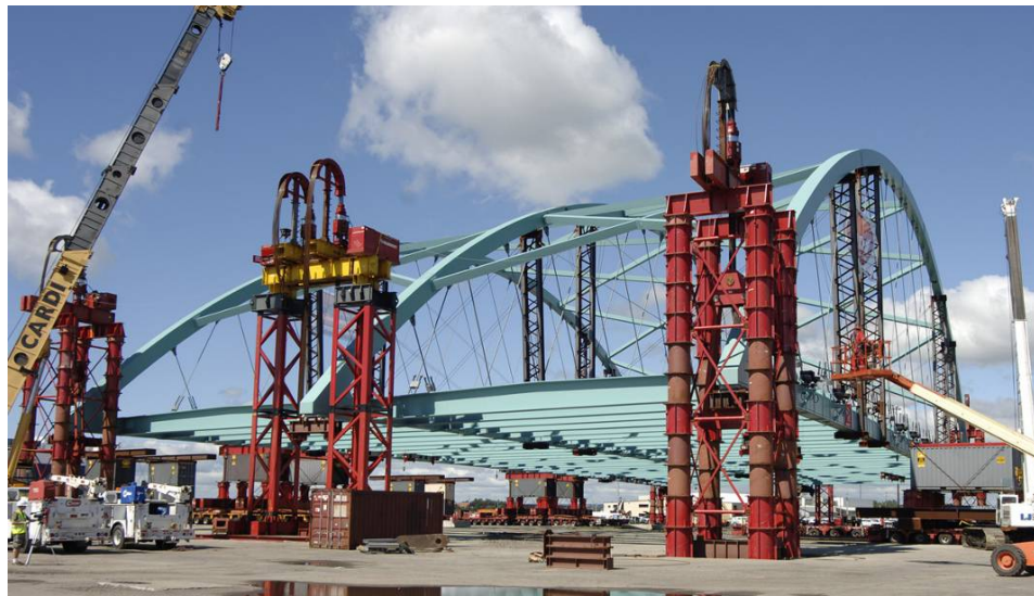
Figure 2.4.4-1 Strand Jack Lifting of the Providence River Bridge (source: Mammoet)
