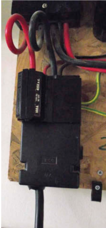
Figure 5.8 TN-C-S service head
