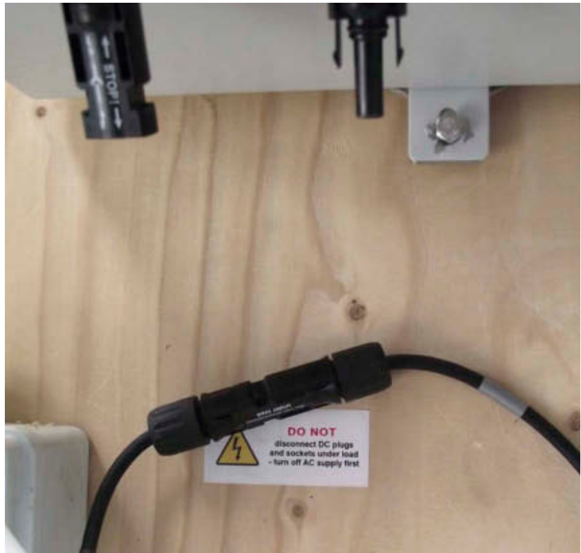
Figure 10.9 D.C. leads joined
