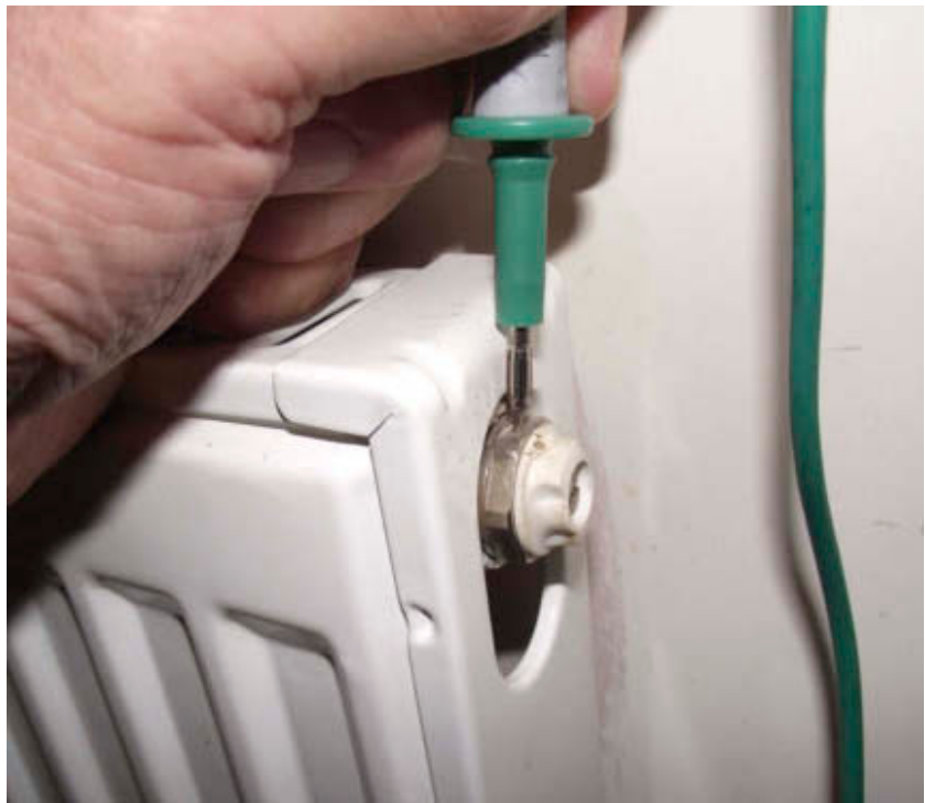
Figure 4.22 Lead on unpainted part of radiator
