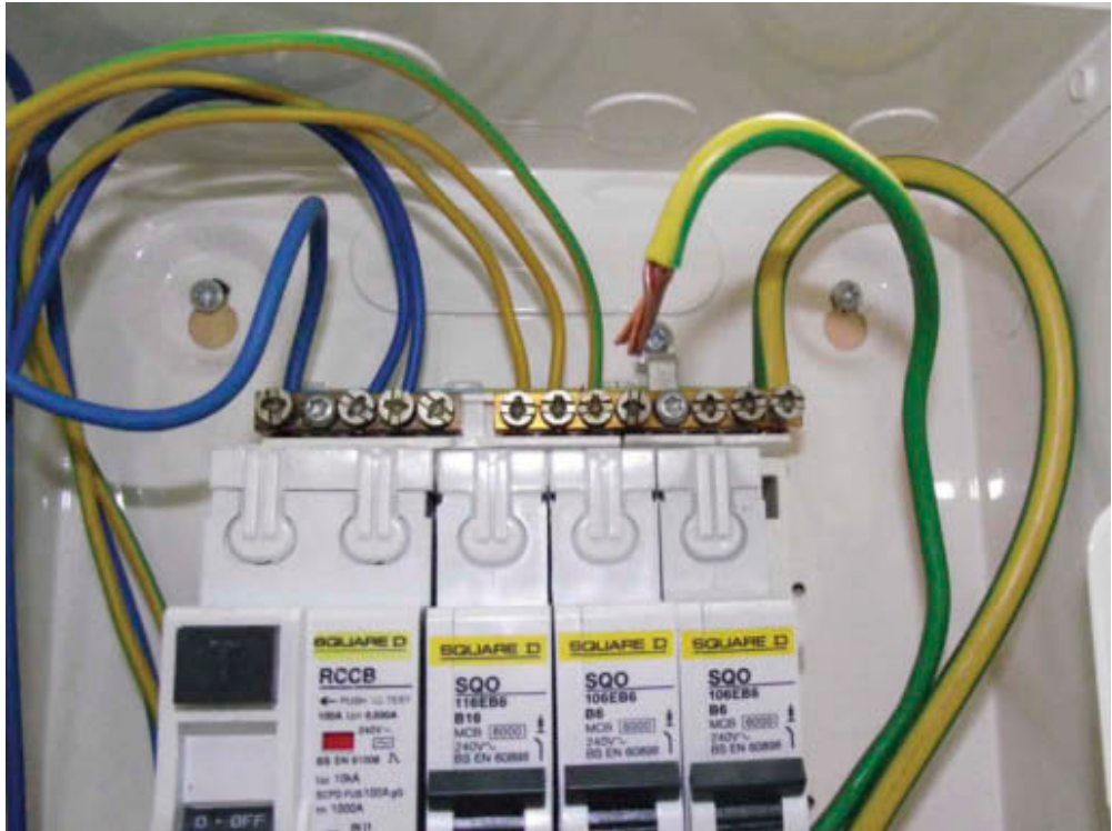
Figure 4.13 Bonding disconnected
