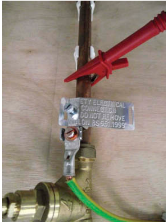
Figure 4.16 Second lead connected
