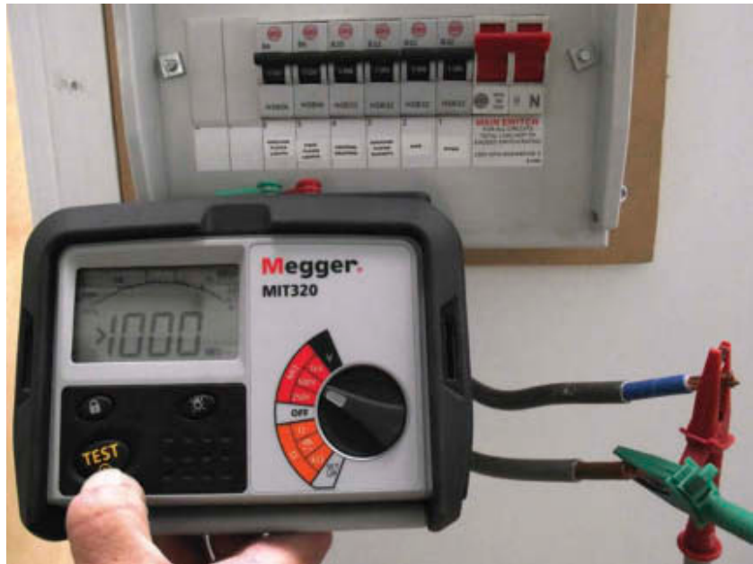
Figure 4.46 Test between live conductors
