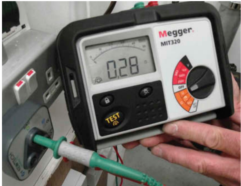
Figure 4.39 Test line to earth at each socket
