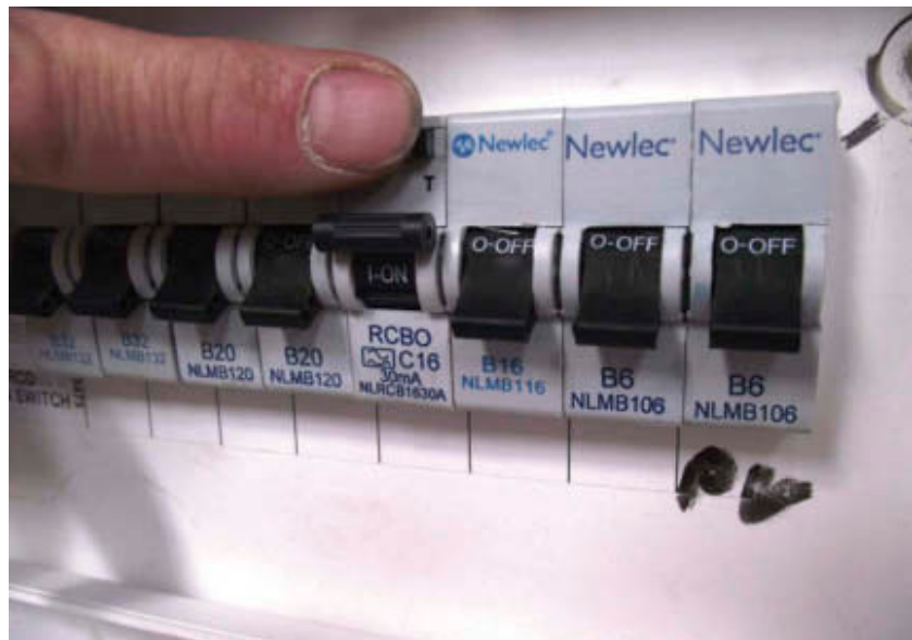
Figure 5.45 Manual test
