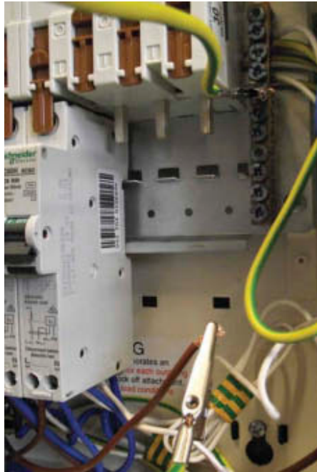
Figure 4.61 Line and earth terminal linked
