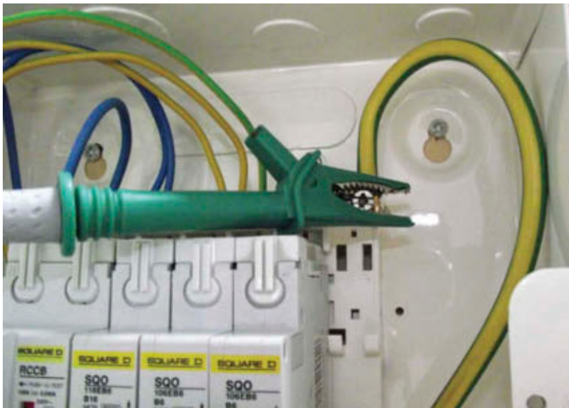
Figure 4.27 Lead connected to earthing terminal
