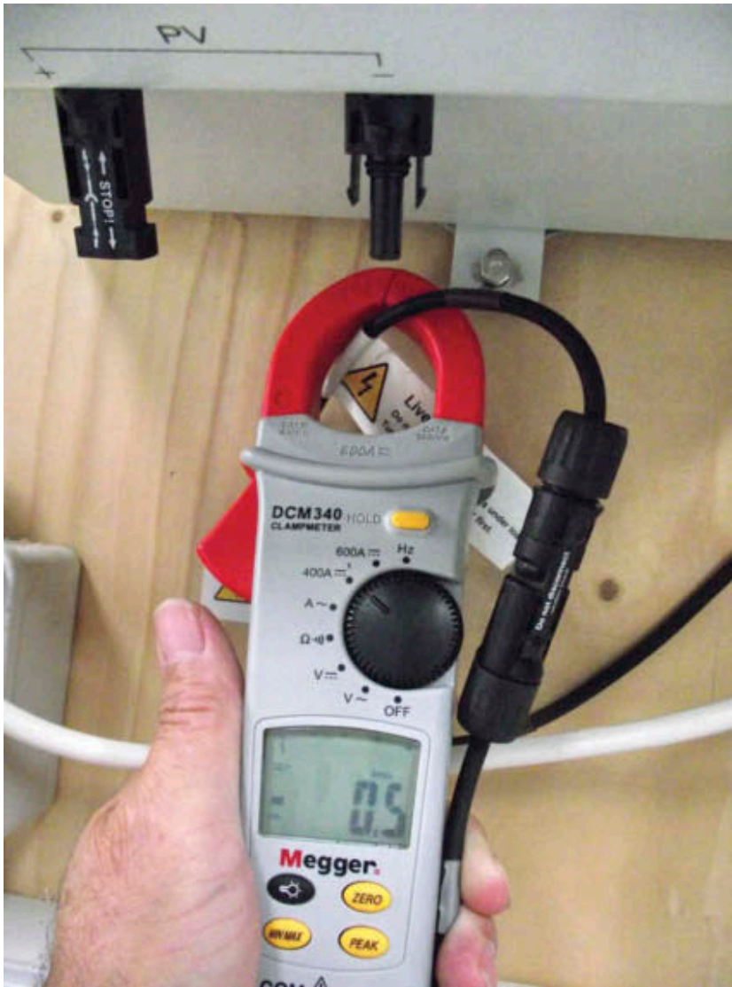
Figure 10.10 Current measurement using clamp meter
