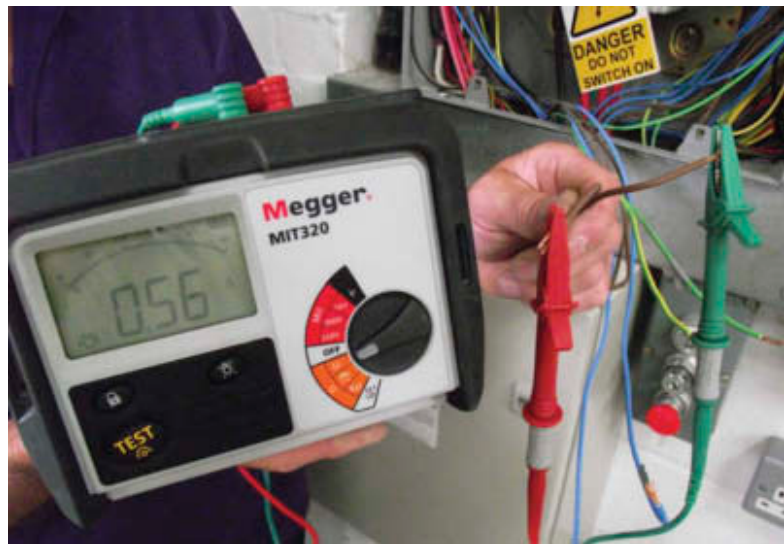
Figure 4.33 Test each end of the line conductor
