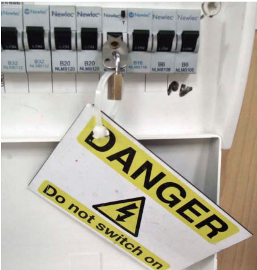
Figure 4.8 Locked off
