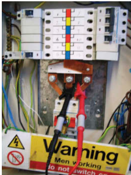
Figure 4.51a Test L2 to L3
