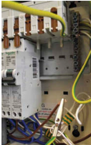
Figure 4.57 Line linked to earth terminal
