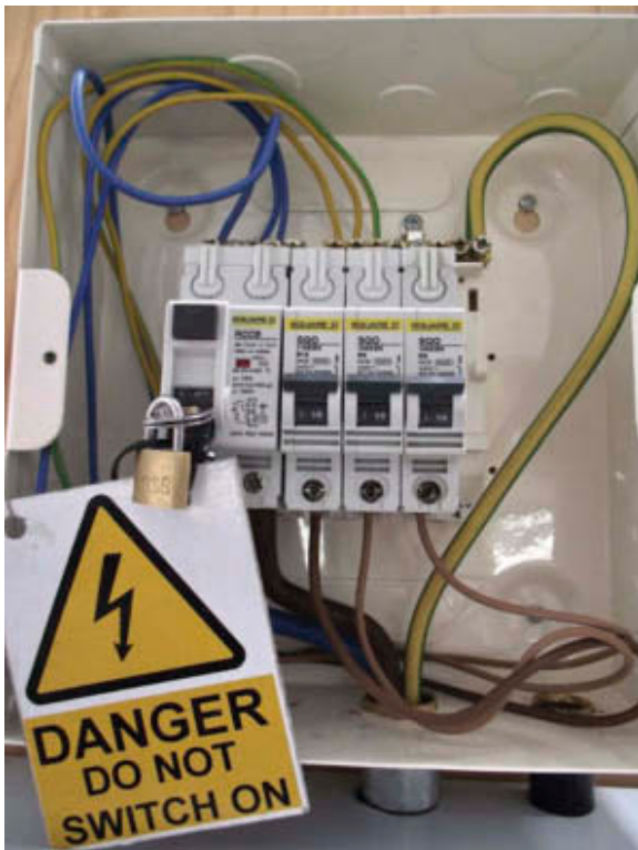
Figure 4.12 Isolate the supply
