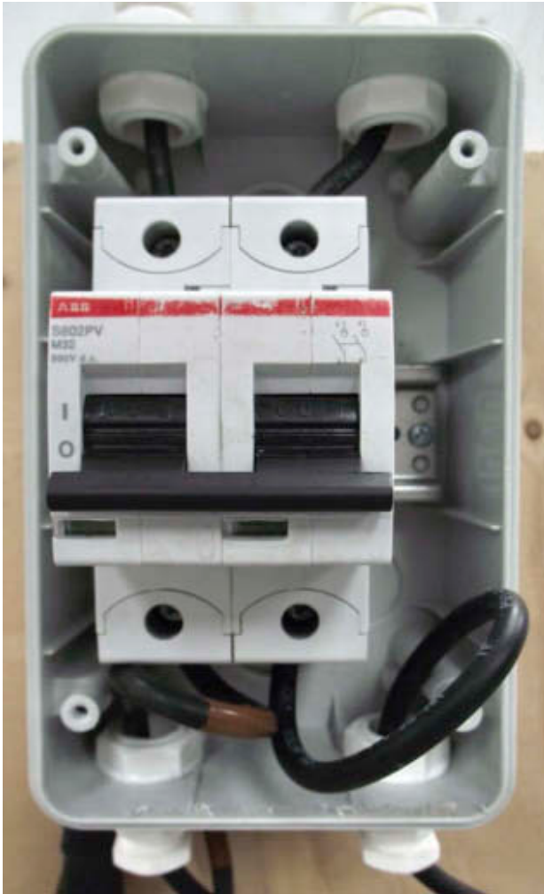
Figure 10.12 D.C. isolated
