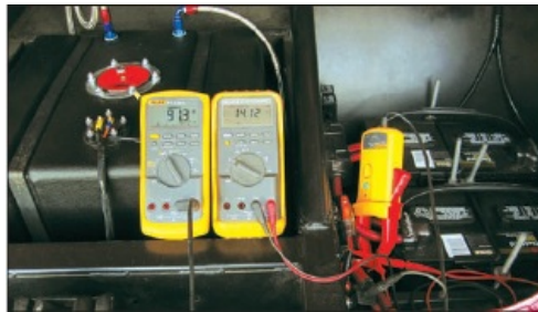
Fig. 2.20. You can quickly and easily determine the health of your charging system with two DMMs and a Hall effect DC ammeter accessory, such as the Fluke i410.
