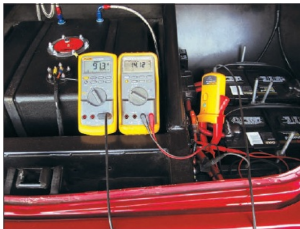
Fig. 4.19. 12-Volt Batteries—With all accessories on and the engine at operating temperature and at idle, I measured 91.3 amps at 14.12 volts. This is the sign of a healthy 12-volt charging system with a proper-size alternator.
