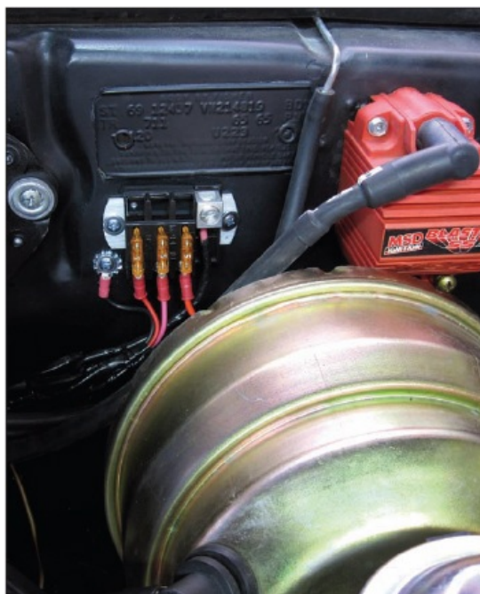
Fig. 2.36. I mounted a small fuse panel behind the brake booster. This supplies switched power to the ignition box, tach adapter, and the switched side of the coil for the fuel pump relay.
