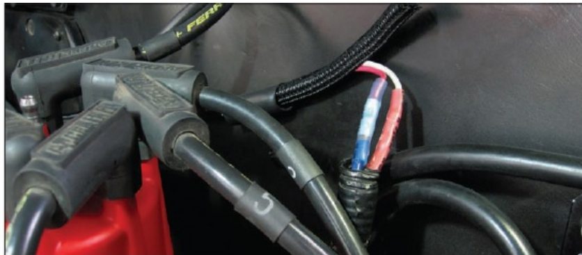
Fig. 5.58. I made these connections with heat-shrinkable butt connectors, as they were both low current, and then slid the heat shrink (left) over the connections to insulate them. Yes, I realize that the number-3 plug wire is in the wrong location. Keith swapped it with number-6 and all was good.
