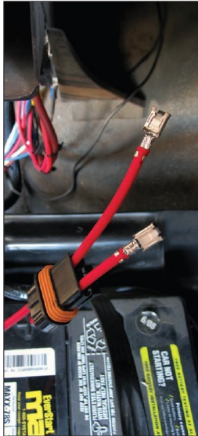
Fig. 6.45. I always crimp and solder all 10 AWG open-barrel terminals for maximum current transfer. After the wires cool, they can be snapped back into the housing.
