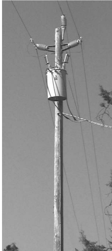
Figure 2.27 Delta distribution configuration.
