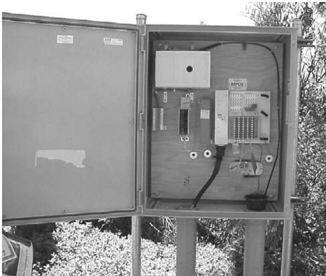
Figure 6.23 CFJ fiber—support structure. Courtesy of RLH Industries, Inc.
