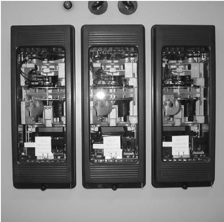
Figure 2.33 Electromechanical relays.
