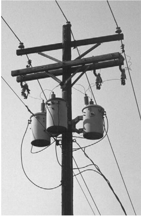
Figure 2.26 Wye distribution configuration.
