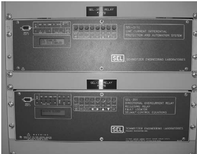
Figure 2.32 Solid-state relays.
