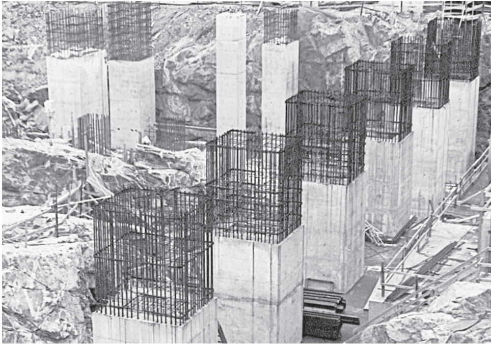
FIGURE 9-2 Foundation columns, turbine generator building, Seabrook Station, New Hampshire. (George Limbrunner)
