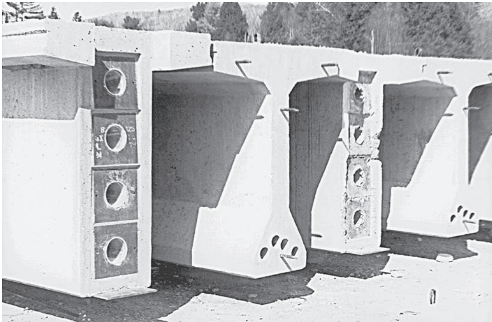
FIGURE 11-1 Precast bridge girder components for post-tensioning. (George Limbrunner)
