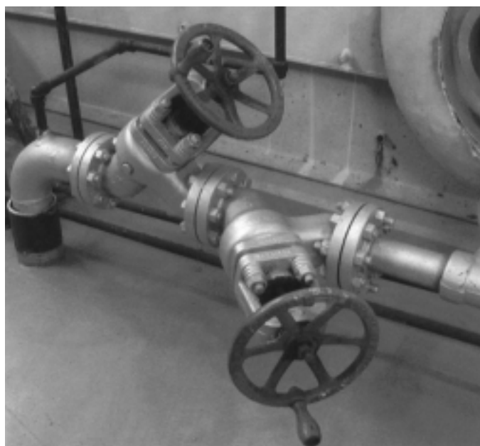
Figure 2-5. Seatless blowoff valves
