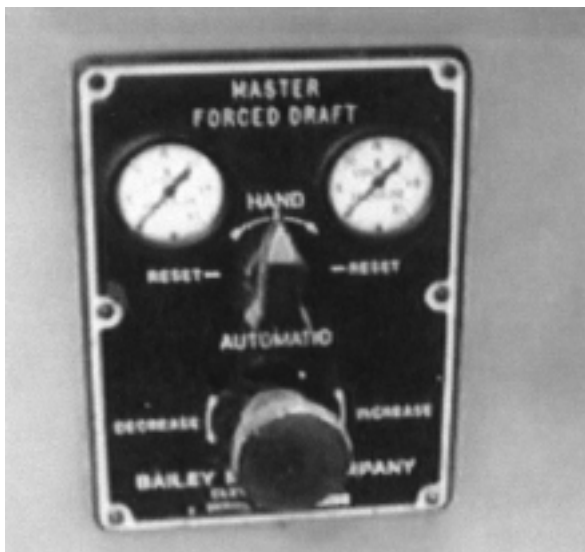
Figure 10-11. Early pneumatic H/A station
