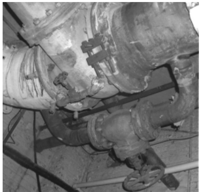
Figure 2-1. Warm-up bypass valves
