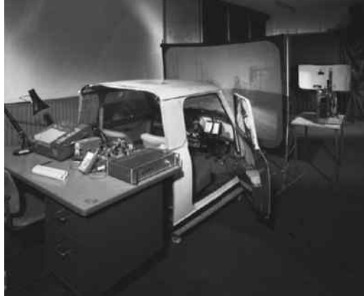
FIGURE 9.4 Early film-based simulator at TRL circa 1970.
