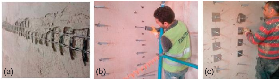
Figure 17.20 (a–c) Strengthening of a masonry wall in the historical building. Kind permission of Fyfe Europe SA.
