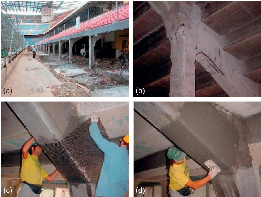
Figure 17.1 (a) Existing RC frame supporting the tier of seats; (b) typical damage found in RC beams; (c) application of a U-shaped TRM jacket for shear strengthening of the beam; and (d) strengthened beam at the end. Kind permission of Ruredil SPA.
