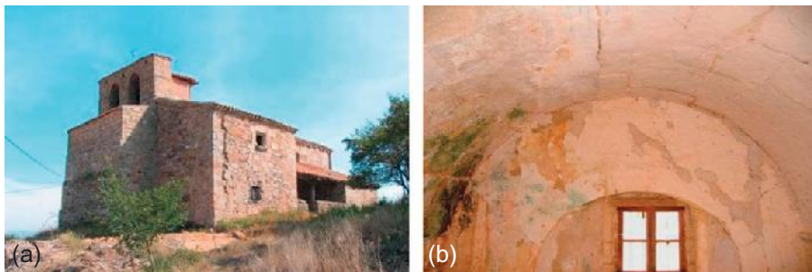
Figure 17.16 San Roque church earthquake damage: (a) wall out-of-plane separation and (b) critical cracks on the main vault. Kind permission of Fyfe Europe SA.
