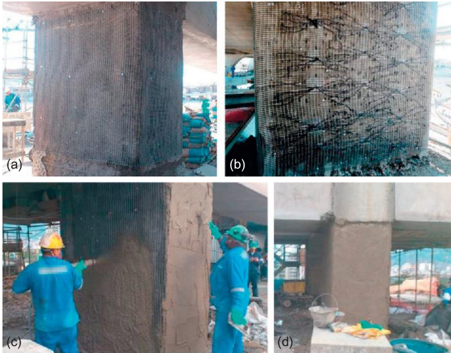
Figure 17.11 (a) Fastening of the carbon textile reinforcement; (b) FRP anchors in wall-like columns; (c) a building worker is spraying shotcrete on the fastened carbon reinforcement; and (d) strengthened column at the end.
