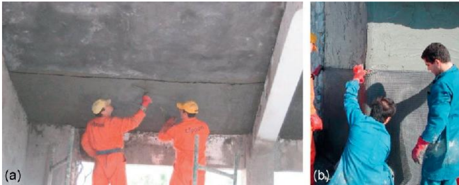
Figure 17.4 Strengthening of (a) concrete slabs and (b) stone masonry walls in a mixed concrete–masonry school building. Kind permission of Triantafillou (2007).
