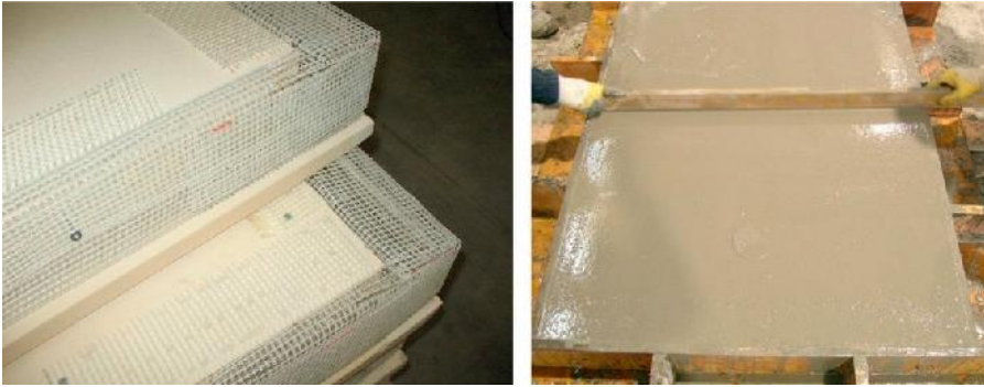
Figure 3.5 Reinforcement cage and cast sandwich element.
