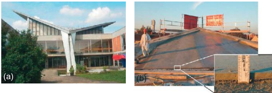
Figure 6.2 (a) Damaged steel-reinforced concrete hypar-shell at the FH Schweinfurt (Germany) and (b) strengthening with TRC (Weiland et al., 2008).
