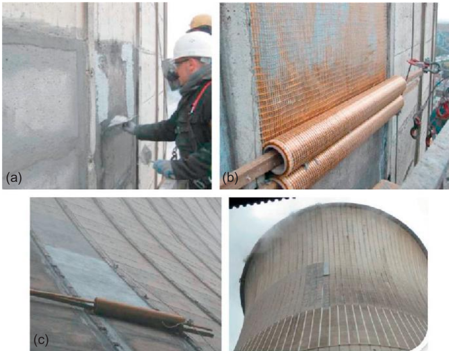
Figure 17.9 (a) Screeding of the inorganic matrix on the tower shells; (b) application of two layers of PBO textile reinforcement; and (c) overview of the strengthening application. Kind permission of Ruredil SPA.
