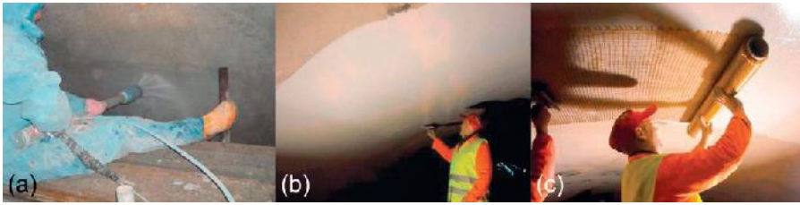
Figure 17.6 (a) Surface preparation by hydrojetting; (b) application of the inorganic matrix; and (c) application of the PBO textile reinforcement.
