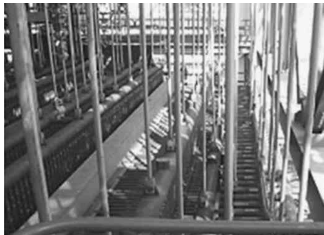
FIGURE 18.24 Sling rods at the top of the boiler.
