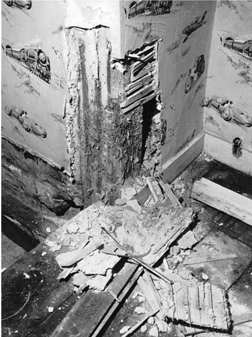
Figure 9.2 Effects of death watch beetle. Reproduced by permission of Harsco Infrastructure
