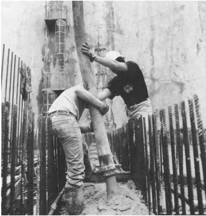
Plate 14a. The typical fluidity of pumped concrete; but it still needs vibrating in place
