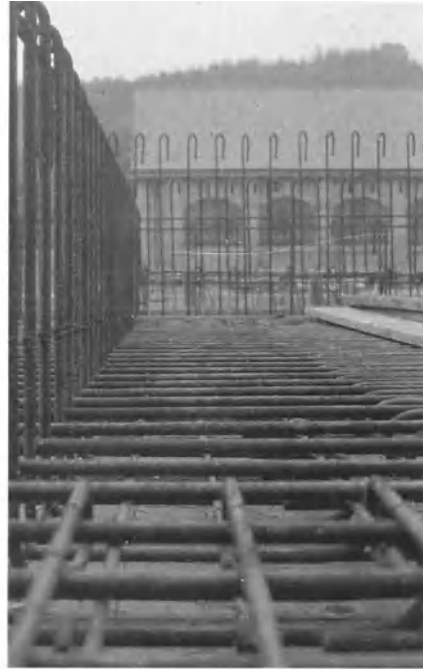
Plate 16b. Accurately placed reinforcement, strong enough to walk on
