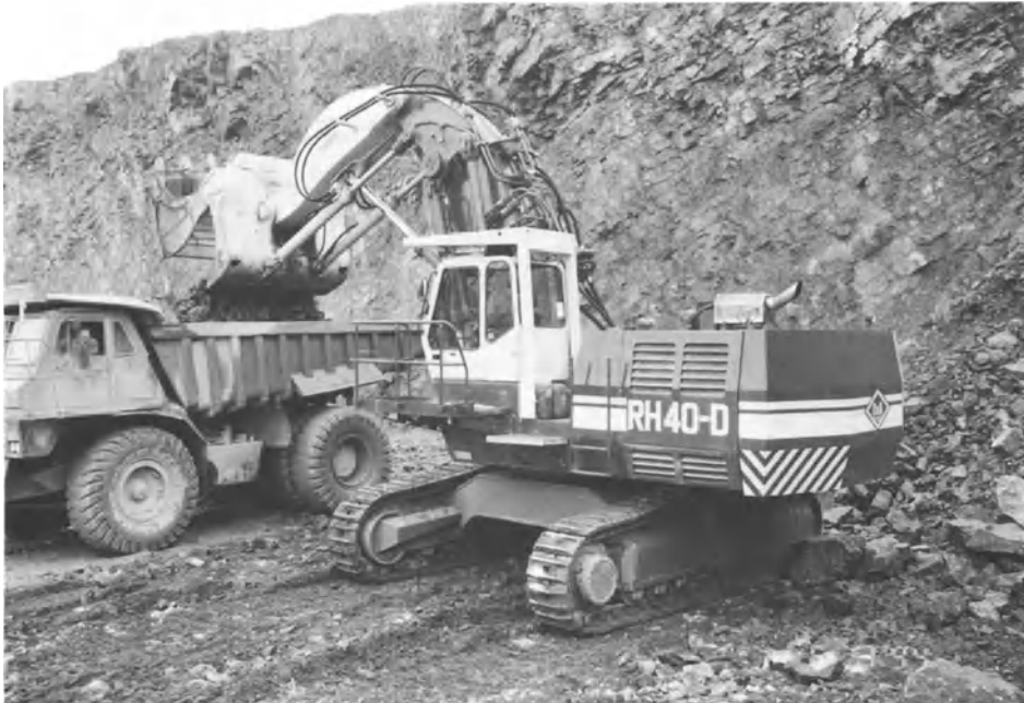
Plate 4a. An O & K RH40D 365 kW tracked excavator operating as a face shovel with 6 m 3 bucket. Orenstein & Koppel Ltd, Northampton, UK
