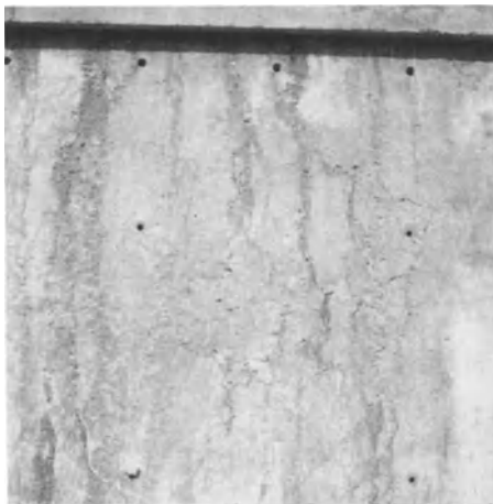
Plate 15b. Sand runs on a concrete surface. Photo on the right also shows lack of compaction probably due to a slight movement of formwork adjacent to the vertical joint
