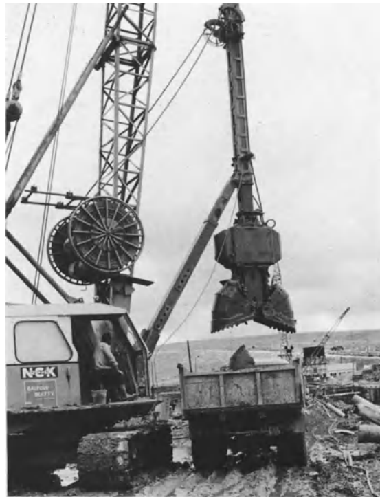
Plate 11b. Excavating grab for diaphragm walling construction
