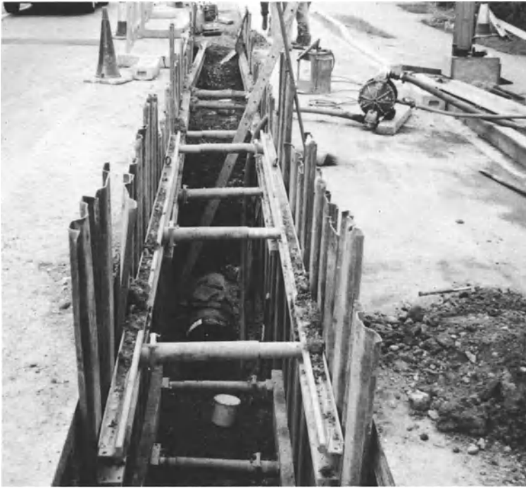
Plate 10a. A properly supported trench
