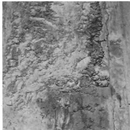
Plate 15b. Sand runs on a concrete surface. Photo on the right also shows lack of compaction probably due to a slight movement of formwork adjacent to the vertical joint
