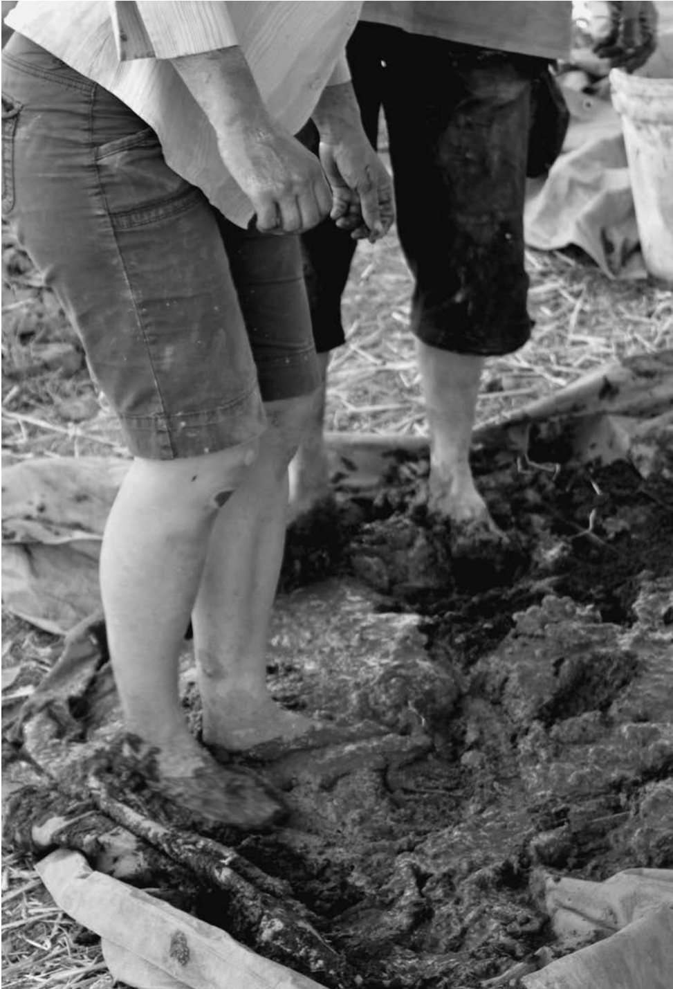
Figure 14.1 Mixing mud to make mudbricks
