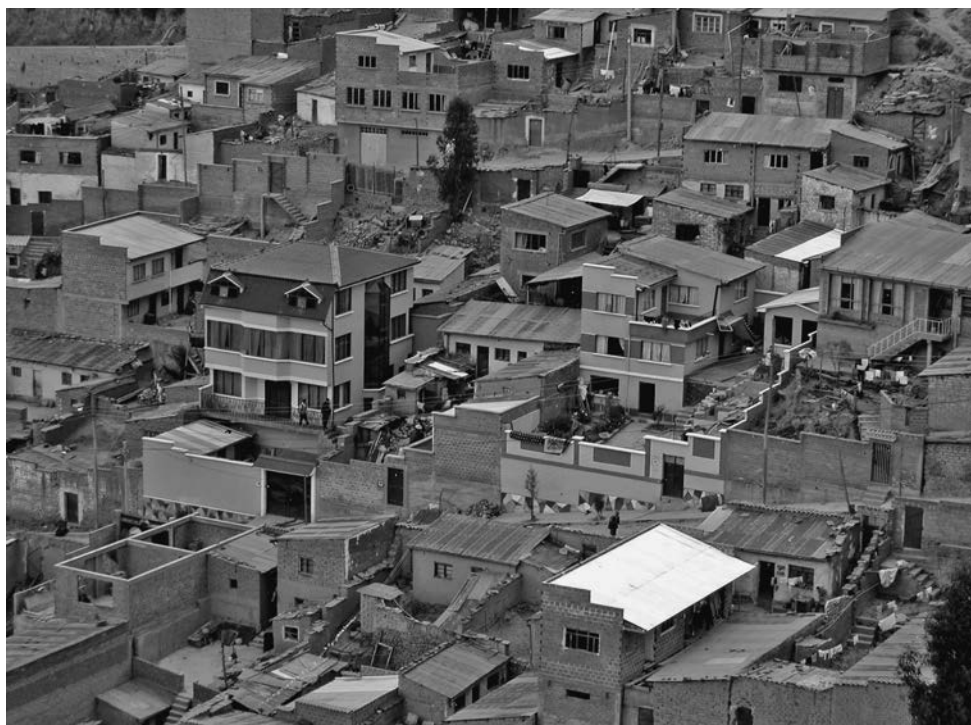
Figure 8.8 Different stages of construction
