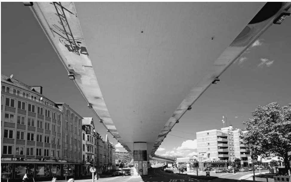
Figure 12.2 Elevated highway in Hagen (Ruhr district, Germany)
