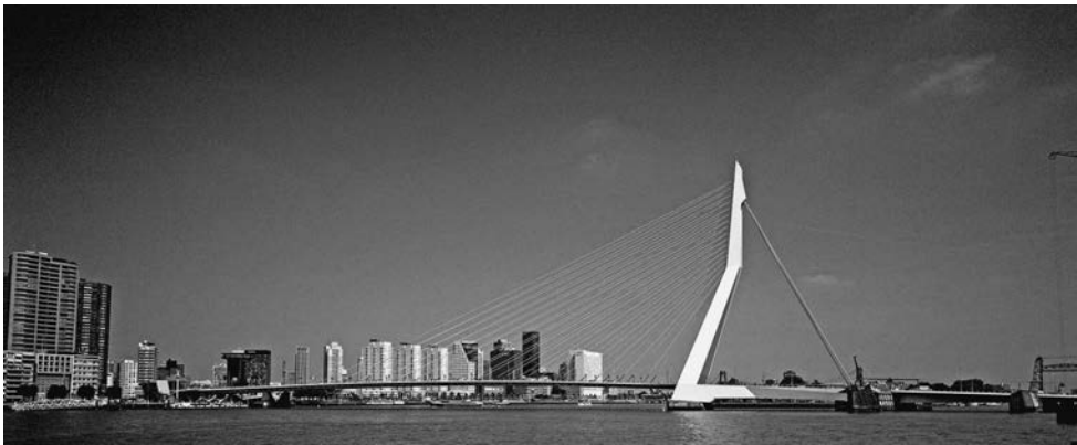
Figure 12.1 Erasmus Bridge in Rotterdam (Netherlands) by Architekten Van Berkel & Bos
