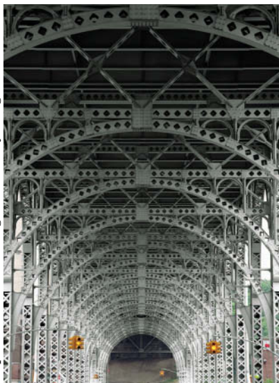
This New York City bridge structure suggests that members of a simple truss need not be straight.
