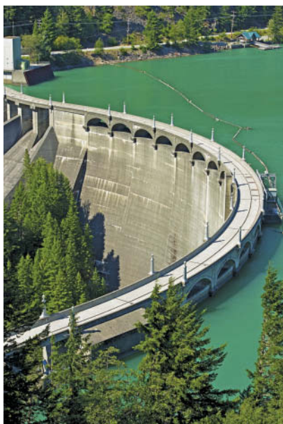
The Diablo Dam supplies electrical power to Seattle, Washington.
