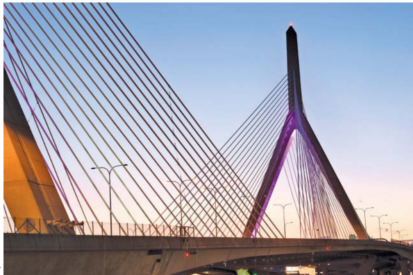
Another view of the Zakim Bunker Hill Bridge in Boston.
