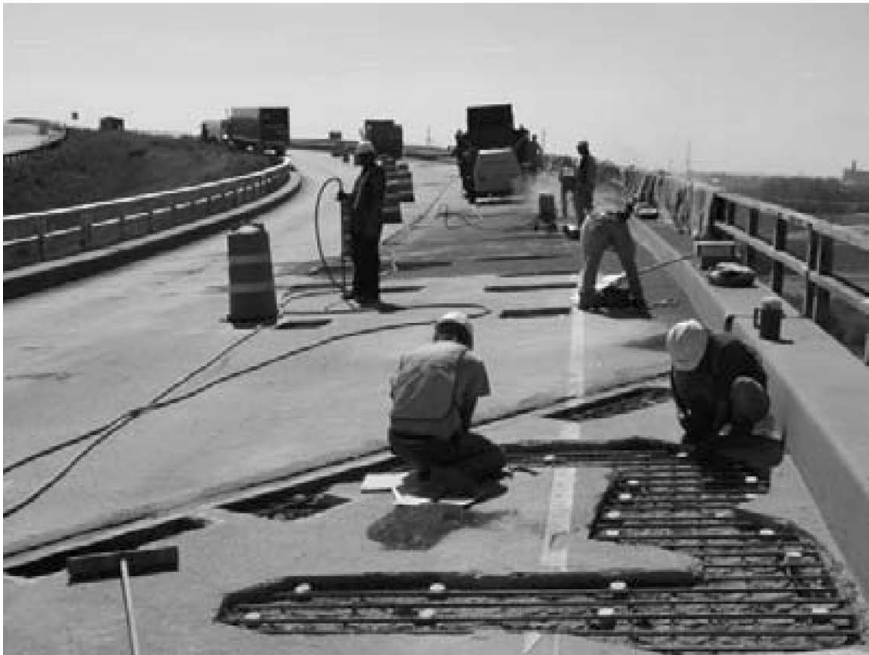
Figure 4.25 A sacrificial anode cathodic protection system, called Galvashield cathodic protection system was installed in SH 85 SB in Greeley, Colorado.
