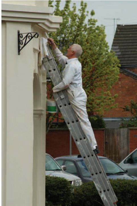
Figure 7.1 Painting contractor at work.
