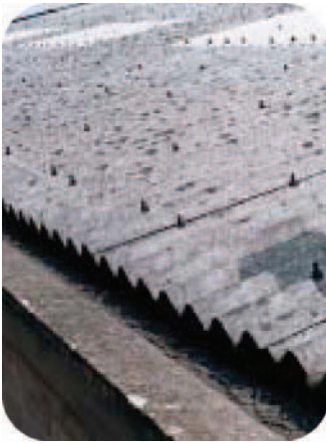
Asbestos cement roof
