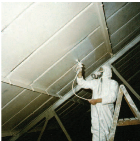
Figure 5.7 Asbestos removed and repainting.
