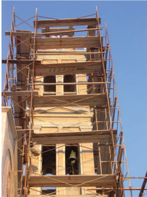
Figure 8.3 Poor scaffold.
