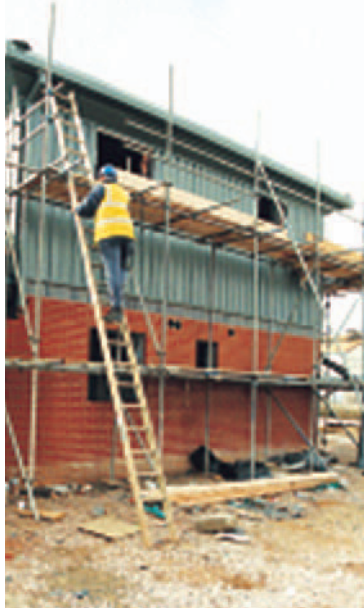
Pole ladder in use
