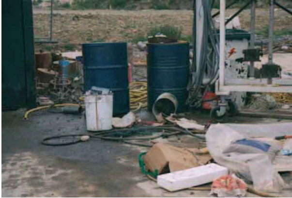
Figure 4.3 Poor housekeeping and waste collection.
