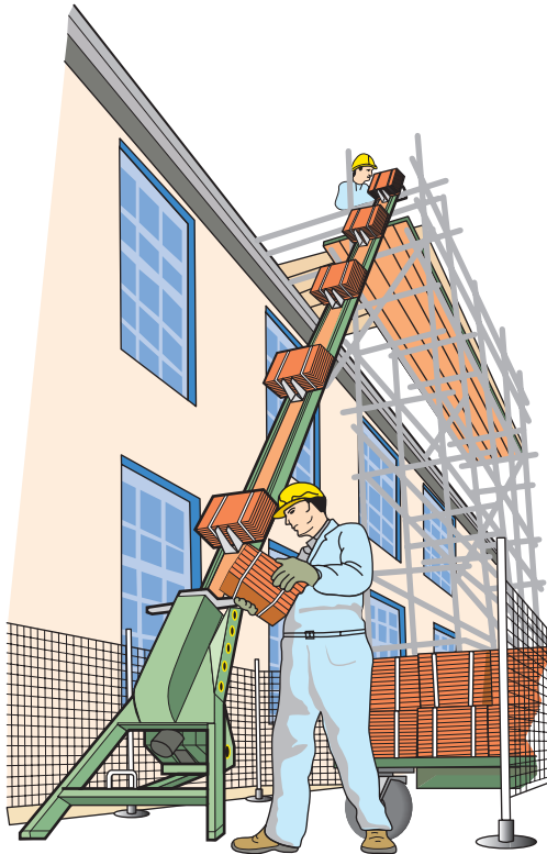
Figure 7.9 Brick elevator to get materials safely to the top of a scaffold.
