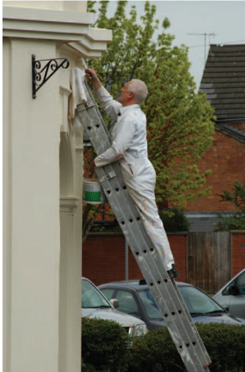
Figure 1.7 Painter at work from a ladder.
