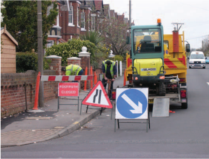
Figure 4.5 Shutting off a footpath to protect workers and the public.
