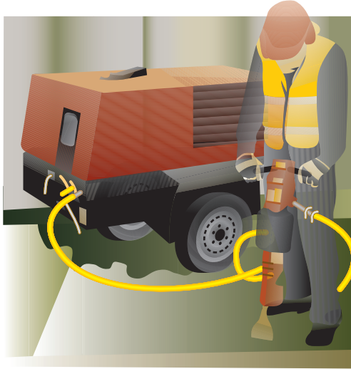
Figure 6.8 Road breaker may cause hand arm vibration problems.
