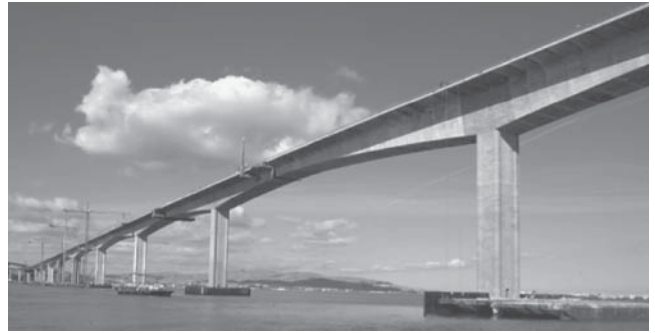
Benicia-Martinez Bridge, California.
