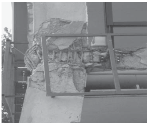
Column–girder connection (joint). Courtesy of Murat Saatcioglu and John Gardner
