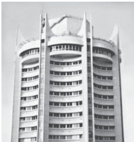
Circular beams in an office building.
