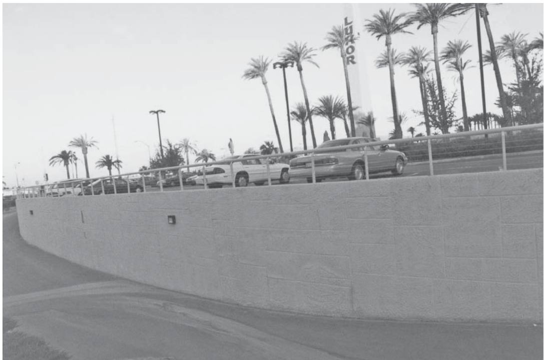
Retaining wall in a parking area.
