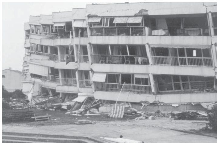
Collapse of frame concrete structures due to an earthquake. Courtesy of Murat Saatcioglu and John Gardner.
