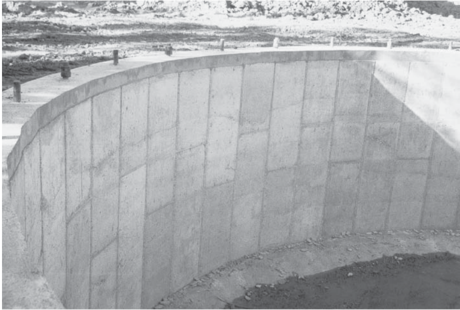
Reinforced concrete retaining wall.
