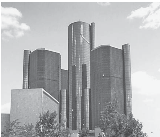
Renaissance Center, Detroit, Michigan.
