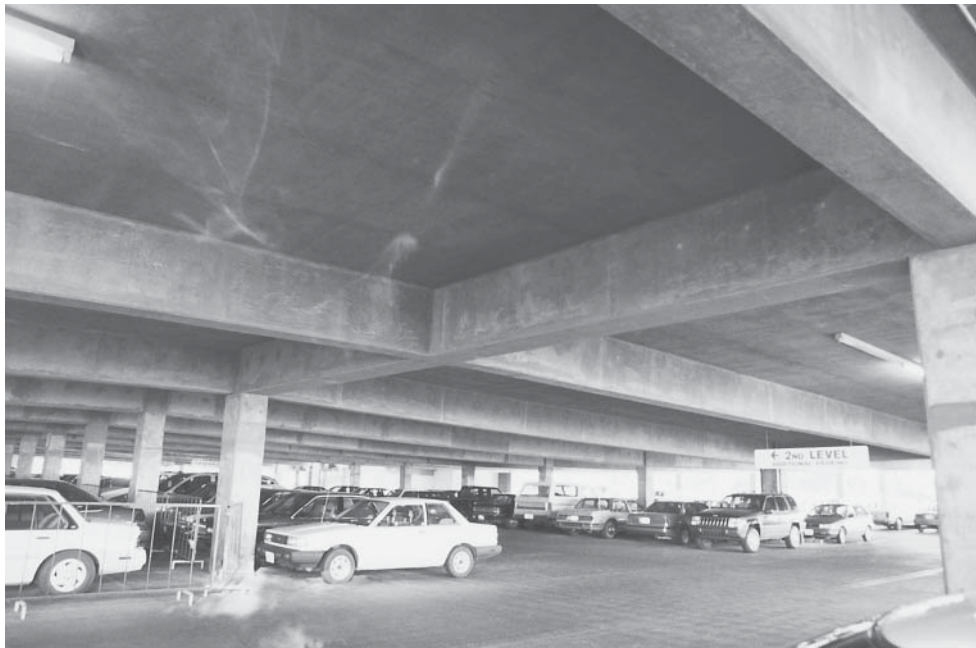
Slab on beams.
