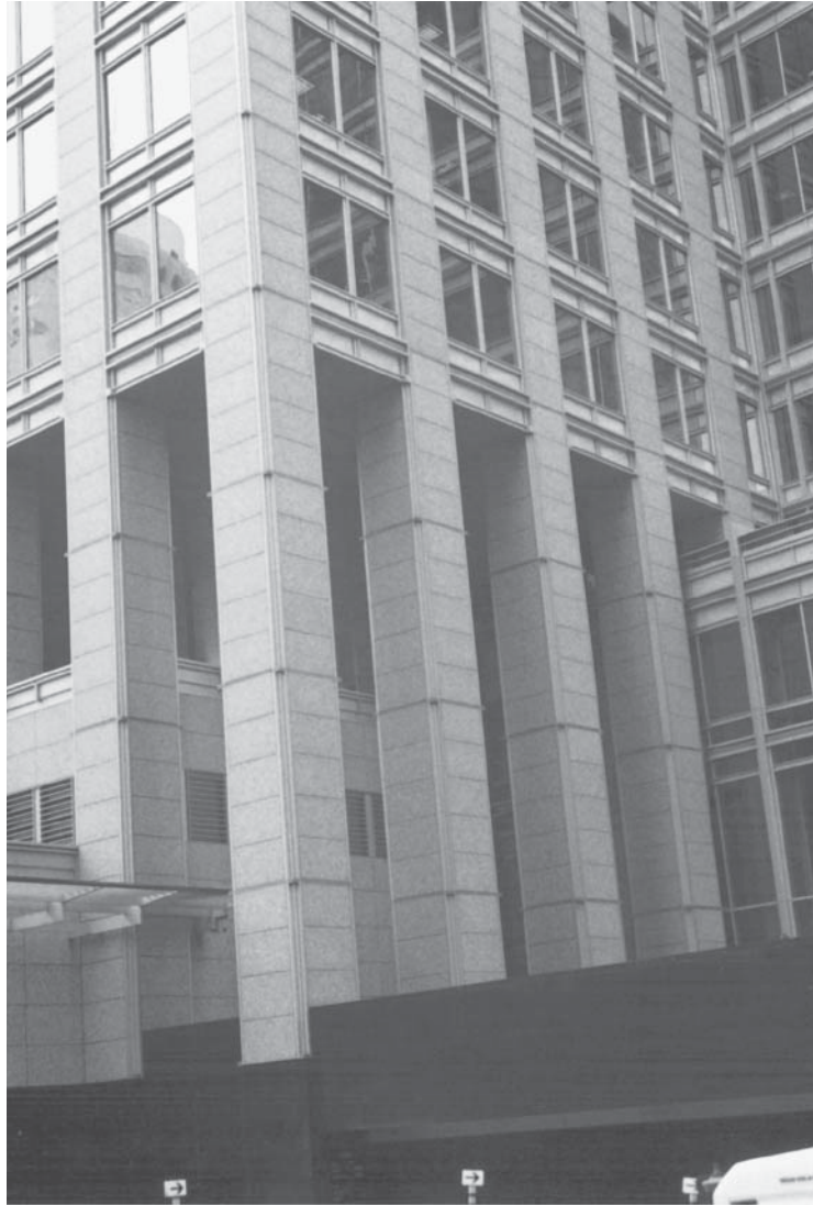
Long columns in an office building.
