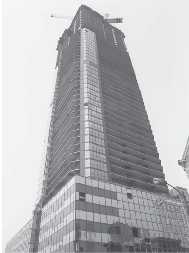
Office building under construction, Chicago, Illinois.
