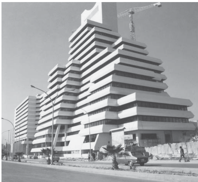
Reinforced concrete office building, Amman, Jordan.
