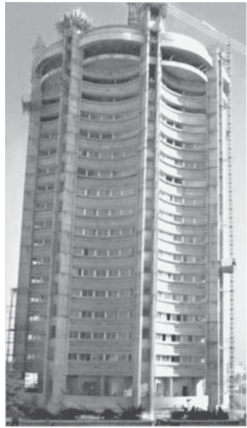
Curved beams in an office building.
