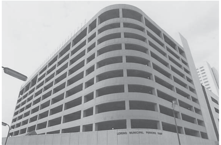
Reinforced concrete parking structure, Minneapolis, Minnesota.
