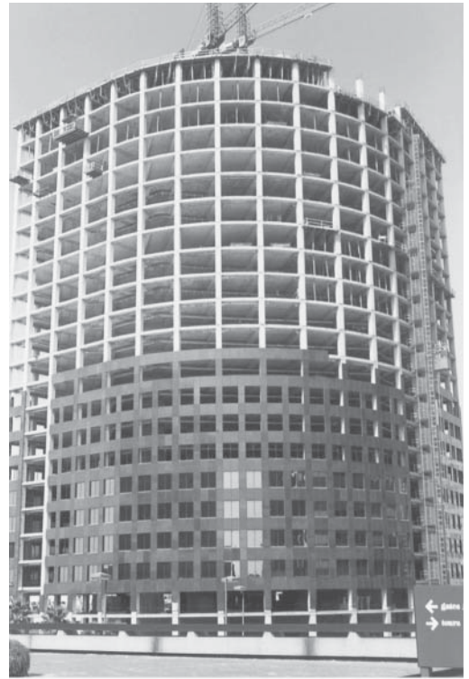
Office building under construction, New Orleans, Louisiana.
