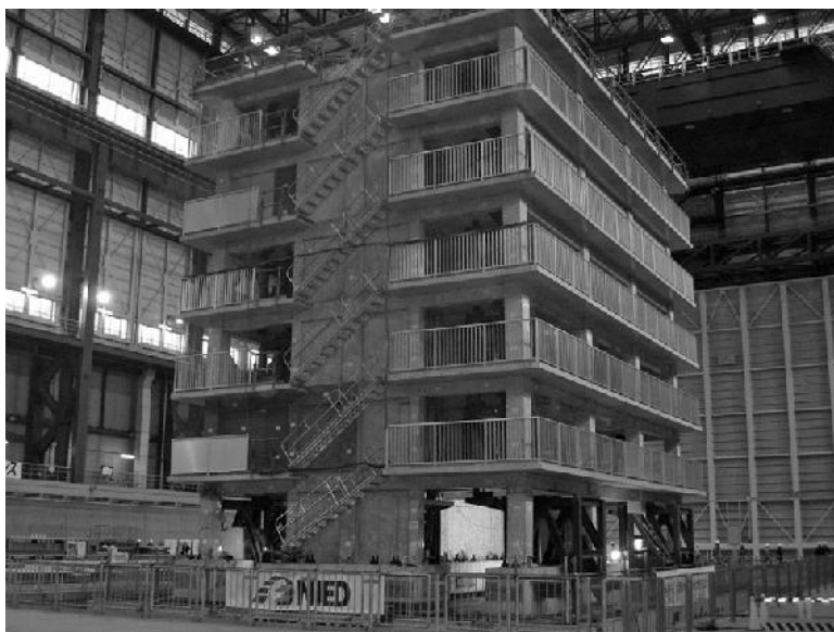
14.2 The reinforced concrete wall-frame building specimen.
