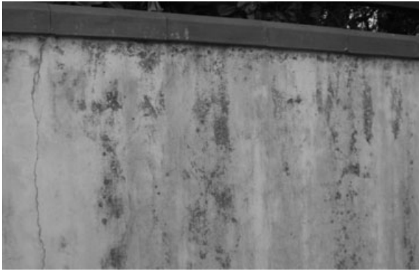
12.2 The availability of moisture is essential for the growth and development of algal species.
