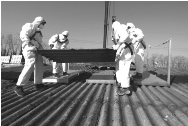
7.6 Workers removing asbestos-cement roofing.
