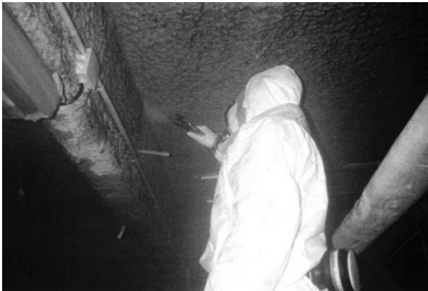
7.7 Worker removing indoor friable asbestos.
