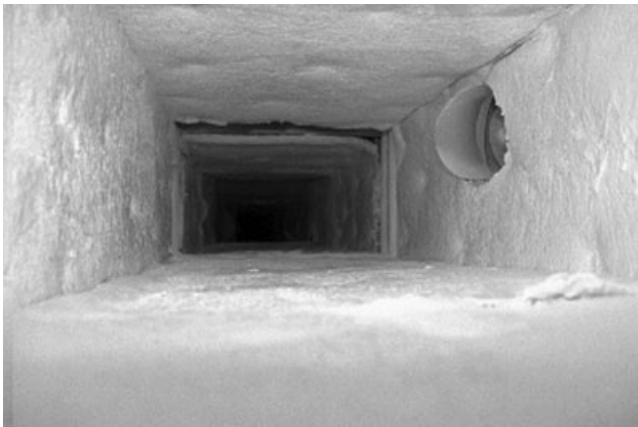
13.7 HVAC duct encapsulant lining.
