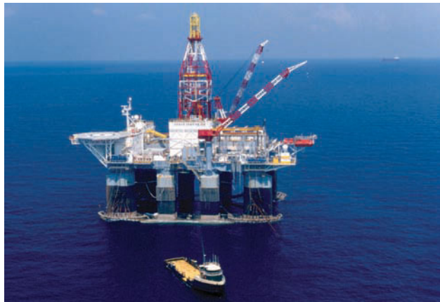
Figure 4.1 Large welded oil platform
