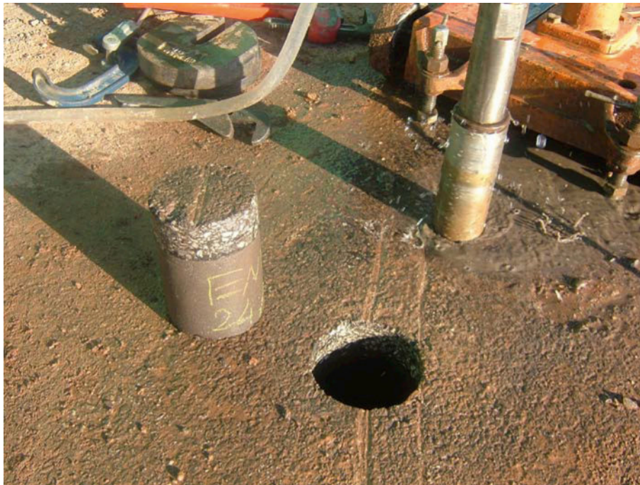
FIGURE 27.7 Core Recovered From Road Slab
