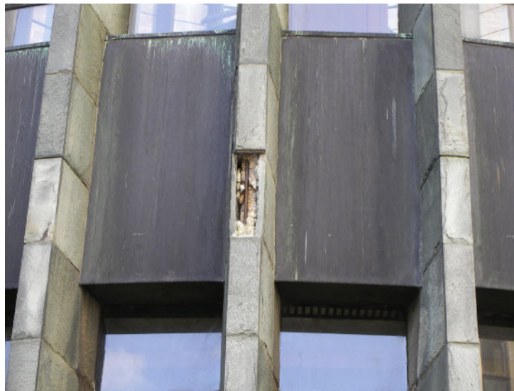
FIGURE 25.6 Carbonated Concrete on a 50-Year-Old Chapel at Coventry Cathedral
