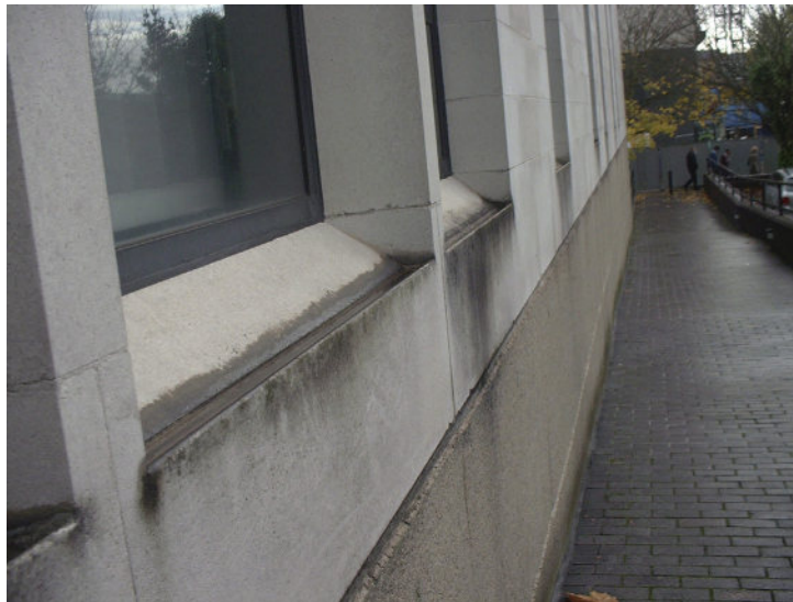
FIGURE 26.3 Poor Detail of Precast Sill That Does not Shed Water
