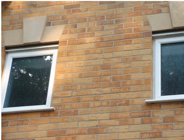
FIGURE 34.8 Well Planned Brickwork
