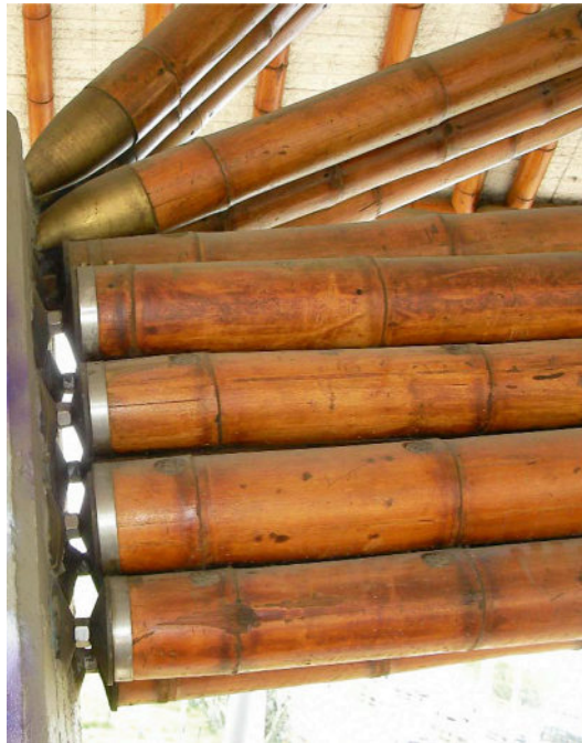
FIGURE 33.11 Tidy Metal End Connectors on Bamboo
