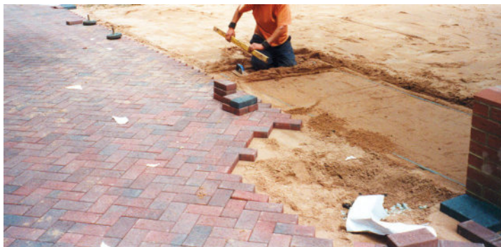
FIGURE 34.5 Brick Paving with Concrete Bricks
