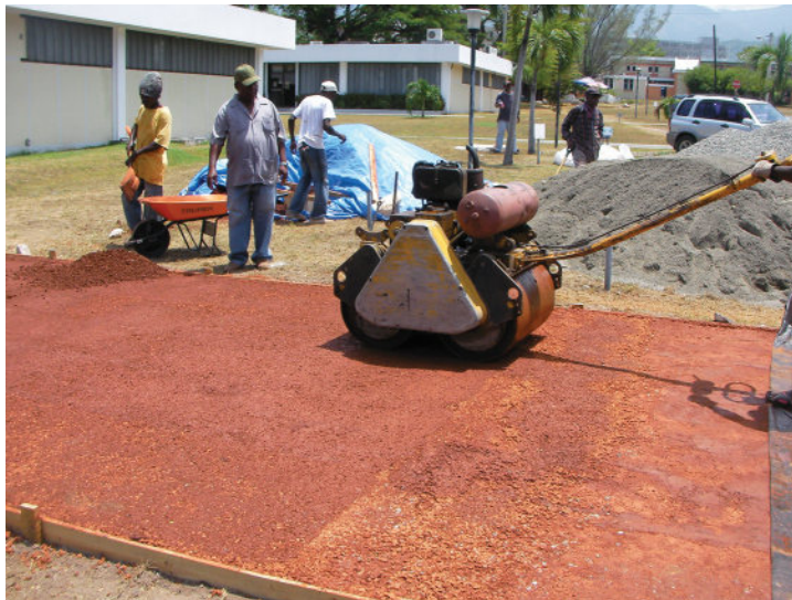
FIGURE 41.1 Roller Compacted Zero Cement Concrete in Jamaica
