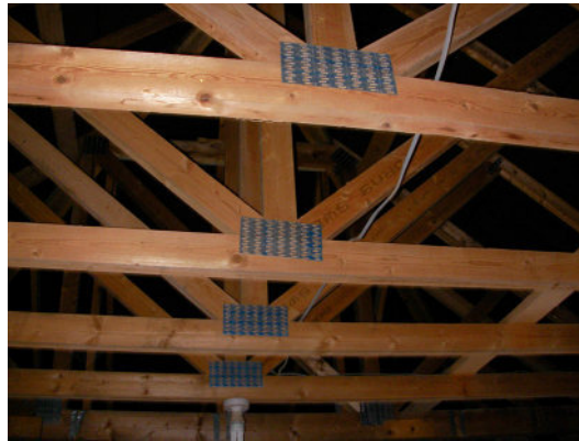
FIGURE 33.6 Typical Application of Metal Plate Fasteners
