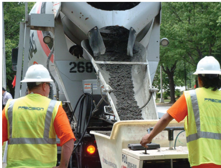
FIGURE 29.1 Pervious (No-Fines) Concrete Being Discharged From a Truck-Mixer
