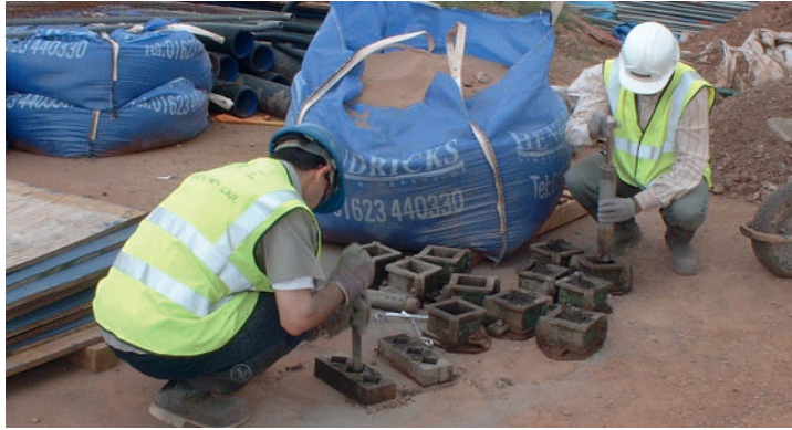
FIGURE 22.11 Compacting Test Cubes on Site
