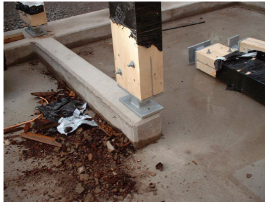
FIGURE 33.7 Metal End Connector to Keep Timber Frame Dry (Note the Polythene Wrapping Used to Keep the Timber Dry During Construction)
