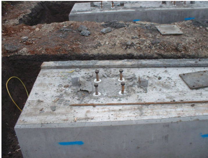
FIGURE 28.4 Holding Down Bolts With the Expanded Polystyrene Void Formers Still in Position Around Them
