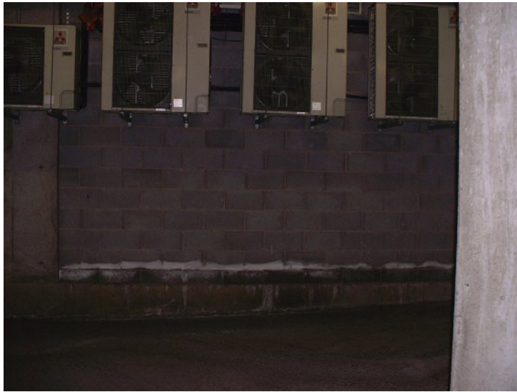
FIGURE 25.11 Salt Accumulation on Concrete Masonry Blocks in a Parking Garage
