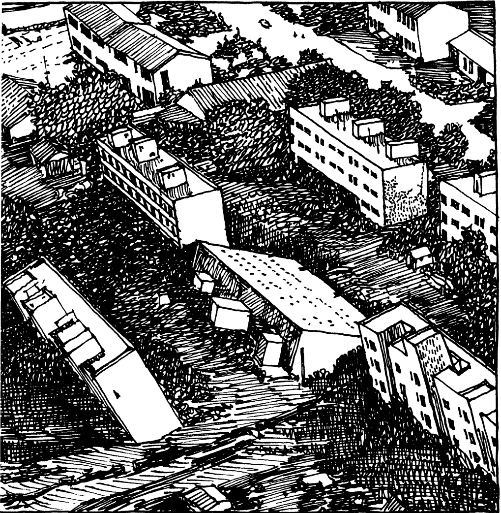
6.6 Niigata Apartment Buildings: After the Earthquake
