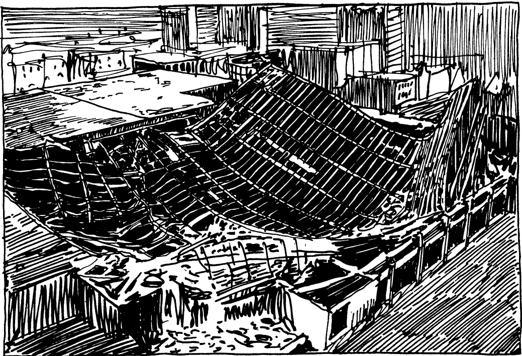
4.10 Hartford Center Roof: after the Collapse
