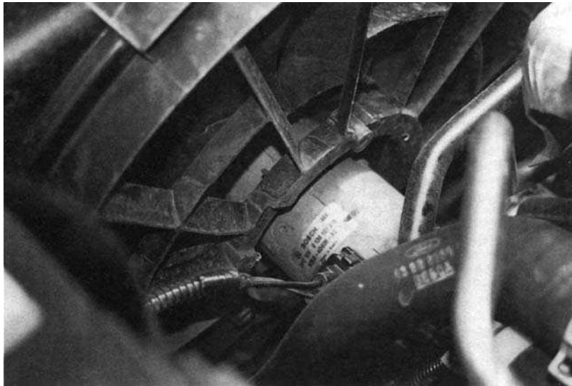
Figure 9.23 Cooling fan motor
