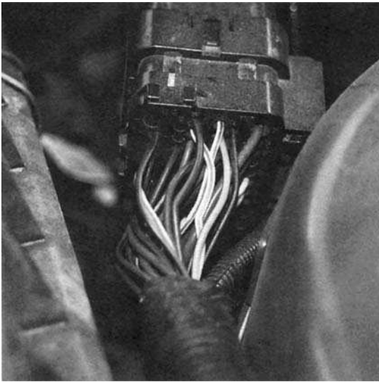
Figure 8.14 Check security of all connectors such as the one shown here
