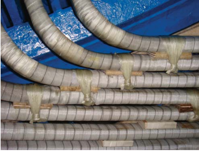
Figure 18.2 Butterfly ties at interbar blocking.
