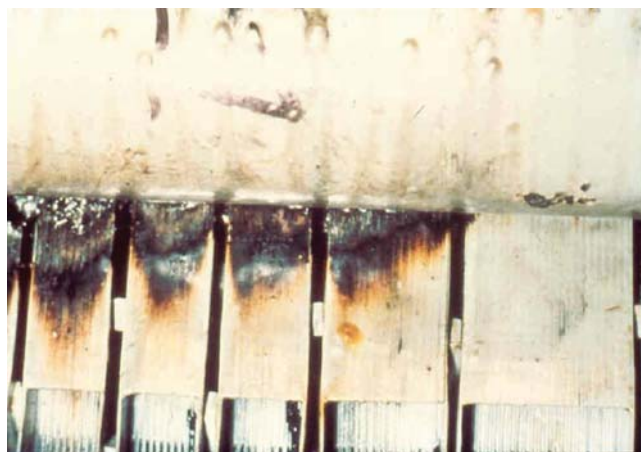
Figure 13.12 Back of core burning at key bar.
