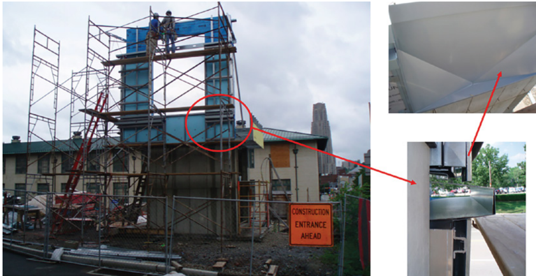
FIGURE 7.8 Exterior enclosure mockup assembly
