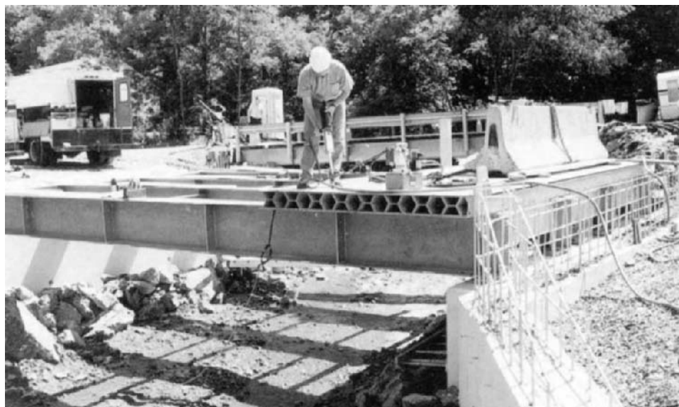
Figure 8.15 Installation of FRP modules (Rao and Craigo, 1999).
