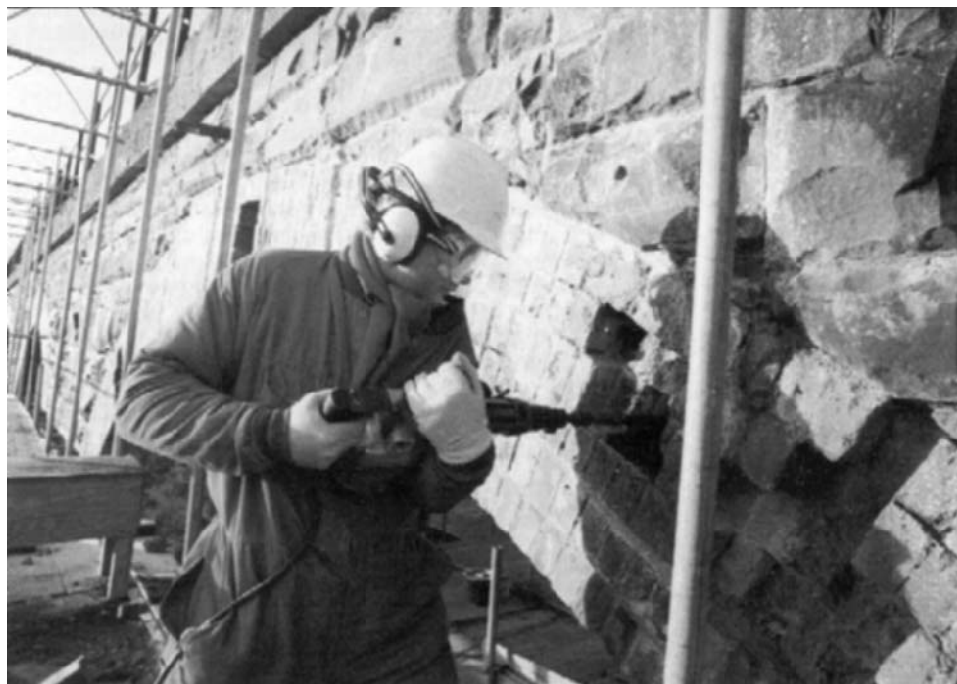
Figure 6.2(b) removing damaged brickwork.
