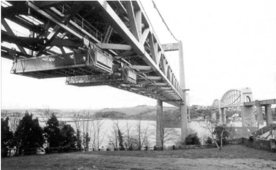
Figure 2.22 Aluminium gantries slung under the Tamar Bridge.
