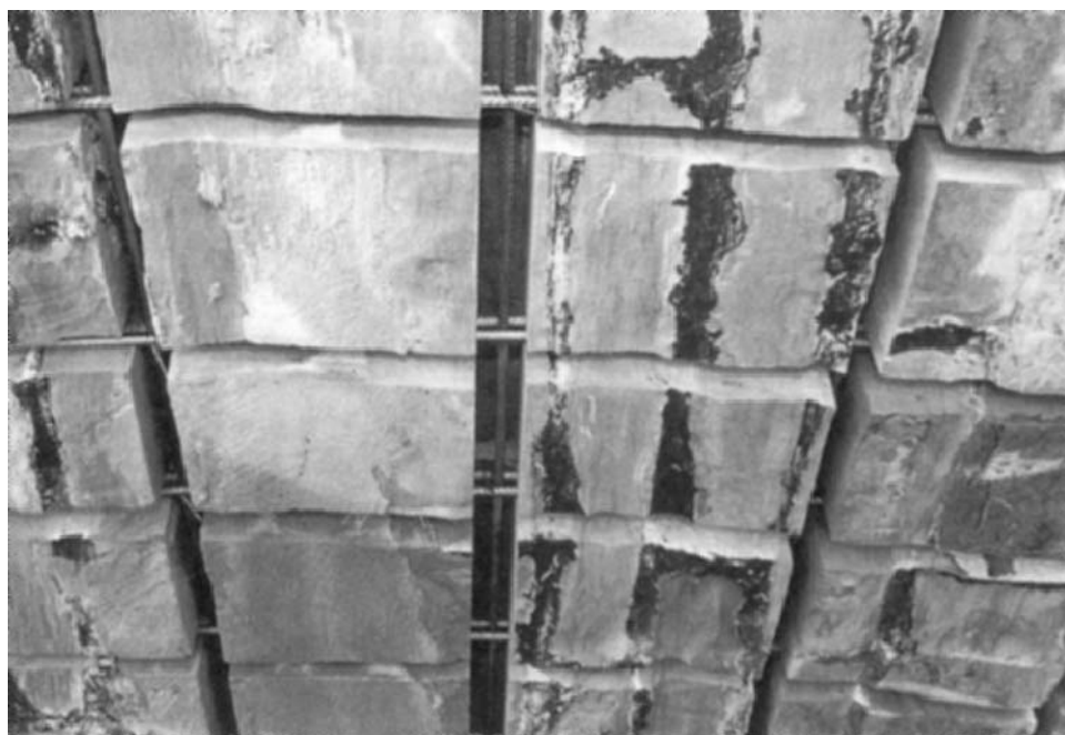
Figure 7.25 General and close-up views of MARS repairs to Well'i'th Lane Canal Bridge (Minnock 1997).
