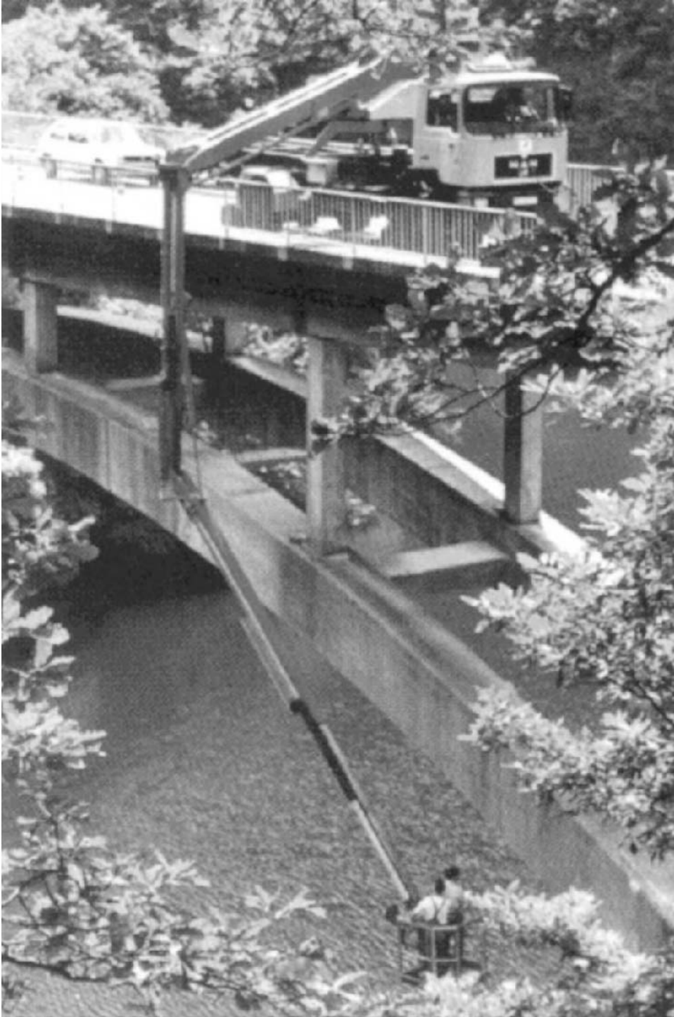
Figure 2.20(b) Cherry picker in use for inspecting a concrete arch bridge.
