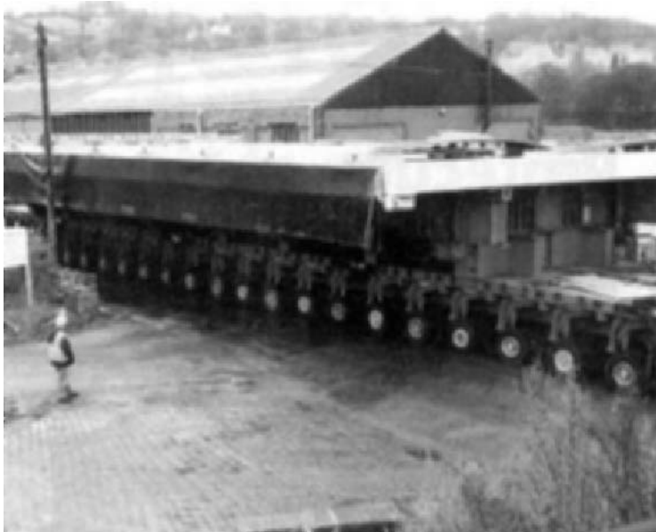
Figure 8.23 (a) Plan of bridge and (b) low loader moving 850 t deck (Hayward, 1999).
