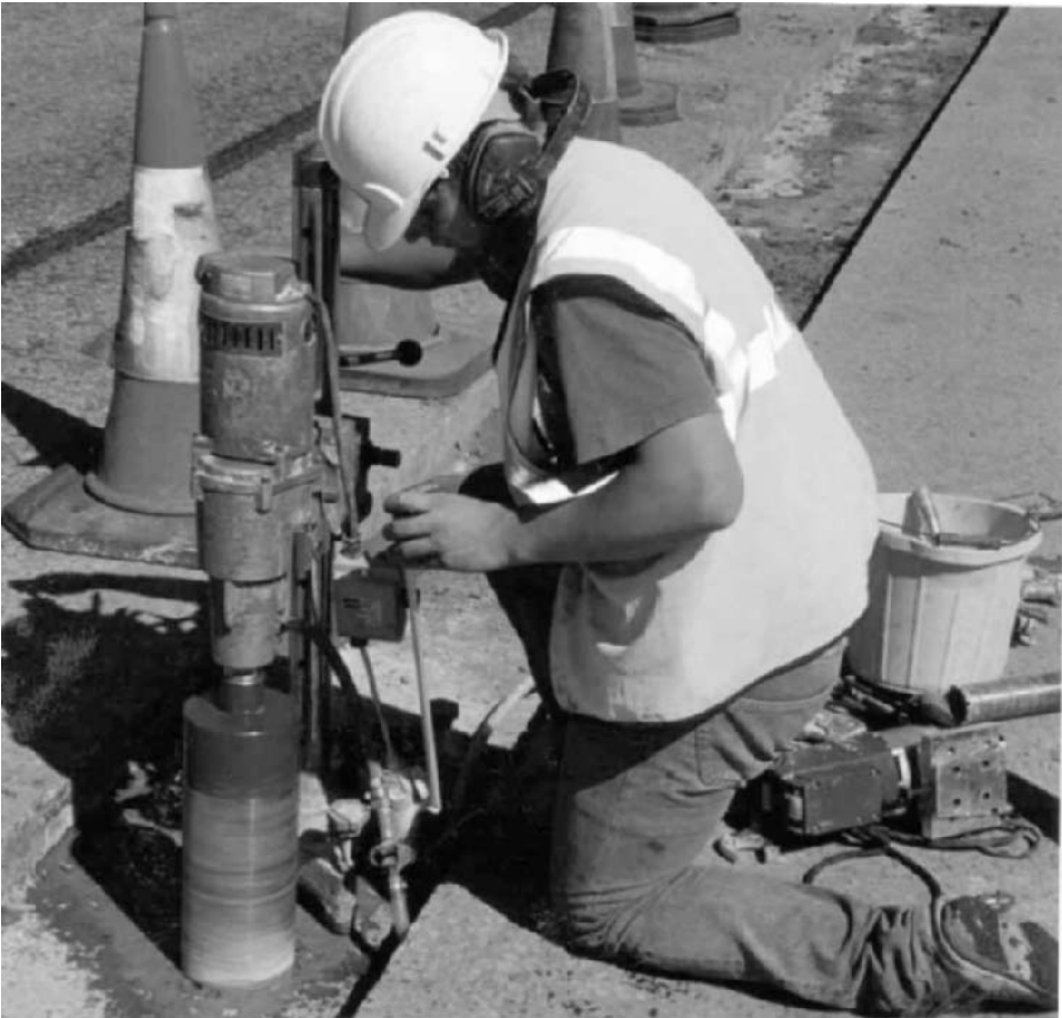
Figure 4.23 Typical coring set-up.
