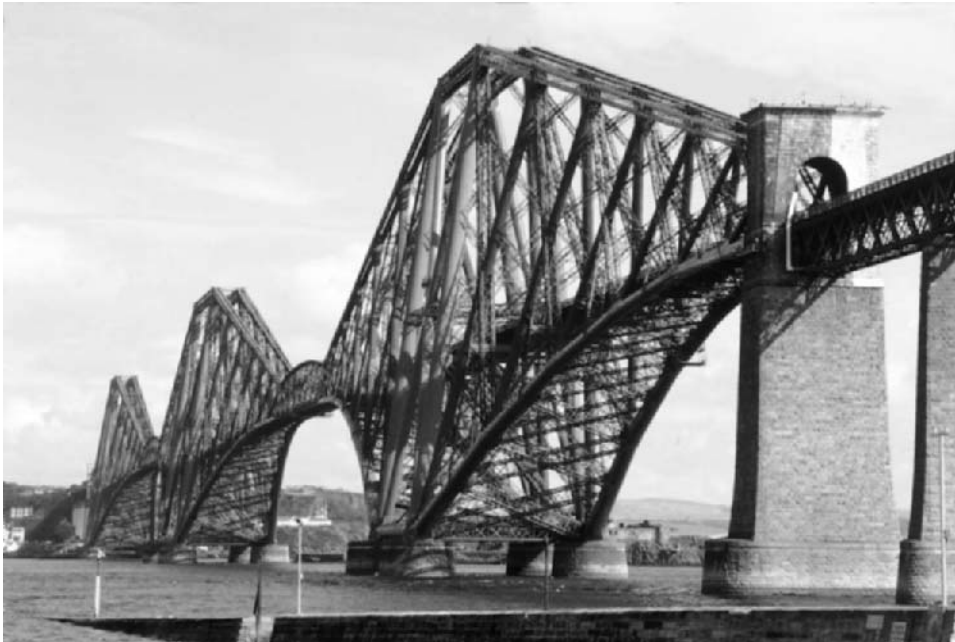
Figure 1.14 Forth Railway Bridge (see colour plate section).
