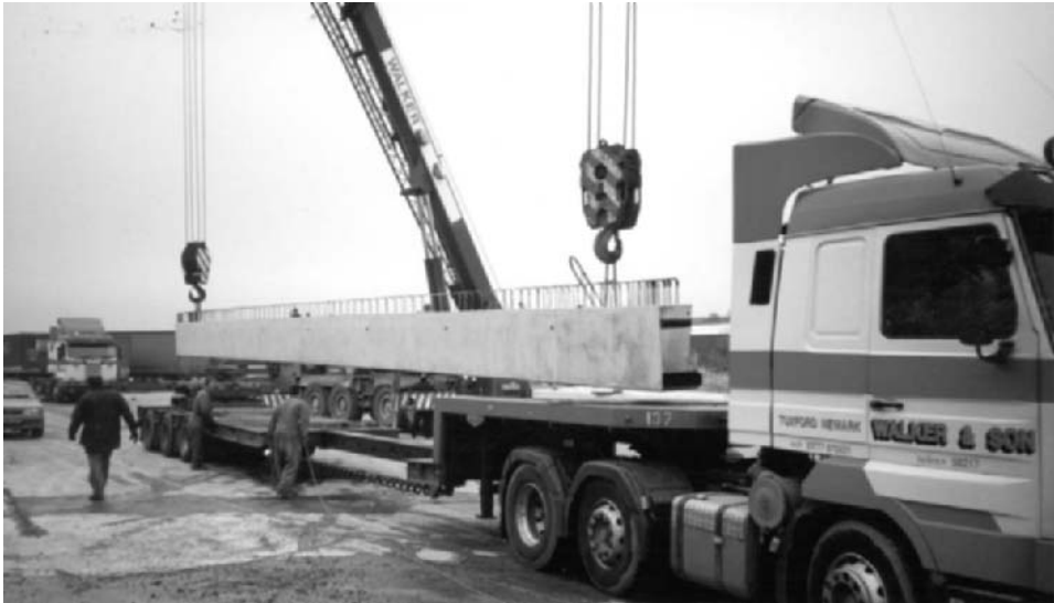
Figure 8.17 Lifting of beams for a replacement bridge.
