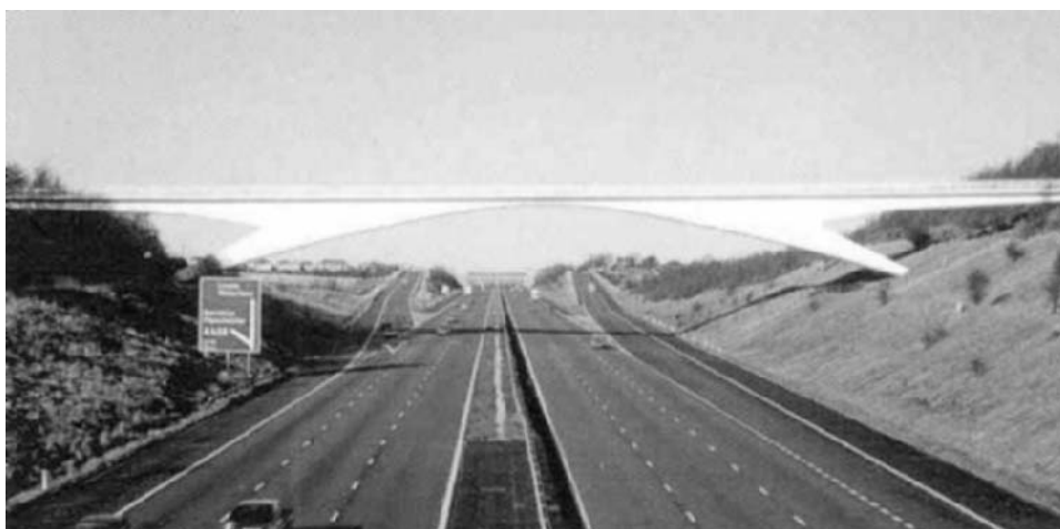
Figure 6.21 The needle eye bridge (courtesy Concrete Repairs Ltd.).
