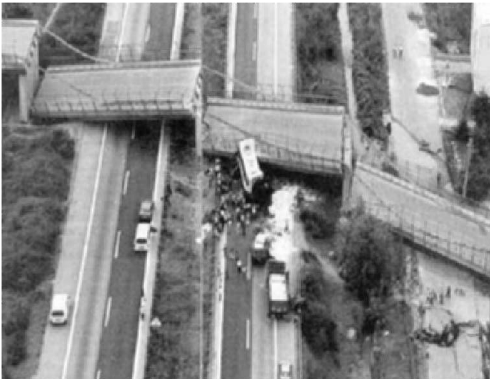
Figure 8.32 Collapse of a viaduct due to an earthquake in Istanbul, Turkey.
