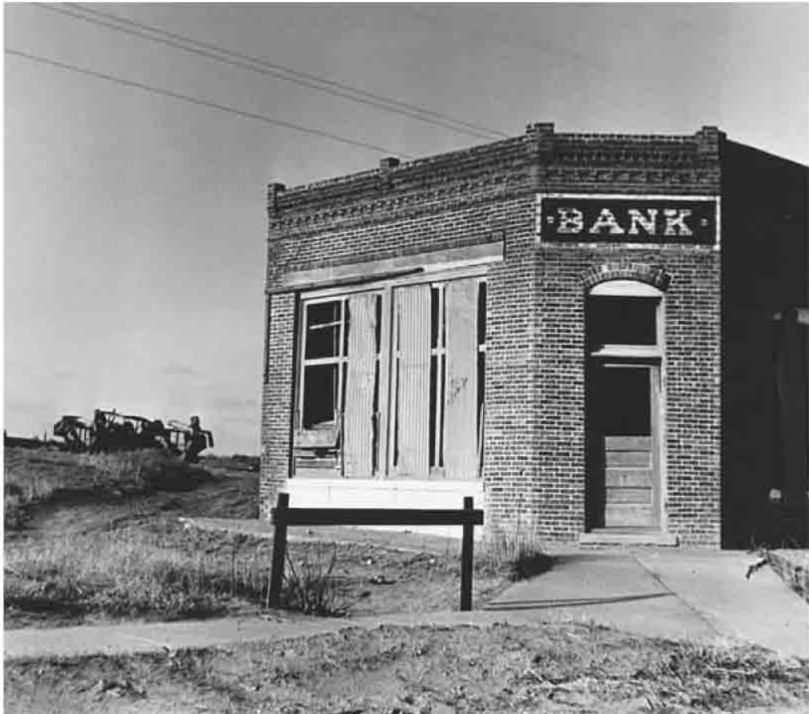
Failed bank, Kansas, 1936
