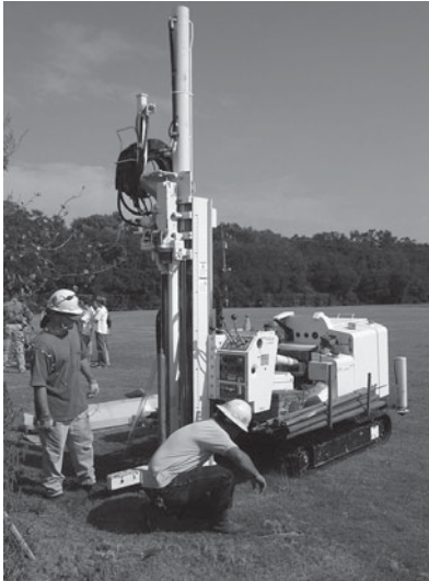
Groundwater well drilling.
