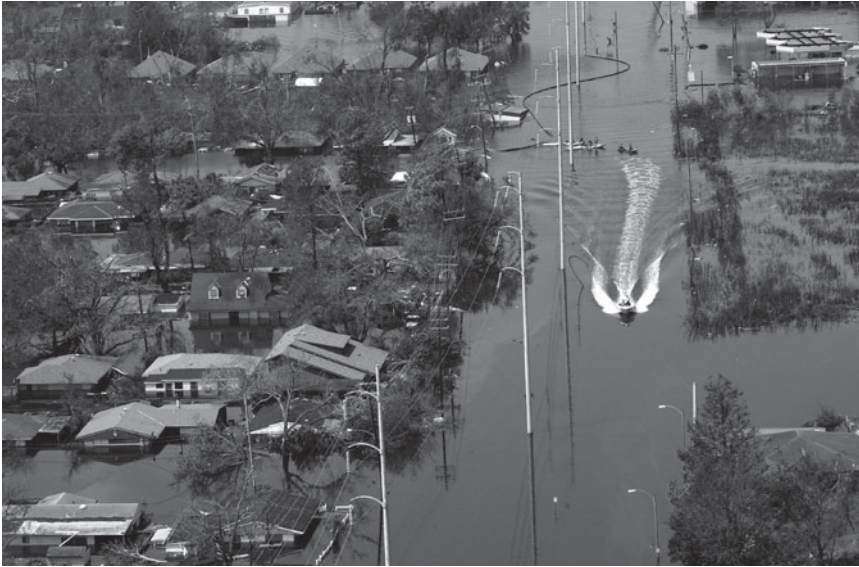
Figure 12-4c Severe New Orleans flooding due to levee breaks from Hurricane Katrina.
