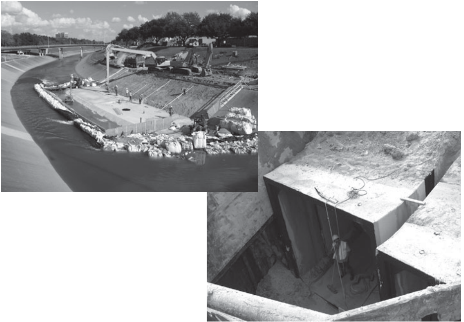
Open channel improvements in Houston, Texas.
