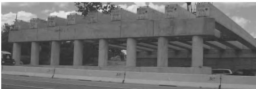
Figure 6.2-6 Eight-column pier.
