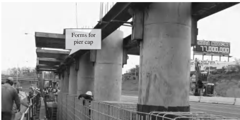
Figure 6.1-7 Forming for pier cap after completing columns.
