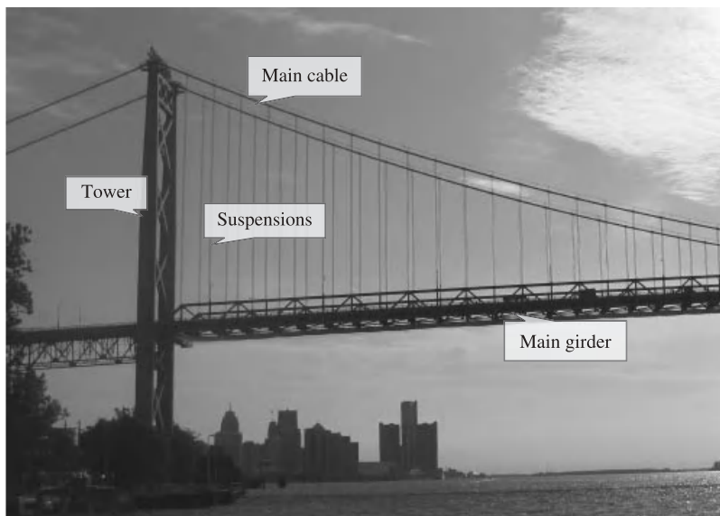
Figure 4.3-6 Main structural components in suspension bridges.
