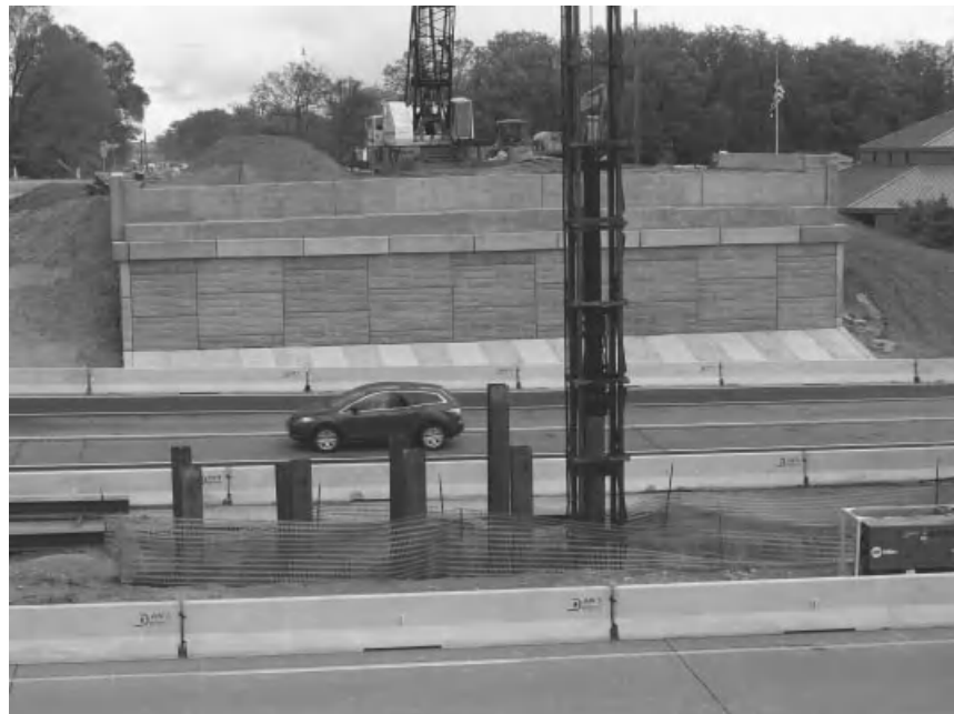
Figure 6.4-5 Driven piles for bridge pier foundation.
