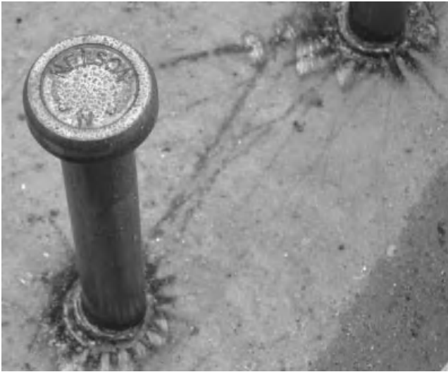
Figure 4.5-19 Shear stud welded on steel beam top flange.
