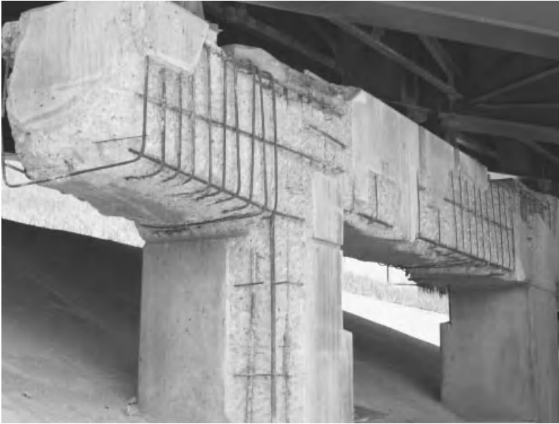
Figure 6.1-10 Concrete pier being rehabilitated.
