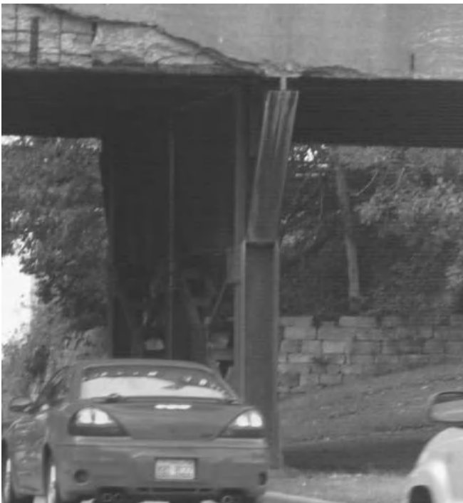
Figure 6.2-9 Steel frame bridge pier.
