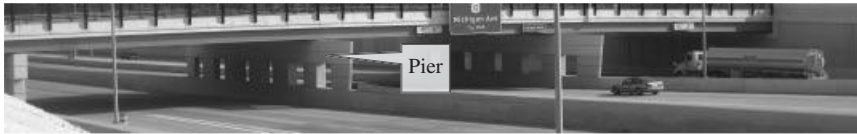
Figure 6.1-1 Highway bridge piers with multiple concrete columns.
