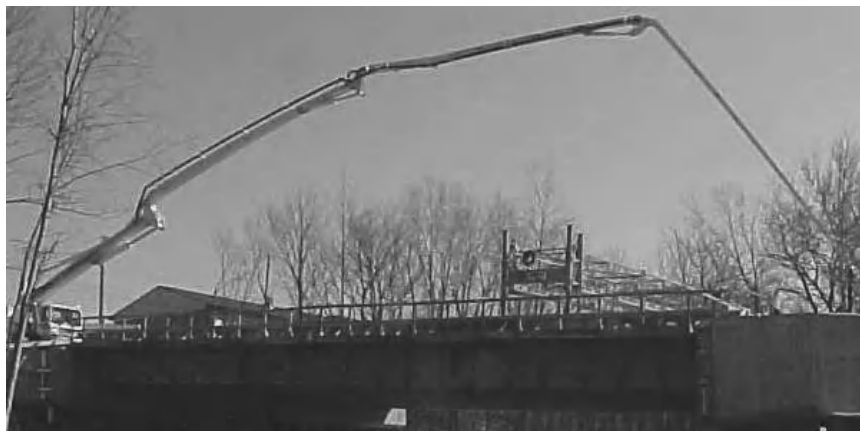
Figure 1.3-1 Concrete deck placement using a concrete pump.
