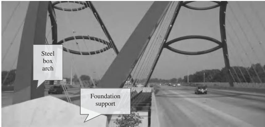
Figure 6.4-1 Foundation support to twin-arch bridges.
