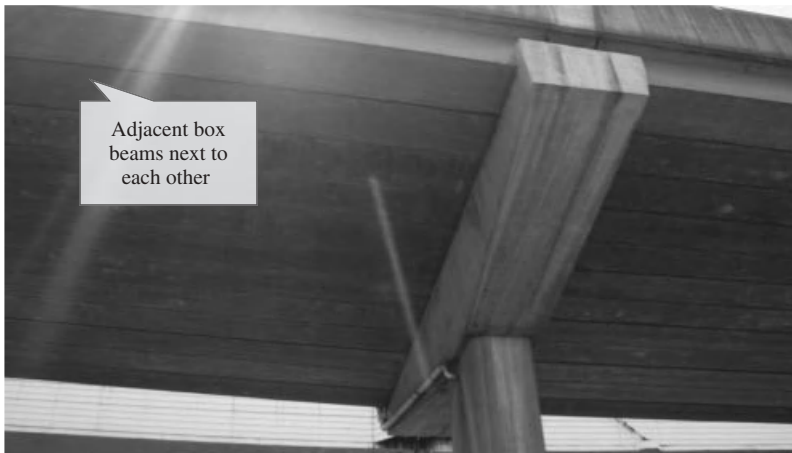
Figure 4.8-2 Highway bridge with prestressed concrete adjacent box beams.
