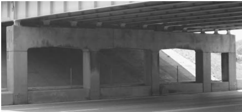
Figure 6.2-5 Five-column pier.
