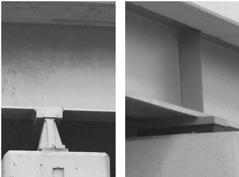
Figure 5.2-13 Contrast of (left) steel and (right) elastomeric bridge bearings.
