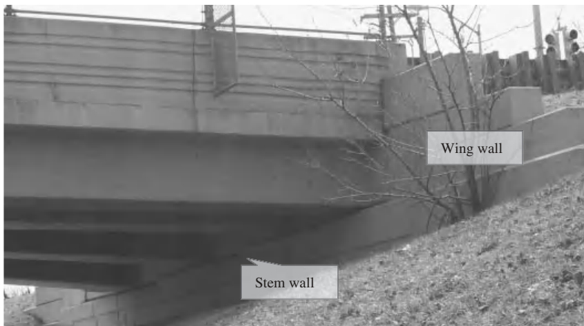
Figure 6.3-1 Stub abutment parallel wingwall in service.
