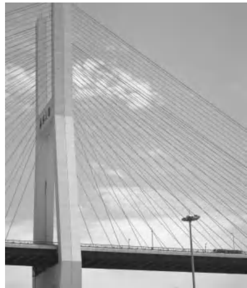
Figure 4.2-4 Cable-stayed bridge system.
