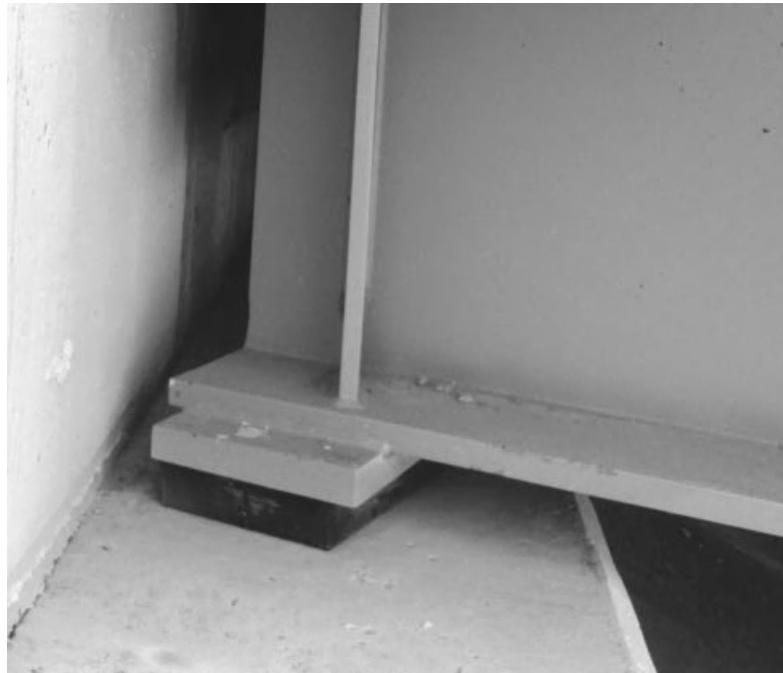
Figure 5.2-14 Elastomeric bridge bearing pad.
