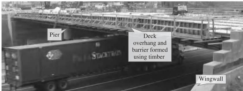
Figure 4.5-15 Deck construction with underneath roadway open to traffic.
