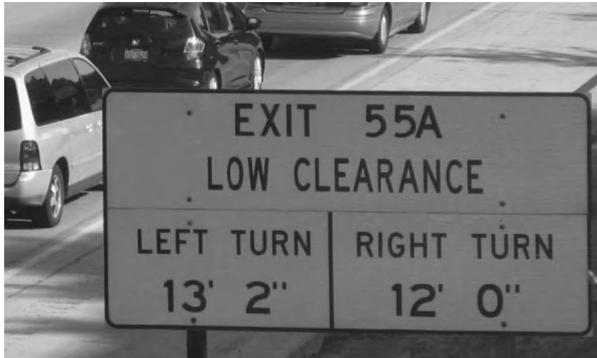
Figure 2.5-1 Inadequate clearance indicated by a highway sign.
