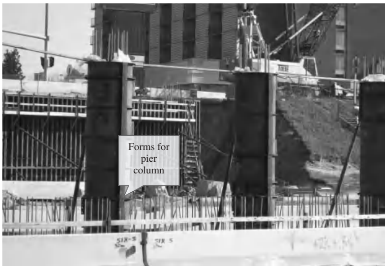
Figure 6.1-6 Forming for pier columns.
