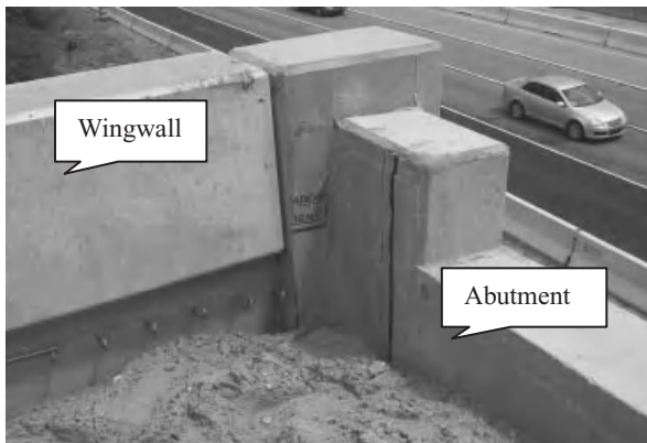
Figure 3.2-5 Soil retained by abutment seen in construction before superstructure erection.
