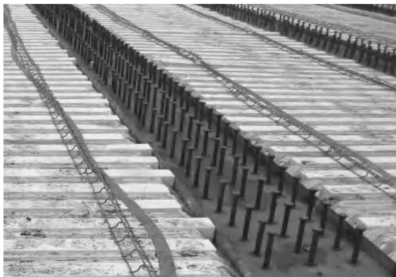
Figure 4.7-11 Shear stud arrangement on steel beam.
