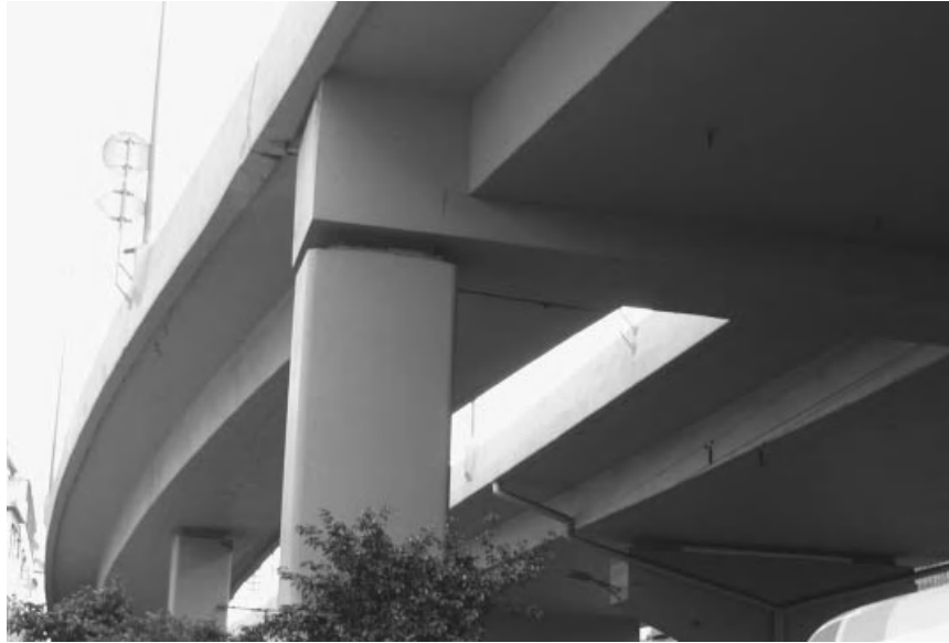
Figure 1.2-3 Curved concrete box beam bridge.
