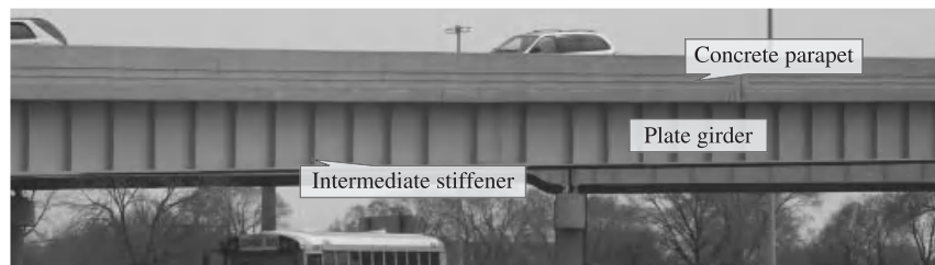
Figure 4.5-14 Steel plate girder highway bridge.
