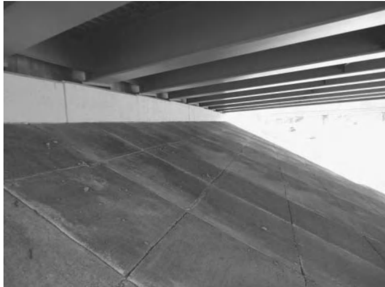
Figure 6.3-3 Partial-depth abutment supporting steel superstructure.
