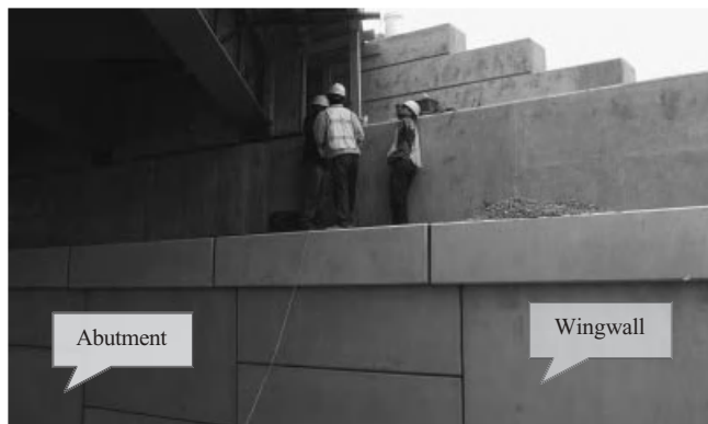
Figure 6.1-4 Highway bridge abutment with parallel wingwall.
