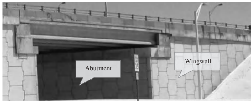
Figure 6.1-3 Highway bridge abutment with orthogonal wingwall.
