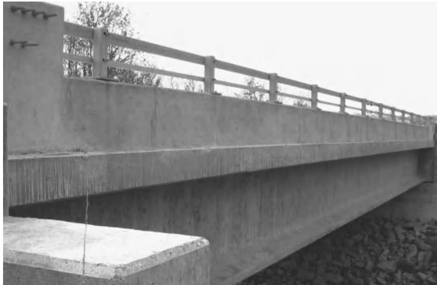
Figure 1.2-4 Prestressed concrete I-beam bridge of single span.
