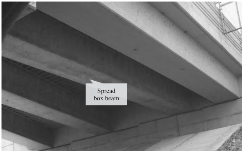
Figure 4.8-1 Highway bridge with prestressed concrete spread box beams.
