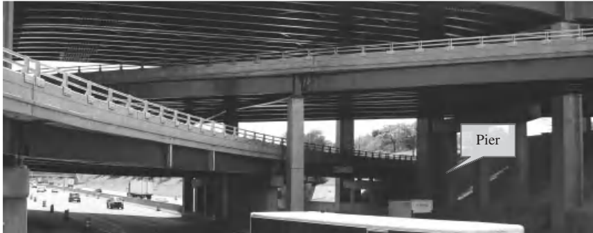
Figure 6.1-2 Bridge piers for crossing highways.
