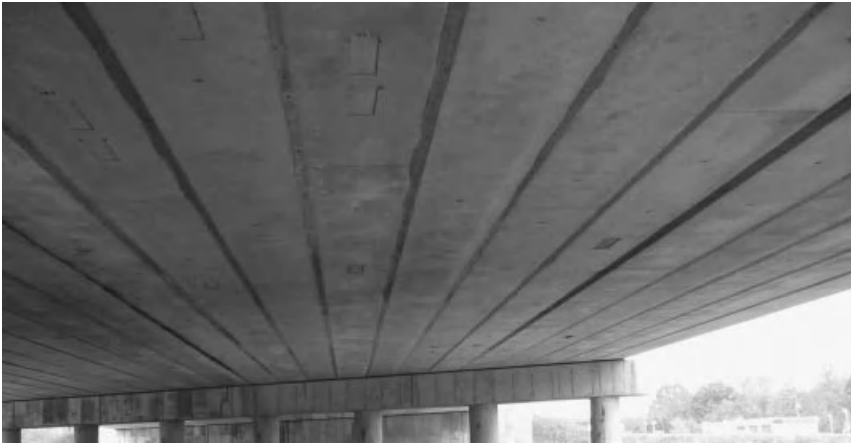
Figure 1.2-5 Prestressed concrete box beam bridge.
