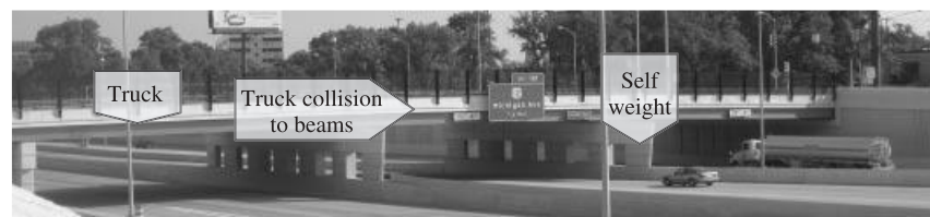
Figure 4.1-1 Typical loads on highway bridge superstructure.
