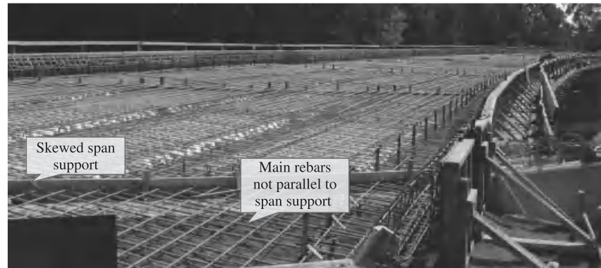
Figure 4.5-8 Reinforcement layout in skewed bridge.
