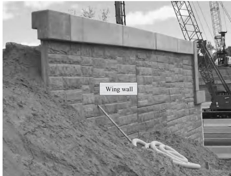
Figure 6.6-2 Wingwall in bridge abutment.
