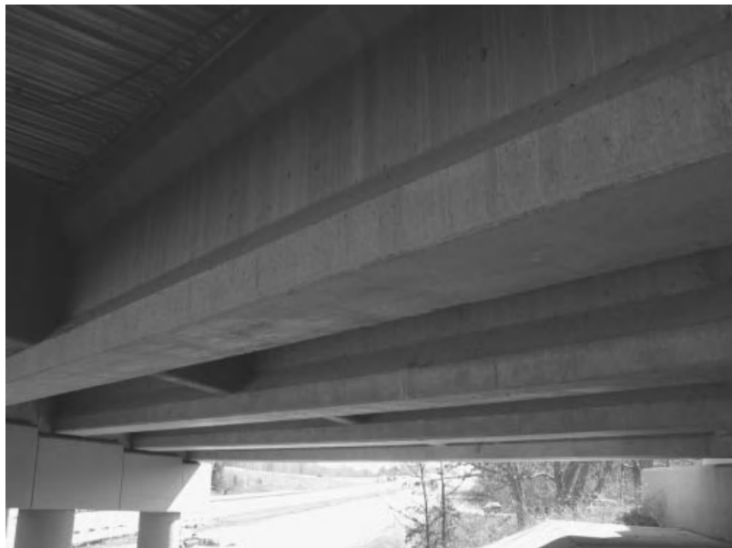
Figure 4.8-4 Prestressed concrete I-beam superstructure with diaphragms.
