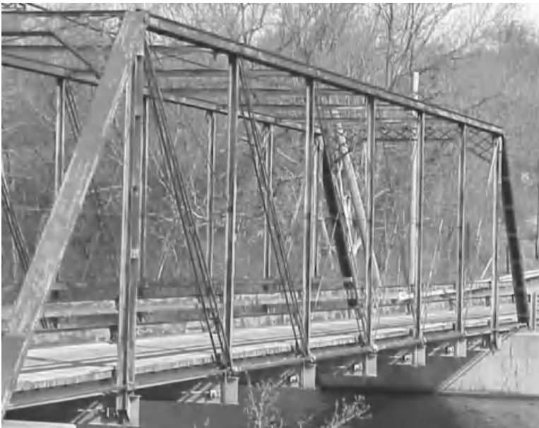
Figure 1.2-6 Steel truss bridge.
