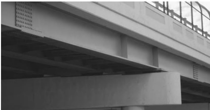
Figure 1.2-2 Continuous steel beam bridge.
