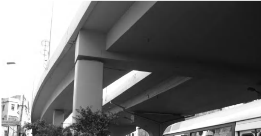
Figure 6.2-4 Two-column pier supporting concrete unibox beam.
