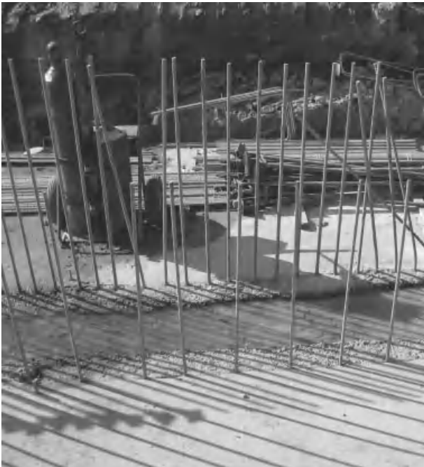
Figure 6.1-11 Abutment footing top with anchored epoxy-coated steel reinforcement.
