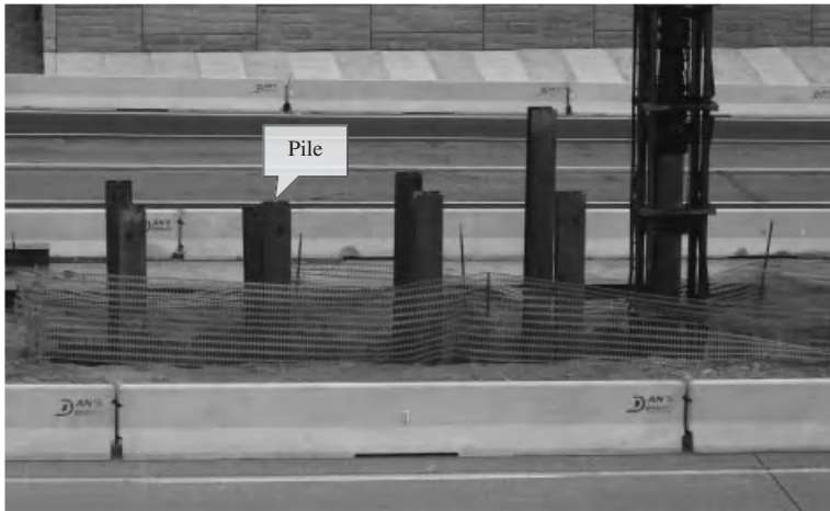
Figure 6.1-5 Piles for pier in median of two-way separated highway.
