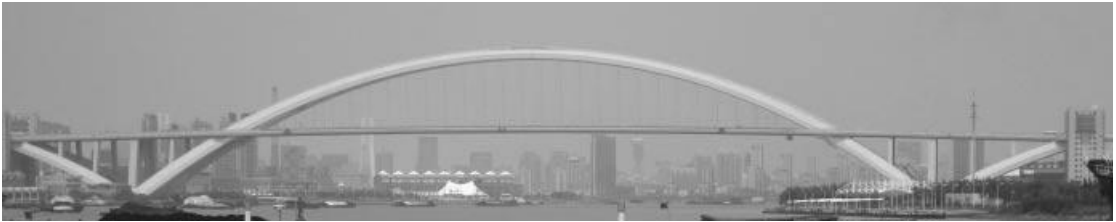
Figure 4.2-3 Arch bridge system.
