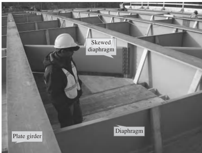
Figure 4.2-1 Beam bridge superstructure frame.
