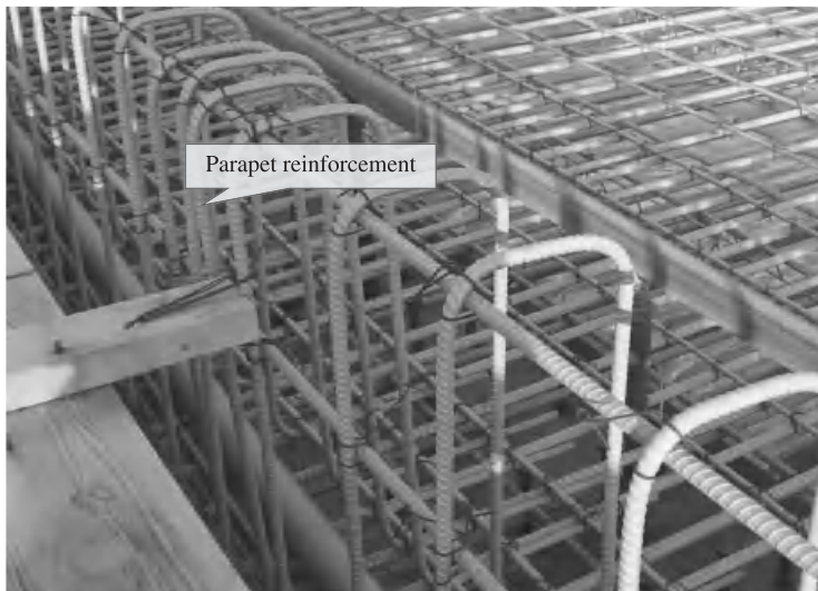
Figure 4.5-10 Steel reinforcement for parapet anchored in deck overhang.
