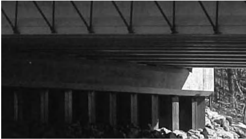
Figure 6.4-6 Driven piles as bridge abutment foundation.
