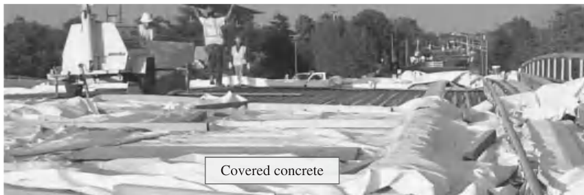
Figure 4.4-3 Burlap-covered concrete deck for curing at site.
