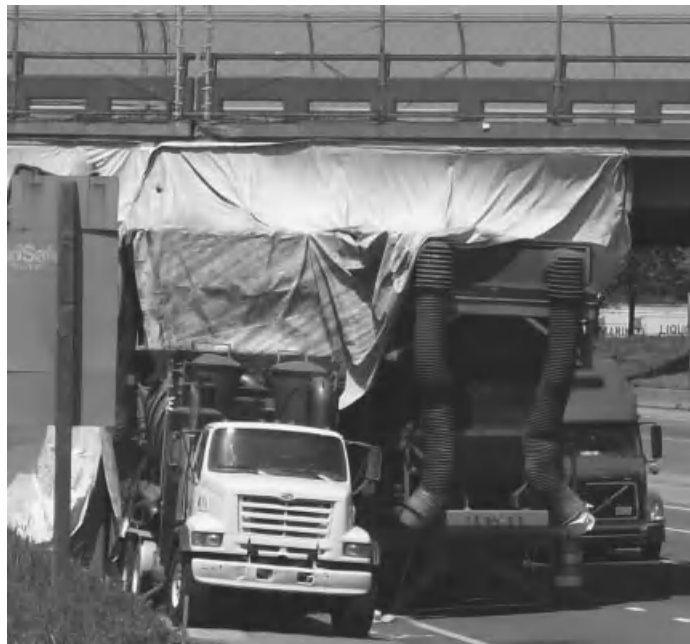
Figure 7.2-1 Vacuum confinement for removing paint from steel bridge beams to repaint.
