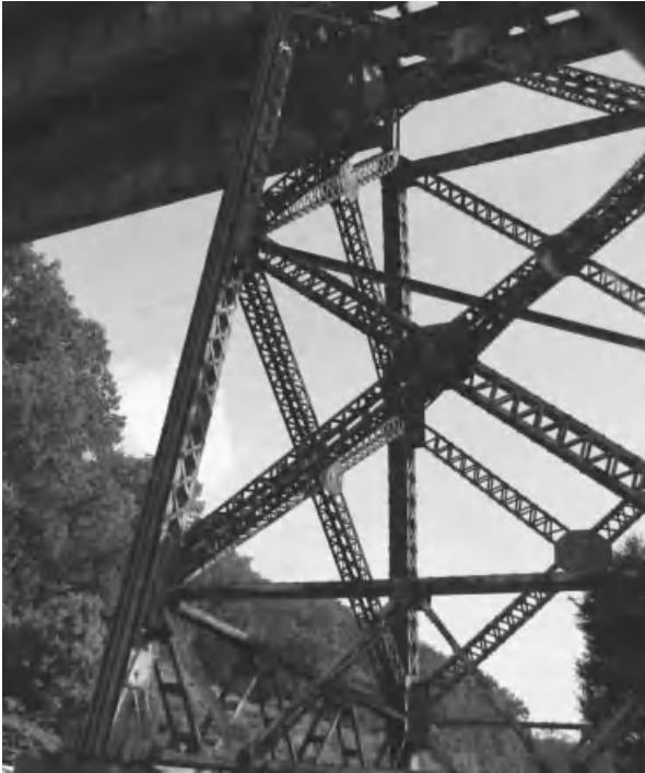
Figure 6.2-8 Steel truss bridge pier.
