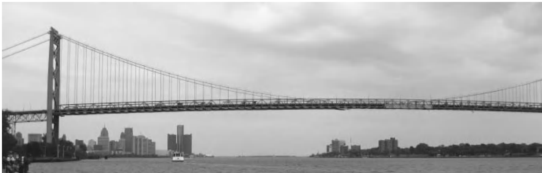
Figure 4.2-5 Suspension bridge system.
