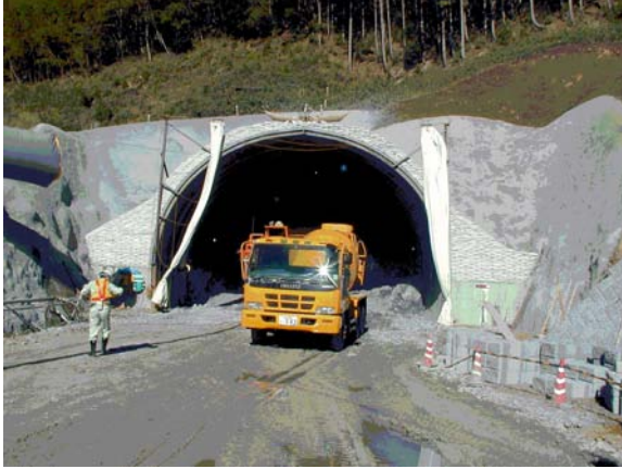
Figure 7: Suemune tunnel in Okayama, Japan.
