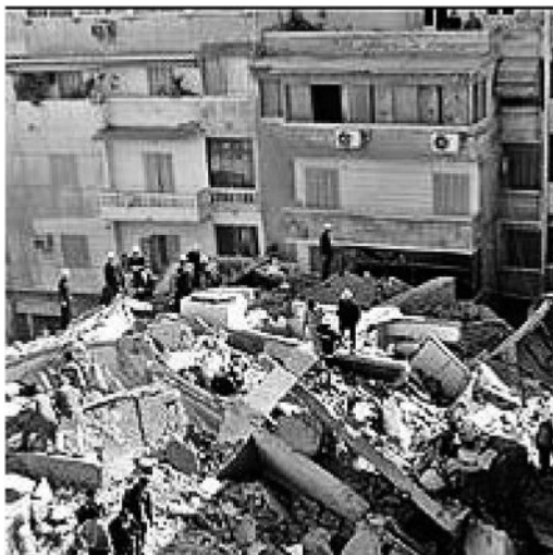
FIGURE 7.21 Building collapse in Egypt in 1993.
