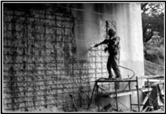
FIGURE 10.2 Using pneumatic hammer to remove wall concrete cover.
