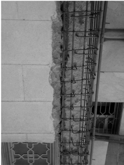
FIGURE 10.10 Adding steel for an exterior column.
