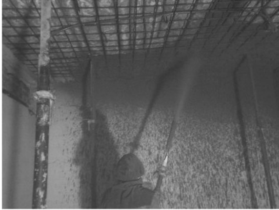
FIGURE 10.15 Shotcrete in concrete repairing.
