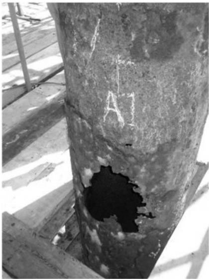
FIGURE 8.24 Corrosion of a bridge support.
