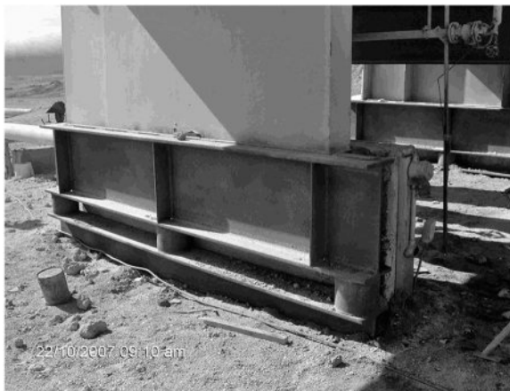
FIGURE 10.25 Repair for pedestal foundation under vessel.
