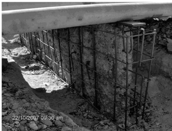
FIGURE 10.11 Repair of pedestal carrying pipelines.
