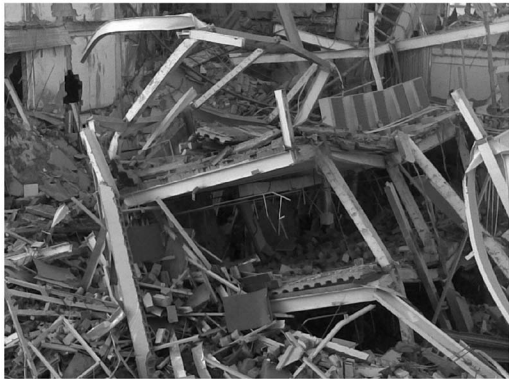
FIGURE 1.8 Dubai building collapse.
