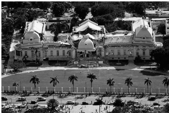
FIGURE 6.11 Collapse of Haiti palace during earthquake.
