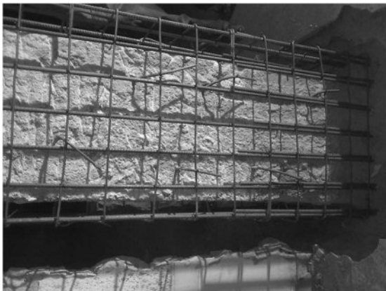
FIGURE 10.8 Steel installed for beam repair.
