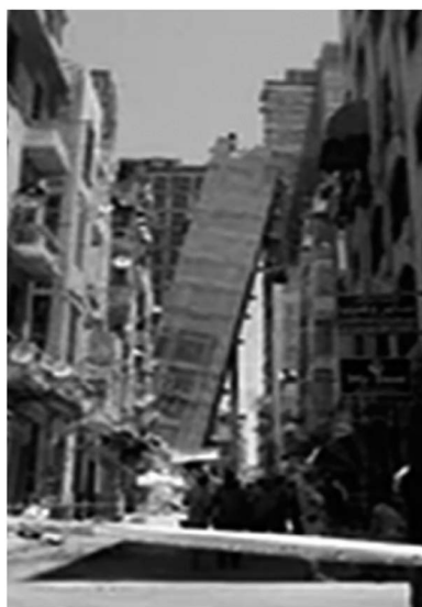
FIGURE 1.2 Building collapse at Alexandria.
