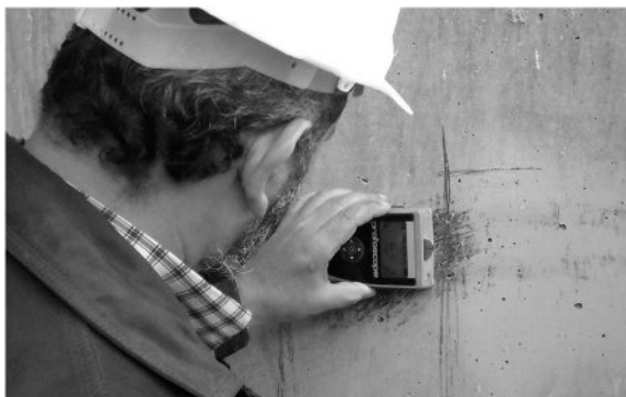
FIGURE 9.11 Concrete cover measurement.
