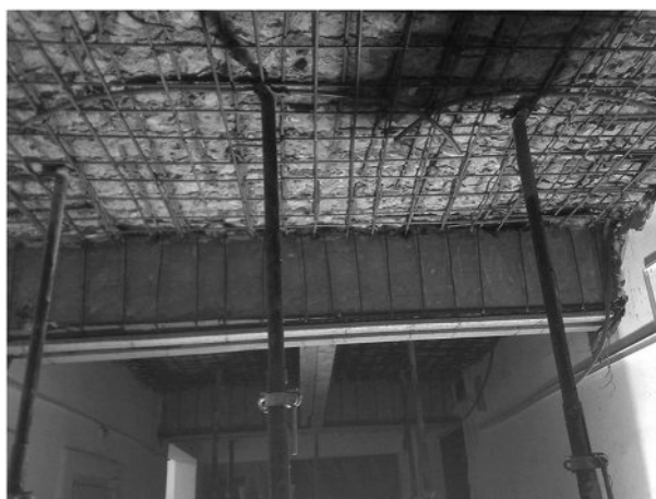
FIGURE 10.12 Slab and beam repair.
