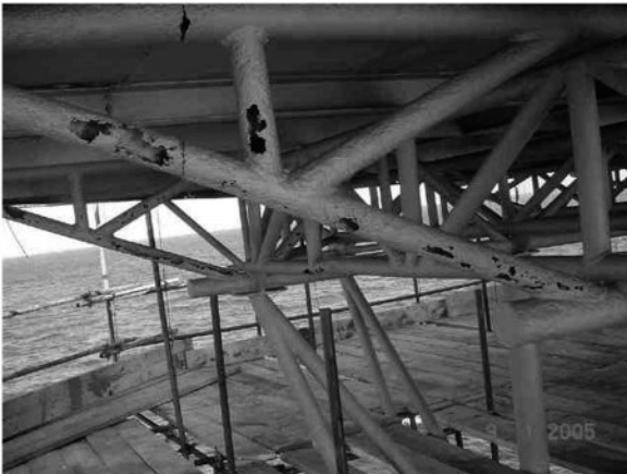
FIGURE 8.26 Truss corrosion.
