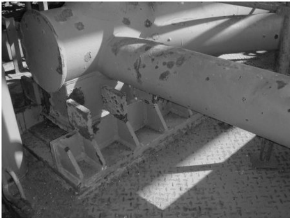
FIGURE 8.24 Corrosion of a bridge support.
