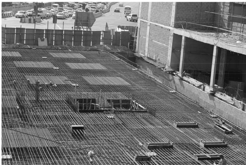
FIGURE 1.6 Dubai building during construction.
