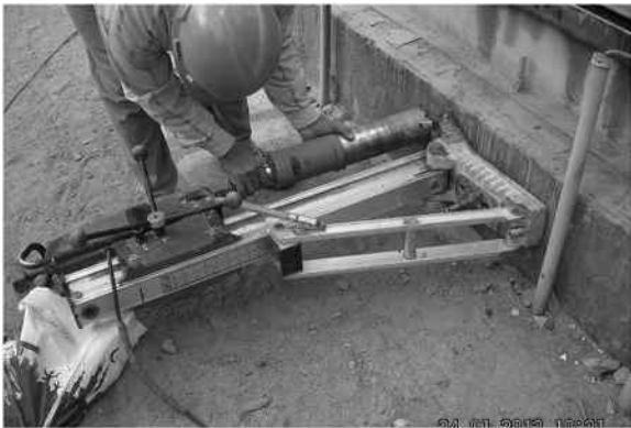
FIGURE 9.1 How to take a core.
