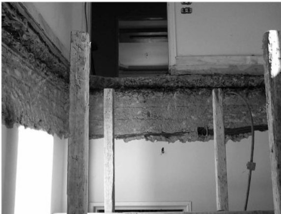
FIGURE 10.16 Pouring a new slab.
