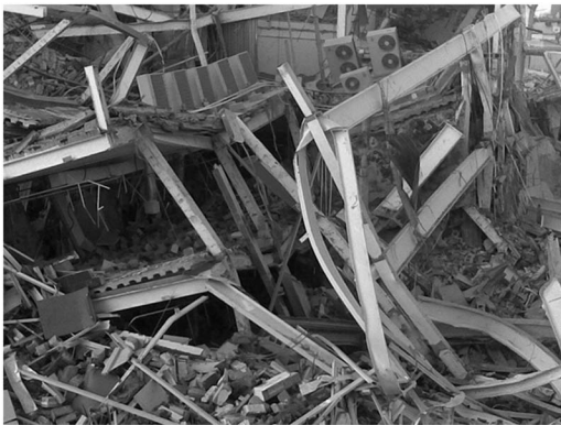
FIGURE 1.7 Dubai building collapse.
