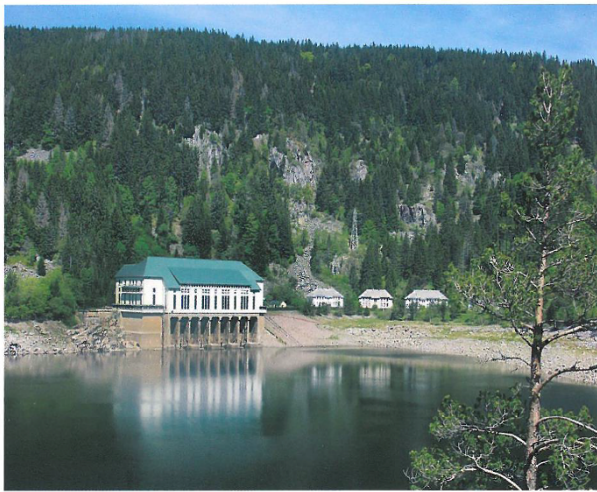
Figure 2.4. Lac Noir in the Vosges massif and the old pump-turbine station
