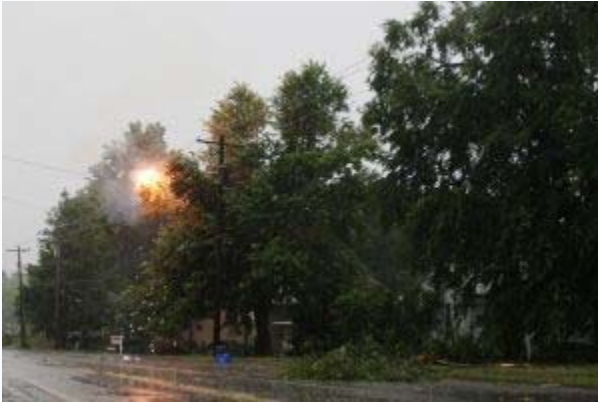
Tree limbs cause a short circuit during a storm
