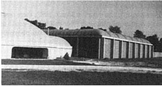
Figure 2. Overall picture of facility including manufacturing area.
