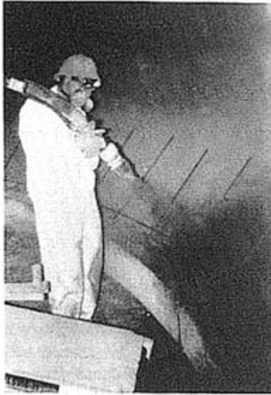
Figure 3. Shotcreting base of dome at footer location.
