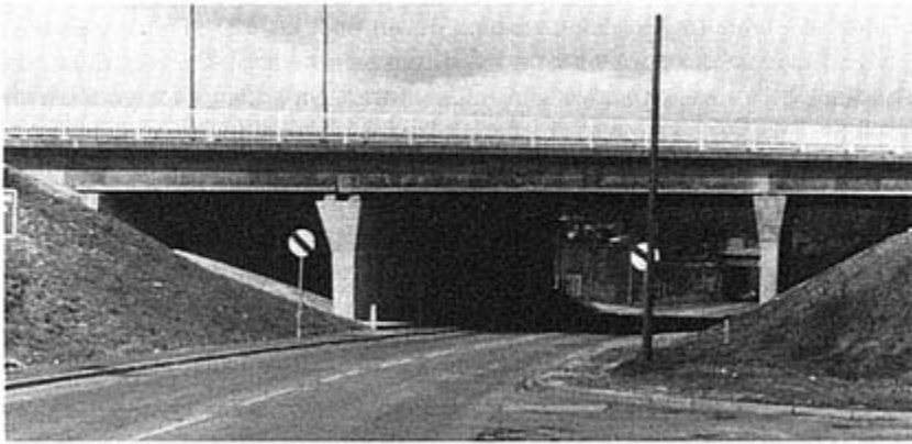
Fig. 2. View of Lawns Lane Bridge
