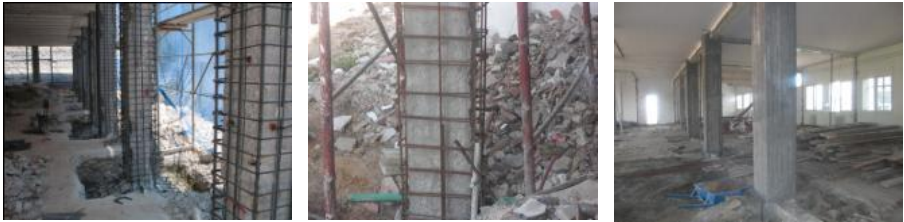
Figure 7. Increasing the section of column by reinforced concrete jacketing.
