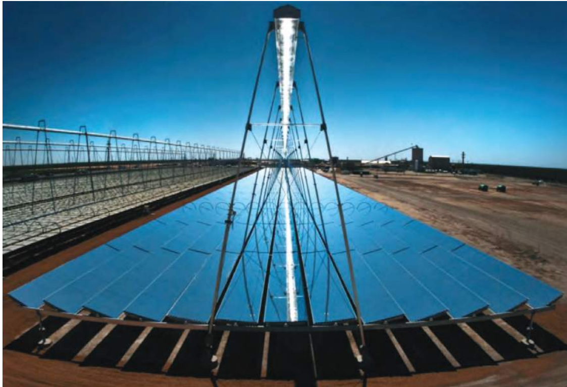
Figure 3.6 Linear Fresnel Collector Design 9
