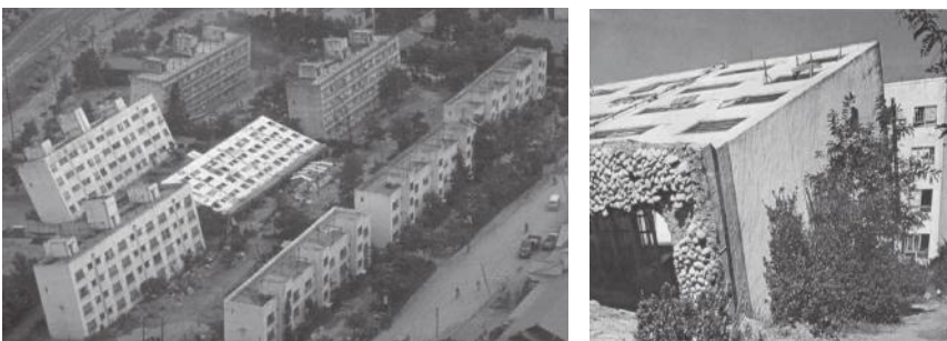
FIGURE 1.5 Building tilt and settlement due to liquefaction during the 1964 Niigata earthquake.
